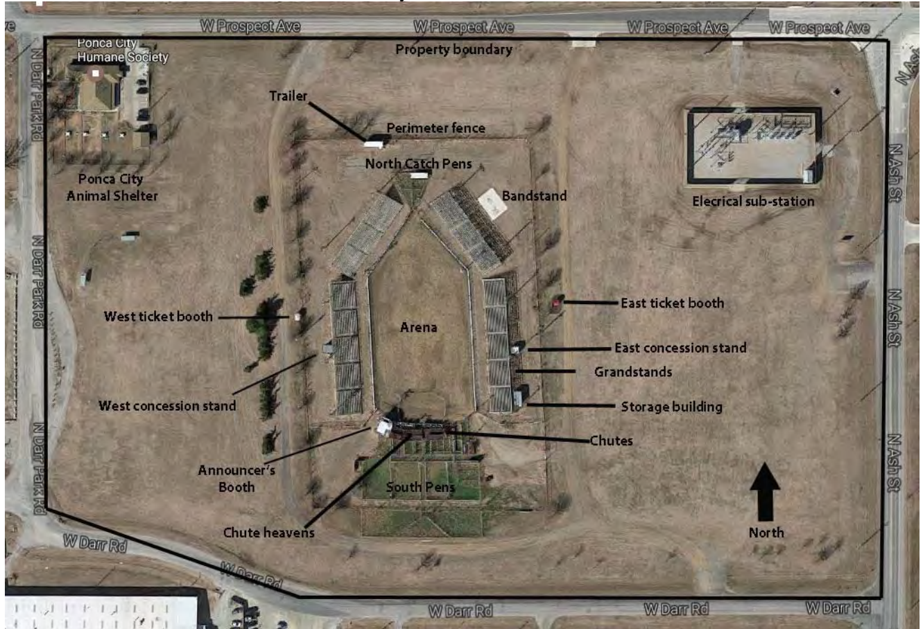
Figure 3: Aerial photo. Source: Google Maps, 2017 101 Rodeo Arena, 2600 N. Ash Street Ponca City, OK 74601. 36.737544, -97.09235. WGS84 Datum.
