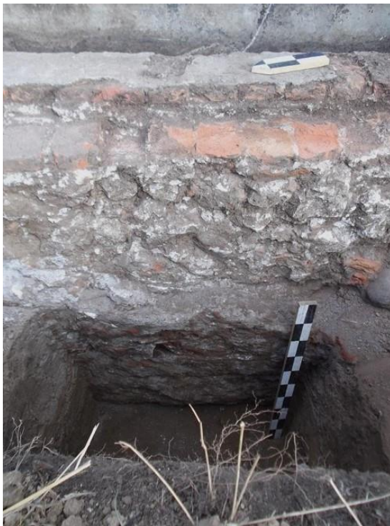
Left, detail of outer side of the west wall and foundation of the supply channel, in an area where the open channel is buried. On the right, detail of outer side of the west wall and foundation, in an open section where the channel is above the surface.
