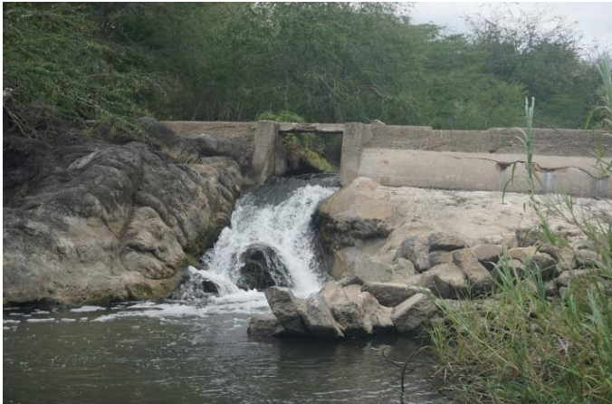
On the left, view the central area of the dam with the added opening for the sluice, seen upstream from the east bank. On the right; detail of the two construction phases of the structure: lower part built from brick masonry in the 19th century, and 20th century upper part of reinforced concrete.
