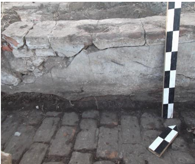
Detail of the makeup and construction method for the Hacienda El Destino Channel. Left, the inside of the west wall of the channel, covered with concrete, with some exposed bricks. Note that the floor has lost its concrete plastering. On the right, exterior view of the same wall segment.
