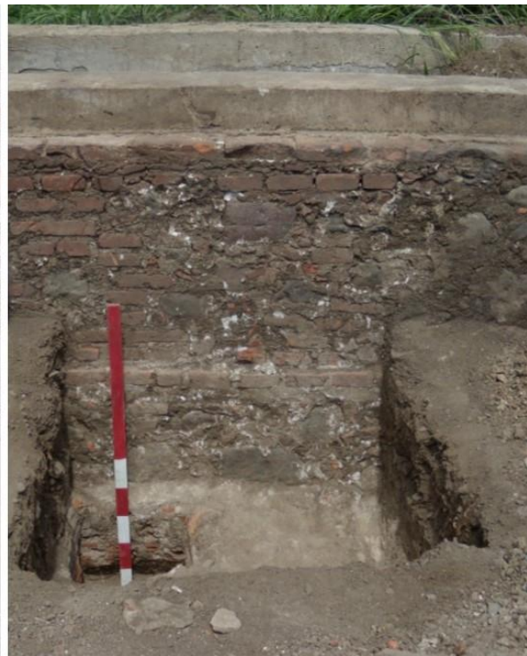
Left, detail of outer side of the west wall and foundation of the supply channel, in an area where the open channel is buried. On the right, detail of outer side of the west wall and foundation, in an open section where the channel is above the surface.
