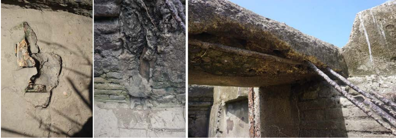
Left and center; remnants of the wood frame of the inner sluice gate of the low waters module. Left; detail of the inner gate of the module, with part of the metal sluice and metal bars that created a garbage trap.
