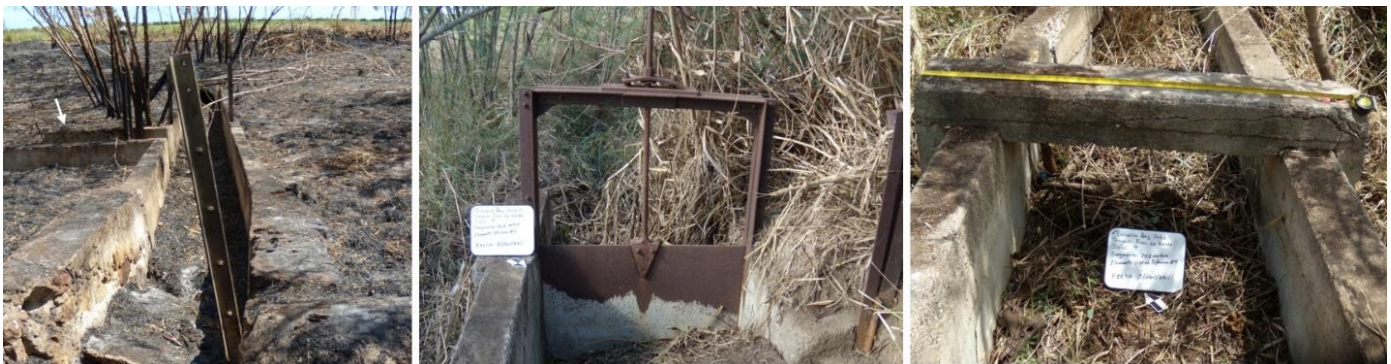
On the left, view of the Hacienda Destino channel, facing west. White arrow shows a channel that was added when it became part of the Irrigation District. In the center, detail of added sluice gate. Right; reinforcement beam added to the Hacienda Florida Channel.
