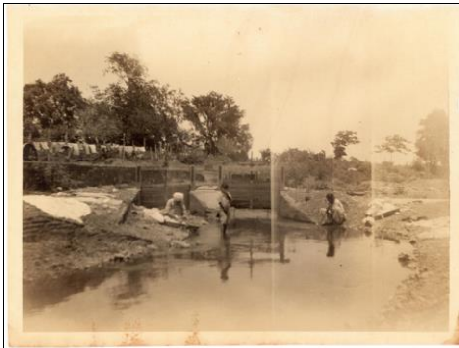
Photo of the main intake for the Florida, Santa Isabel and Destino Haciendas or Tres Haciendas at the junction of the main canal and the Coamo river, 1913, AAA (from Meléndez Maíz 2011).
