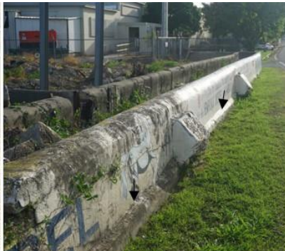
Left; Channel of the Hacienda Florida, raised on arches. Center; Channel of the Hacienda Florida, elevated on a base (note black arrows). Right; Channel of the Hacienda Florida, raised using a staggered base.
