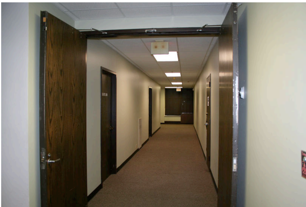
Image 6. Interior – Representative View of 2 nd – 4 th Floor Corridor
