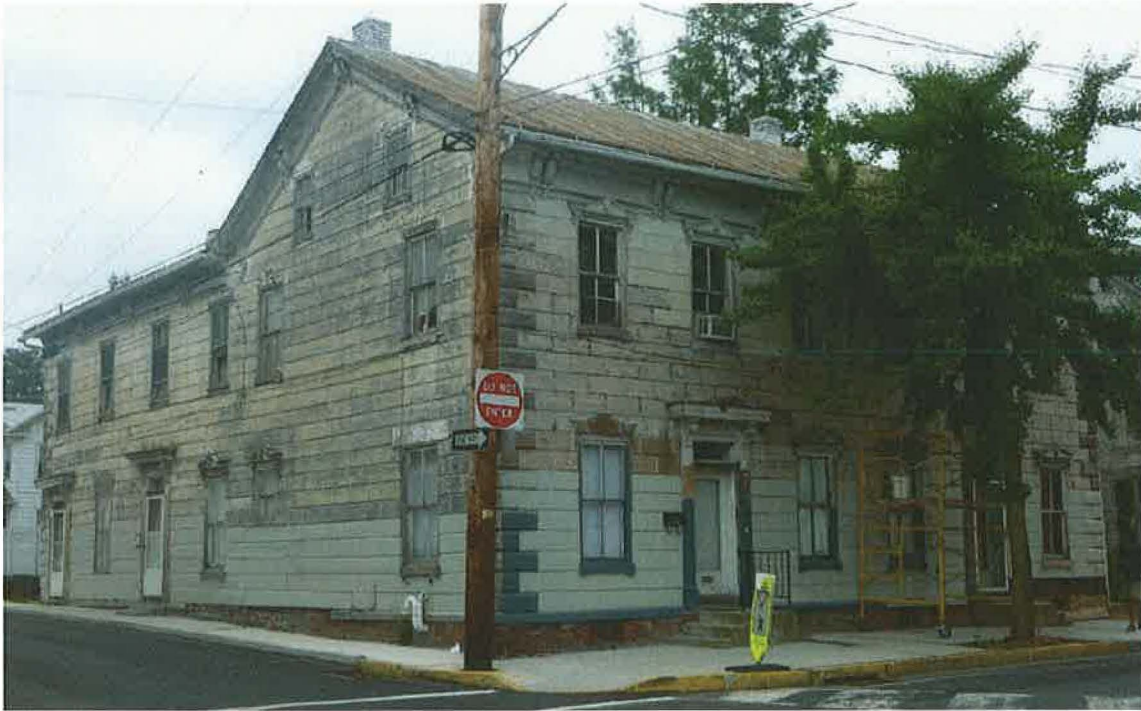
Figure 11: Photos of a house at 203 Main Street, Mechanicsburg, Cumberland County, south-central Pennsylvania. This house features wood siding imitating cut stone, with quoins, similar to the Tioga County examples in Figure 8.
