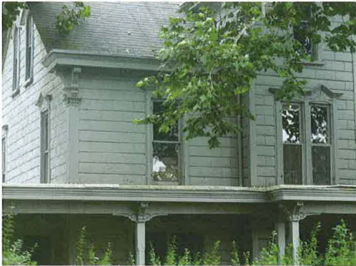
Figure 10: Photos of three houses (c.1885) in an area known as Craighead Station, Cumberland County, south-central Pennsylvania. All three feature at least a front façade of wood siding imitating cut stone.
