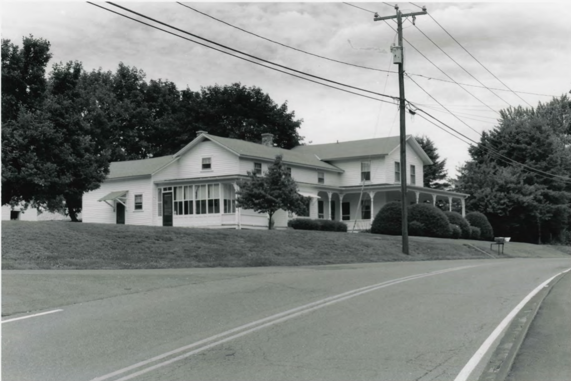
Field-Hubbard-Botkin House Mill-Prospect Street Historic District Hampshire, MA Photograph #2
