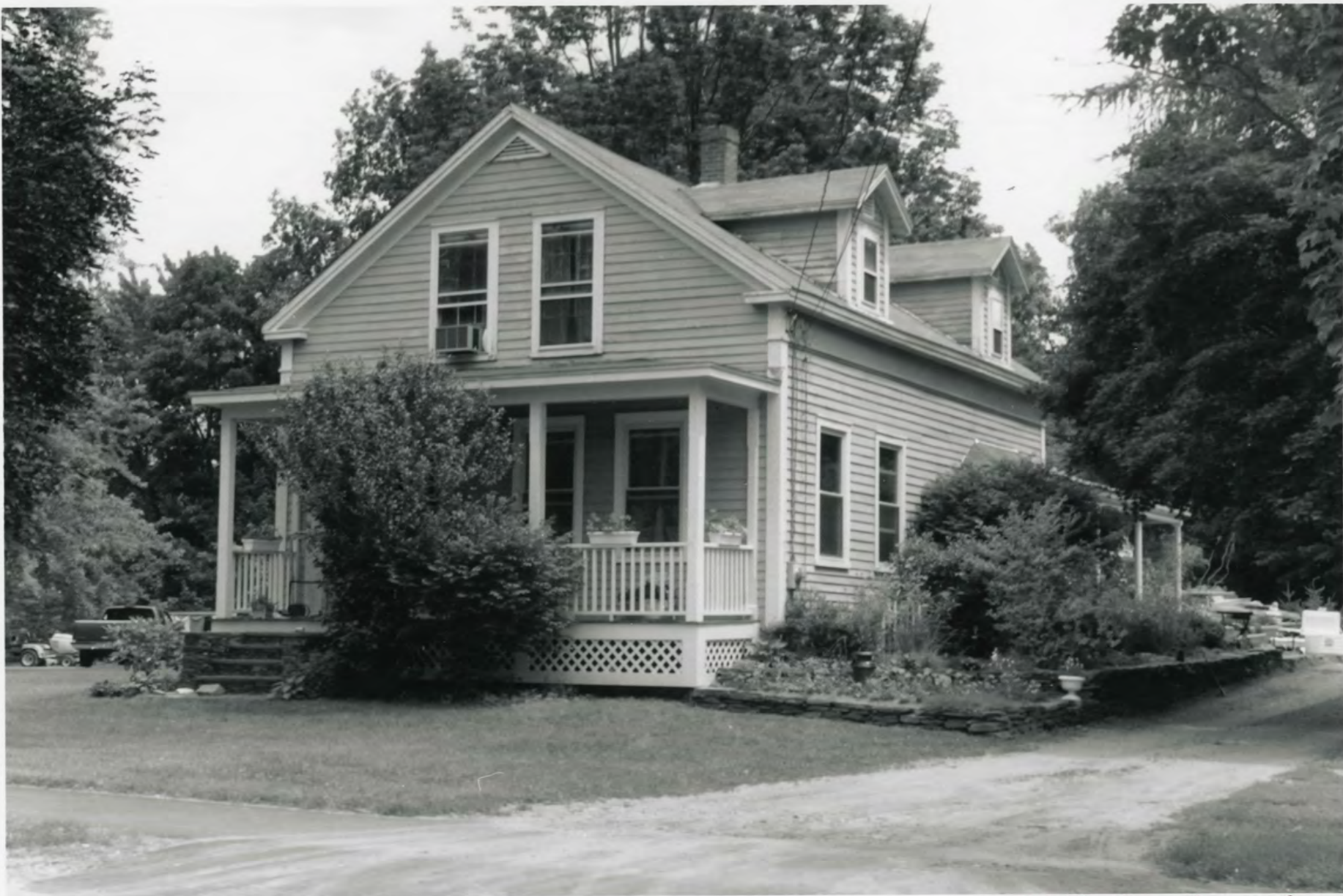
Fitch Brothers General Store Mill - Prospect Street H.D. Hampshire, MA Photograph # 11
