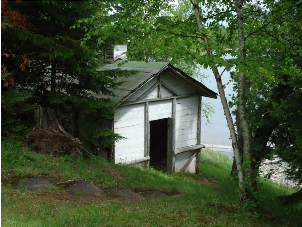
19 of 27. Ice house, West Bay Club, west facade.
