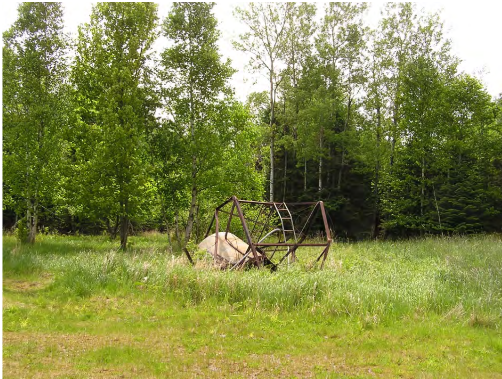
22 of 27. Collapsed water tank and tower at West Bay Club.
