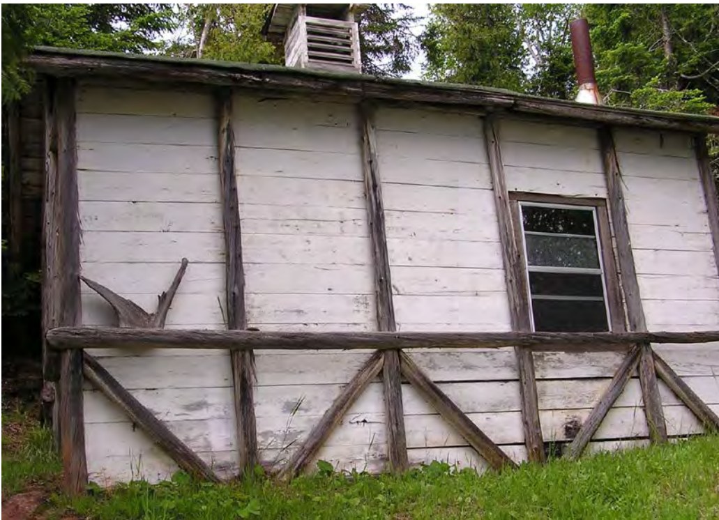
20 of 27. South facade, Ice House, West Bay Club.
