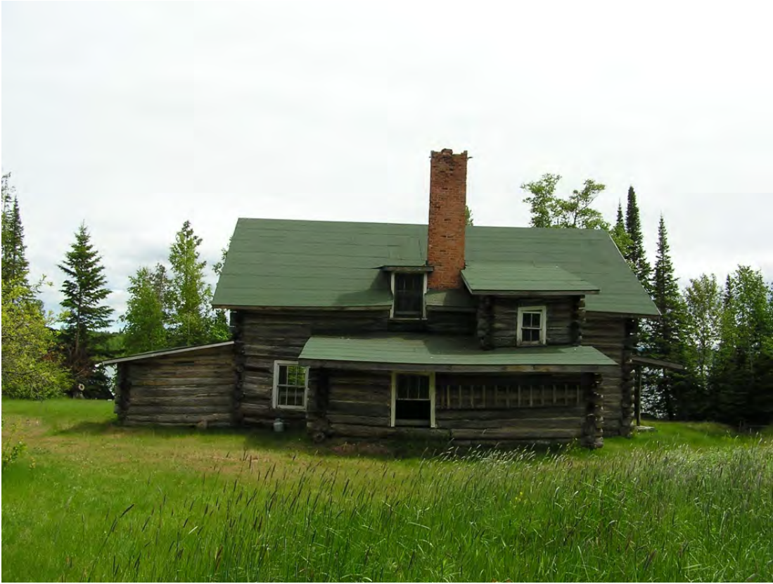
9 of 27. North side of West Bay Club lodge.
