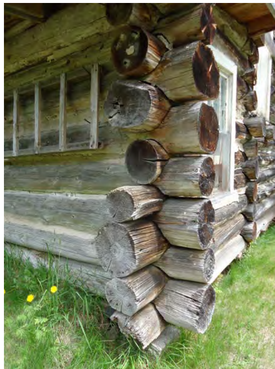
10 of 27. Detail of saddle-notched corners of West Bay Club lodge.
