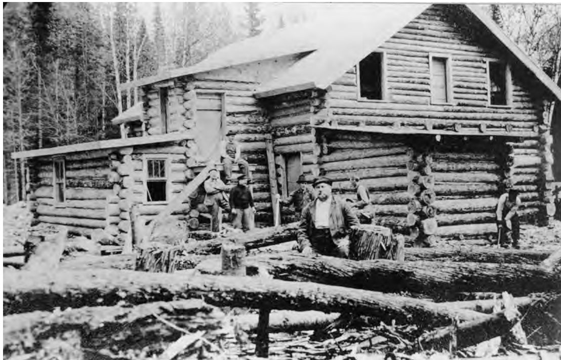
14. The lodge under construction. Apostle Islands National Lakeshore.
