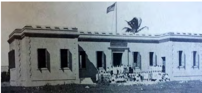
James Garfield Graded School, Guánica
