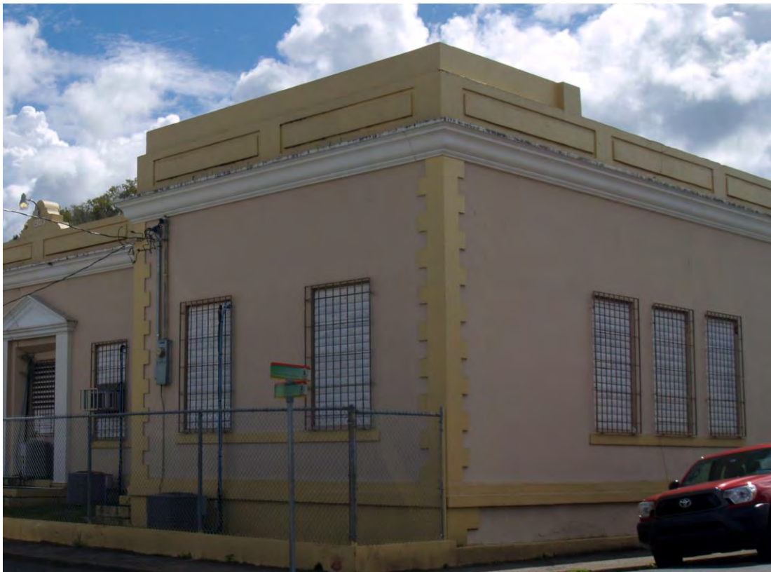
Figure 3. Partial view of the western façade, with the three closely grouped windows, the faux-rusticated quoins in the foreground, and the 1919 concrete structure added over the original parapet (Source: Juan Llanes Santos, 2014).
