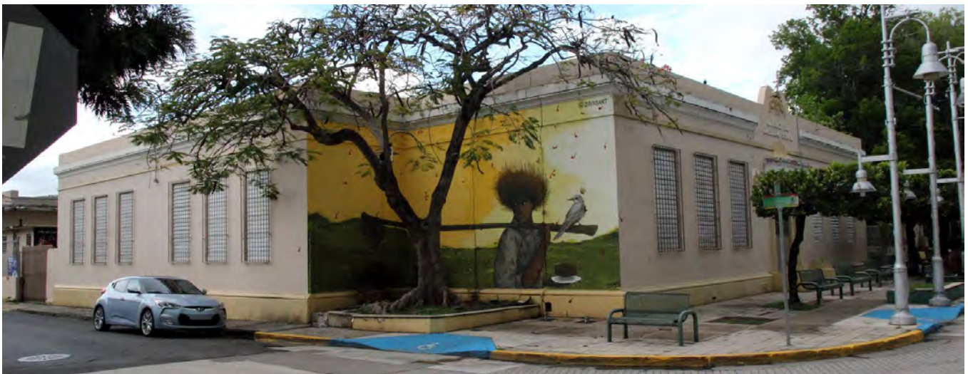
Figure 6. View of the western (left) and southern facades. Mural at the foreground was done by artist David Zayas, to commemorate the 60 th anniversary of the Instituto de Cultura Puertorriqueña (Source: Juan Llanes Santos, 2017).
