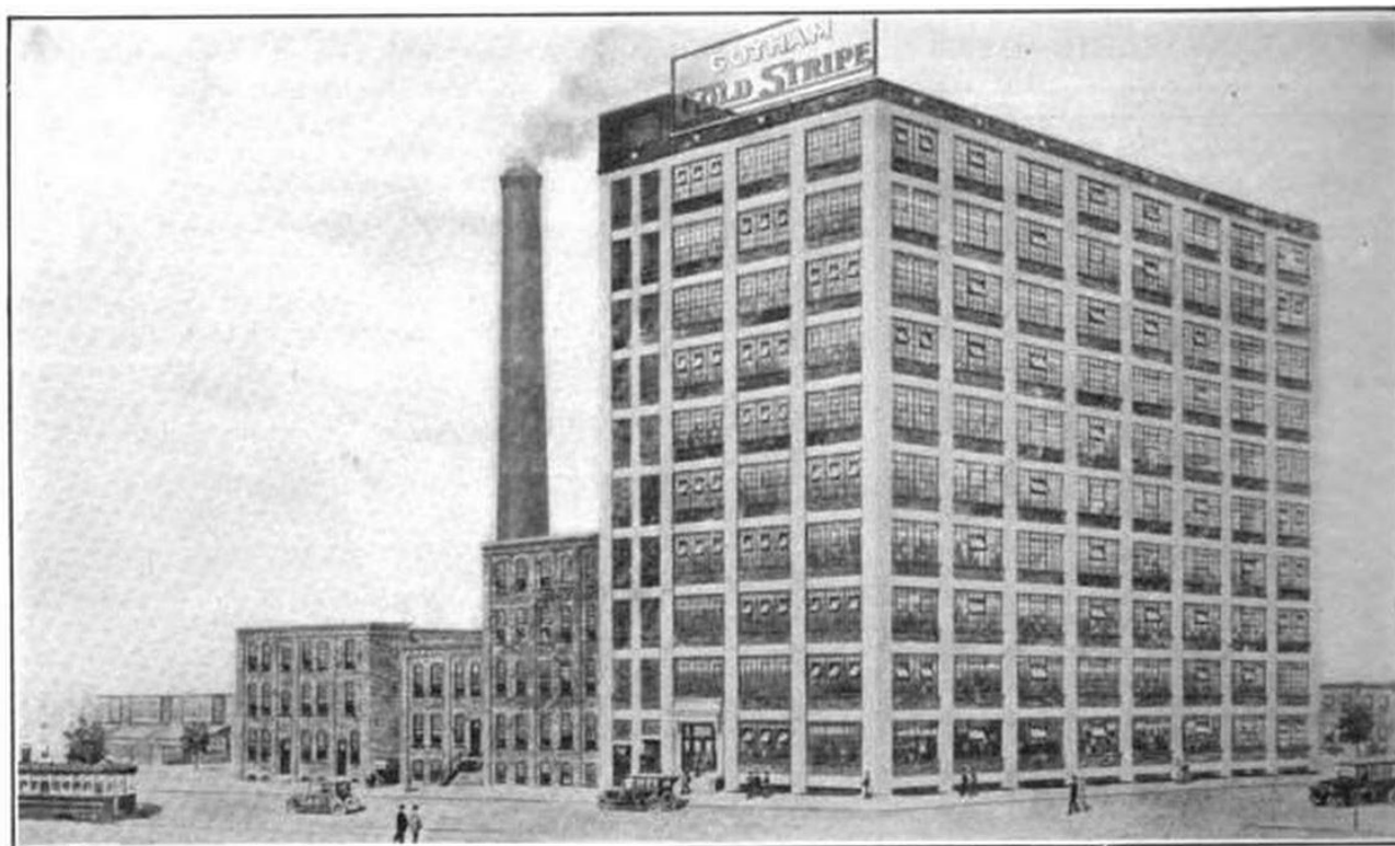
NEW PLANT OF GOTHAM SILK HOSIERY CO. NOW UNDER CONSTRUCTION IN PHILADELPHIA. THE OLD PLANT IS SEEN AT THE LEFT.
