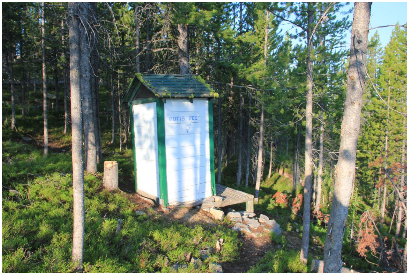
ID_Idaho County_Butts Creek Point Fire Lookout_0013
