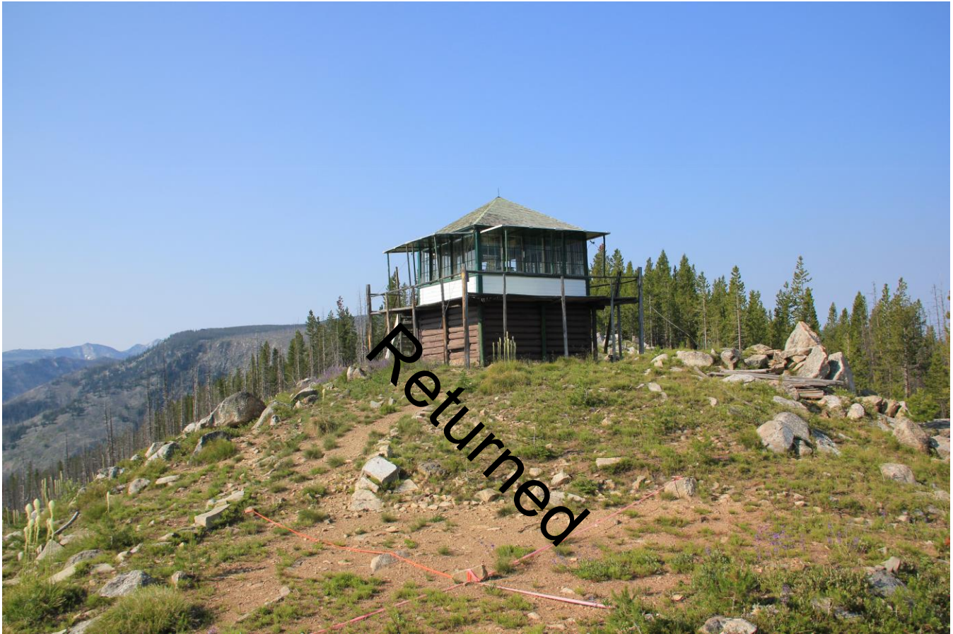
ID_Idaho County_Butts Creek Point Fire Lookout_0015
