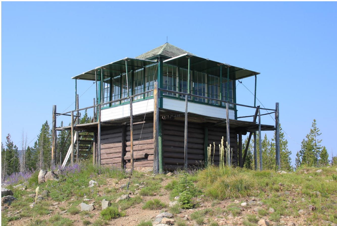
ID_Idaho County_Butts Creek Point Fire Lookout_0005
