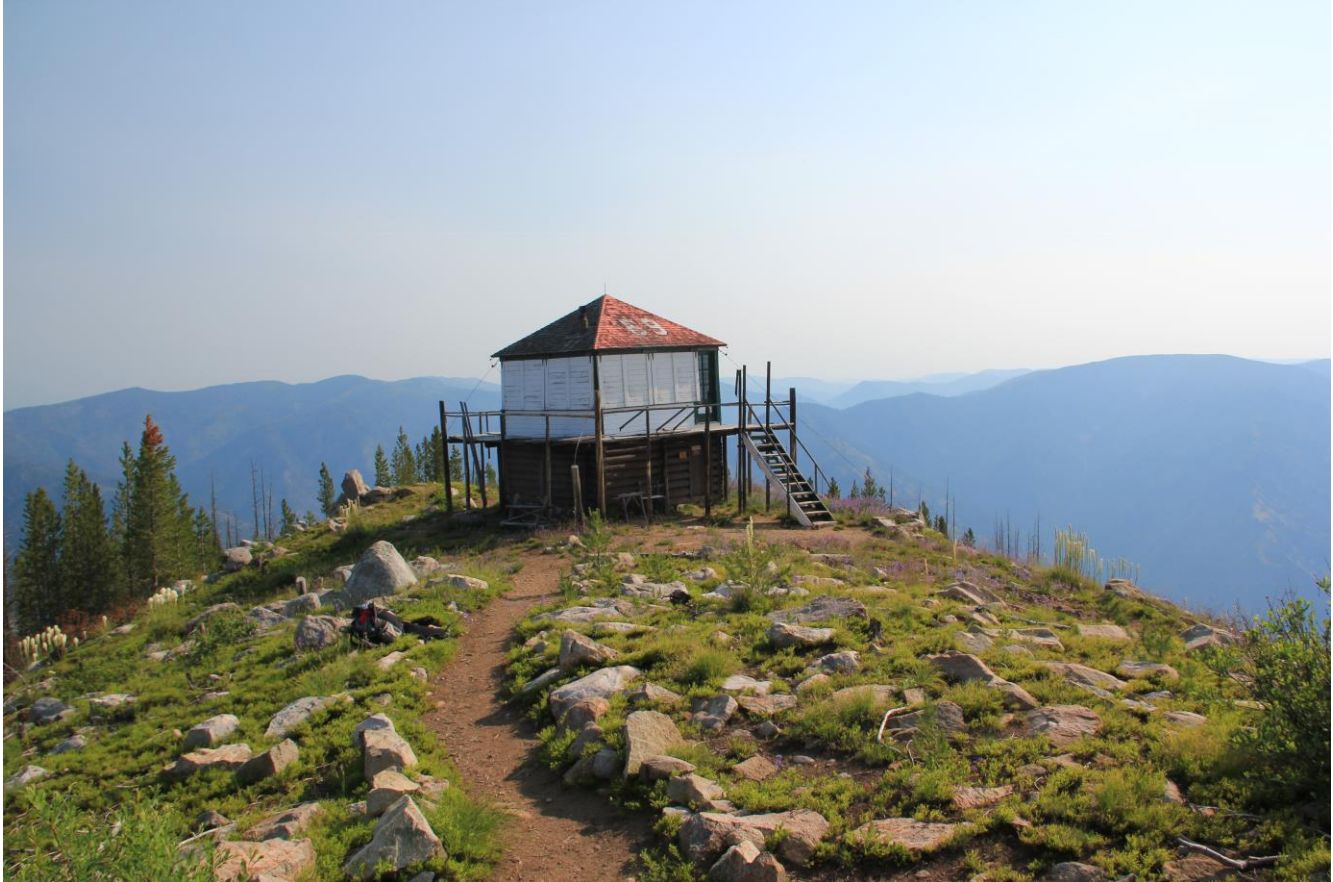
ID_Idaho County_Butts Creek Point Fire Lookout_0002
