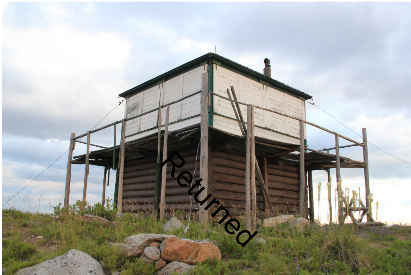
ID_Idaho County_Butts Creek Point Fire Lookout_0004
