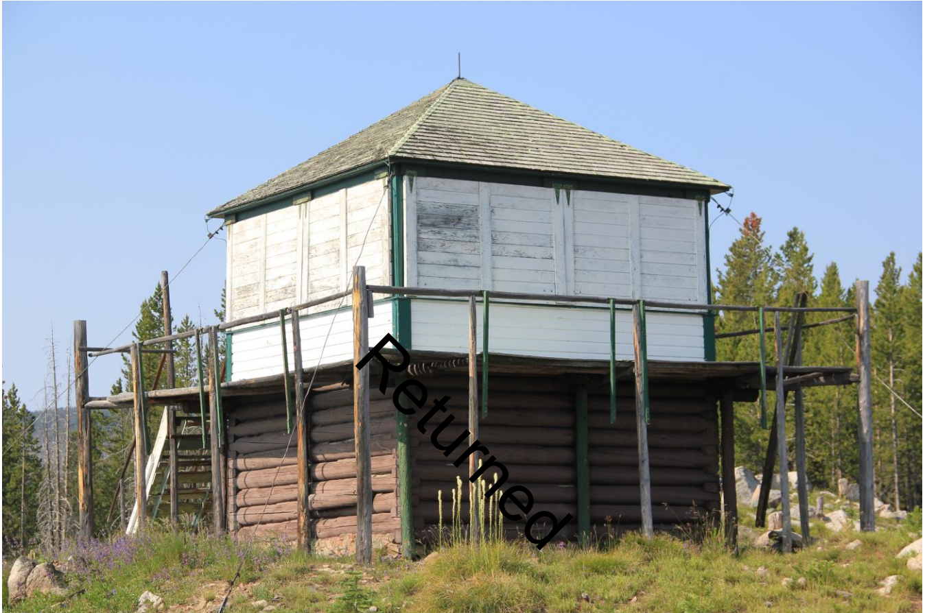
ID_Idaho County_Butts Creek Point Fire Lookout_0007
