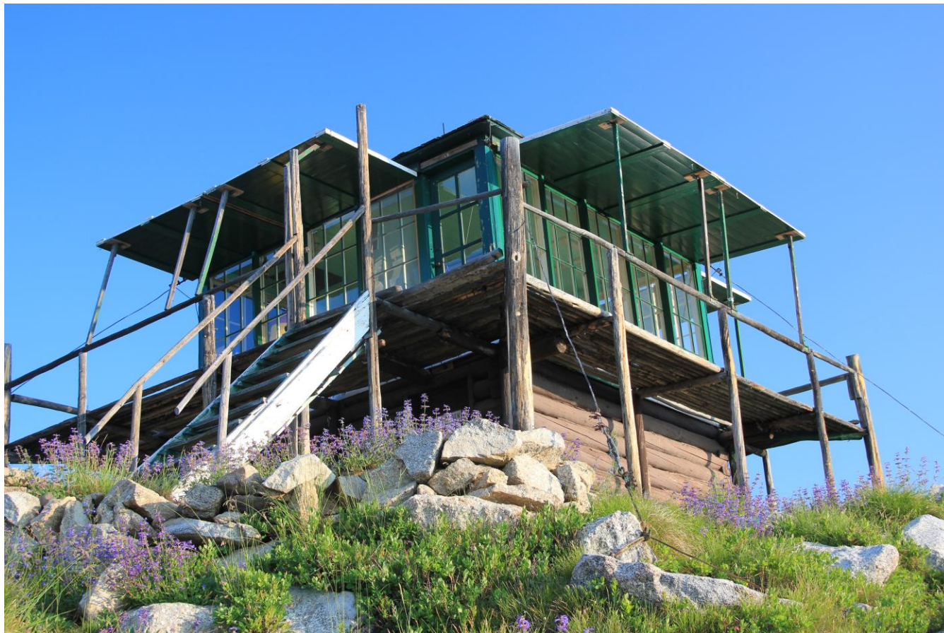
ID_Idaho County_Butts Creek Point Fire Lookout_0006
