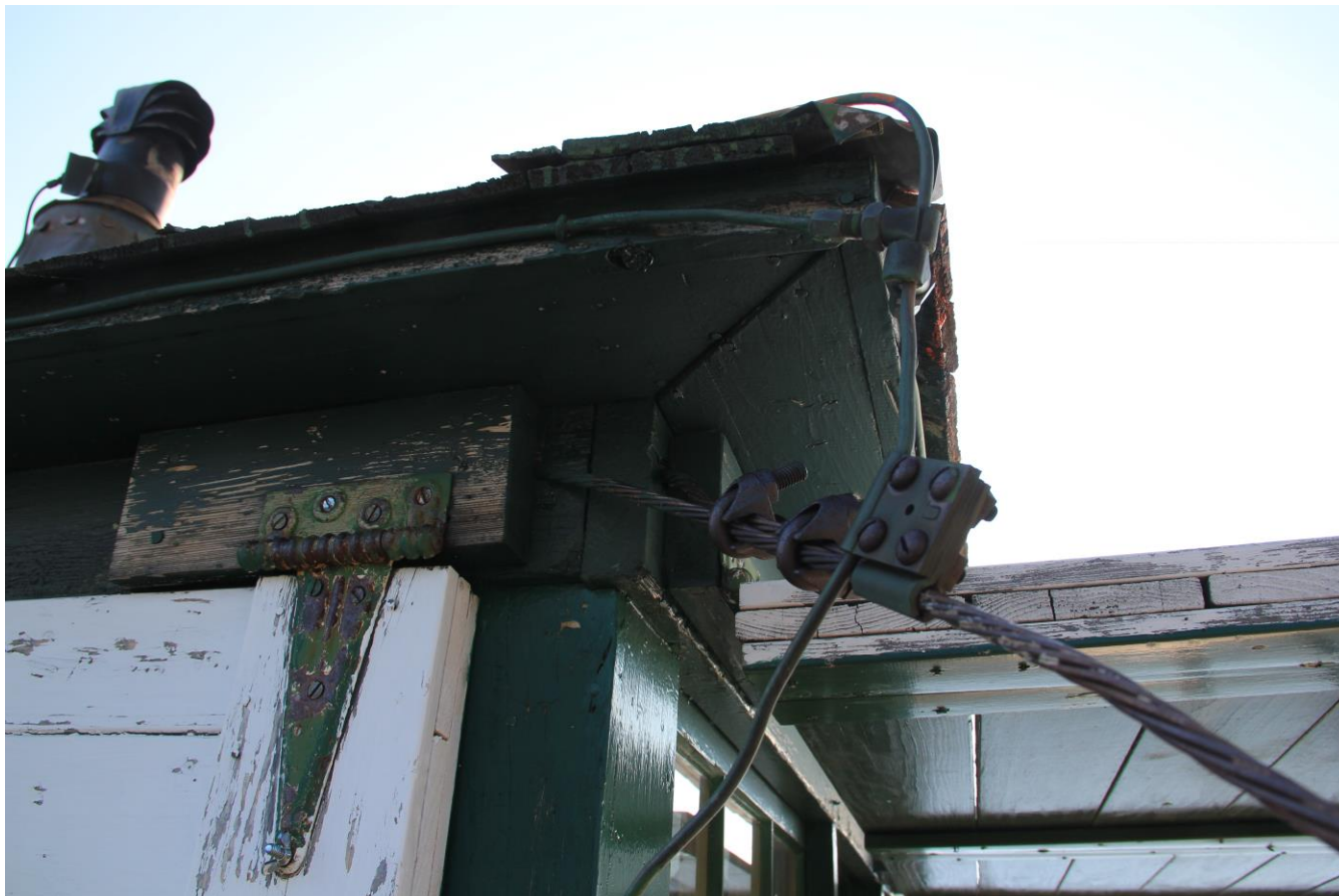
ID_Idaho County_Butts Creek Point Fire Lookout_0008
