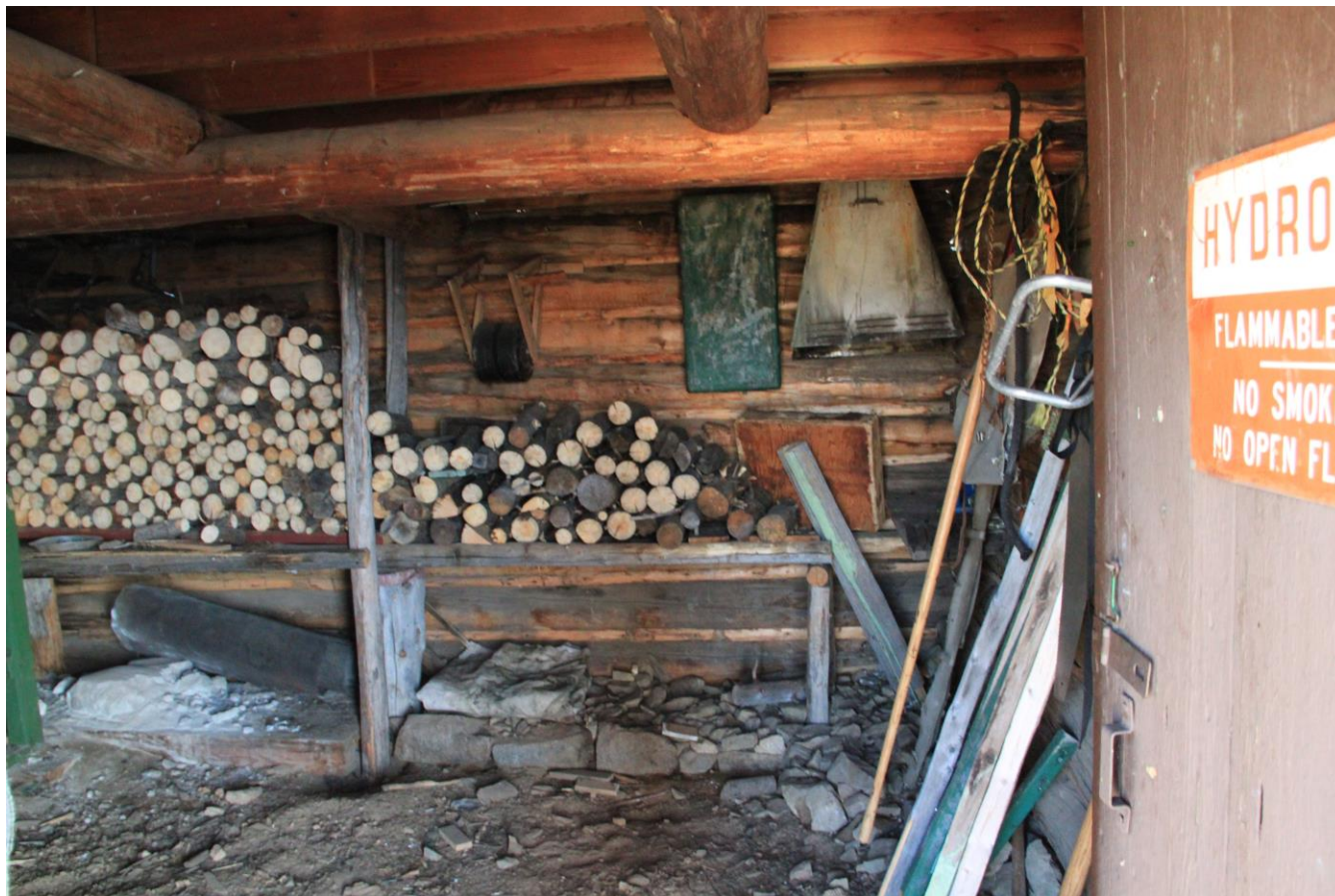
ID_Idaho County_Butts Creek Point Fire Lookout_0012
