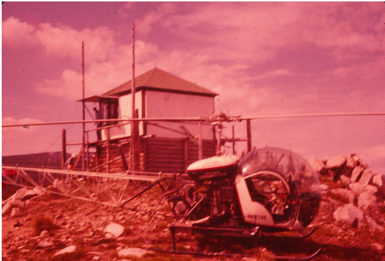
ID_Idaho County_Butts Creek Point Fire Lookout_0016
