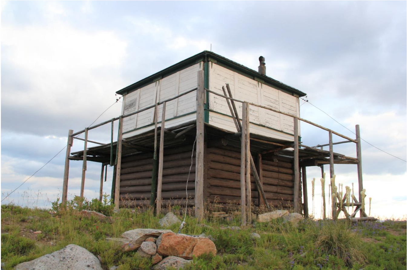
ID_Idaho County_Butts Creek Point Fire Lookout_0004
