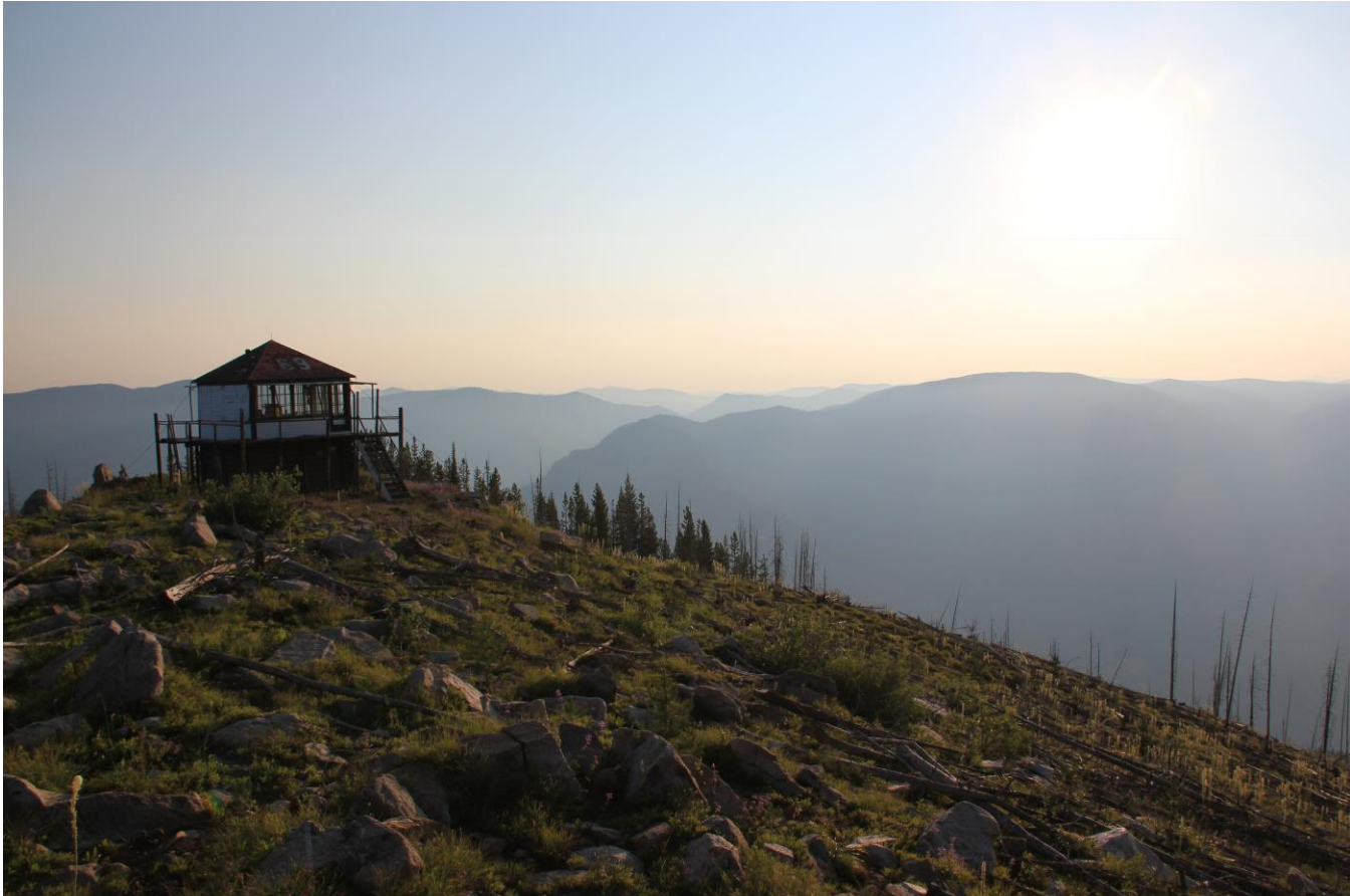
ID_Idaho County_Butts Creek Point Fire Lookout_0001
