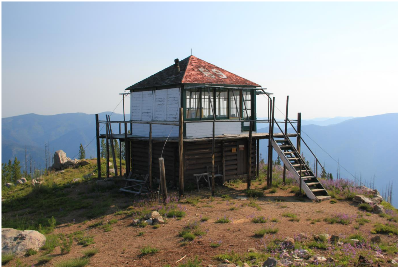
ID_Idaho County_Butts Creek Point Fire Lookout_0003
