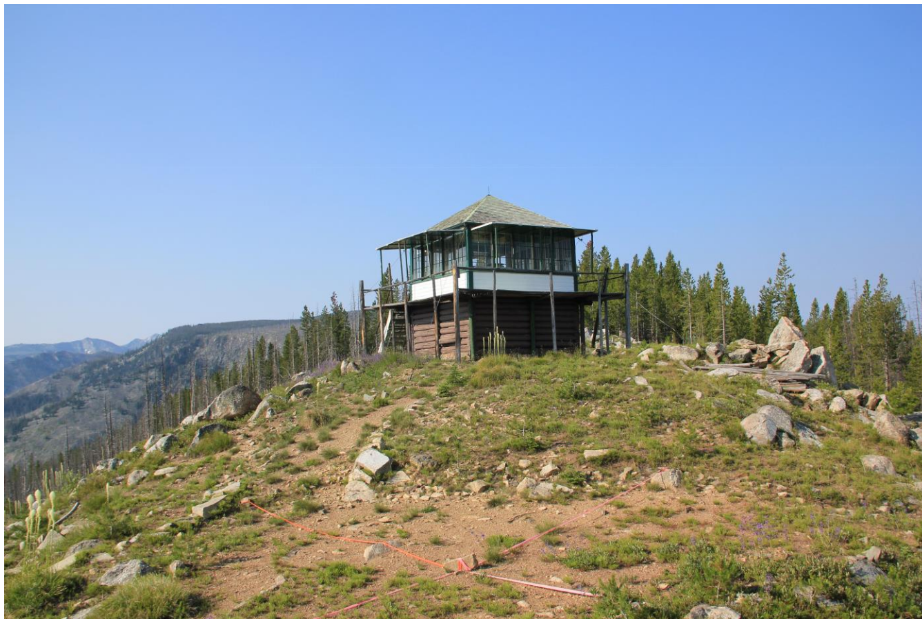
ID_Idaho County_Butts Creek Point Fire Lookout_0015
