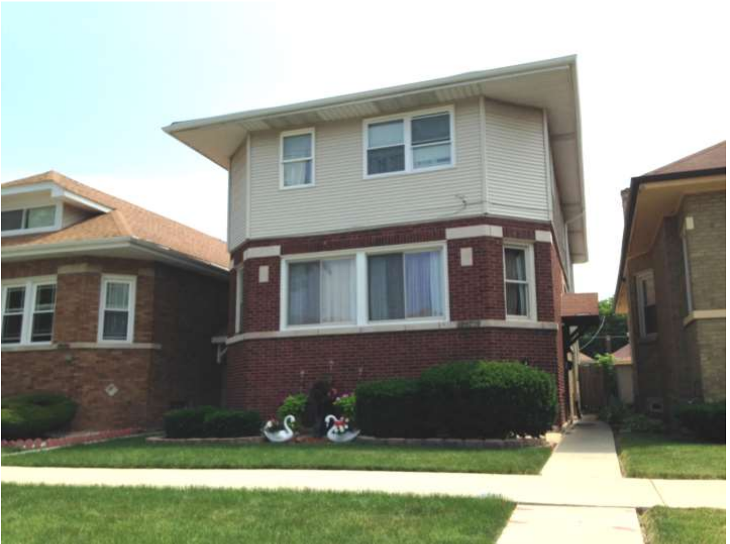
IMAGE 2: An example of a bungalow that is noncontributing due to a second-story addition at 9425 S. Loomis.
