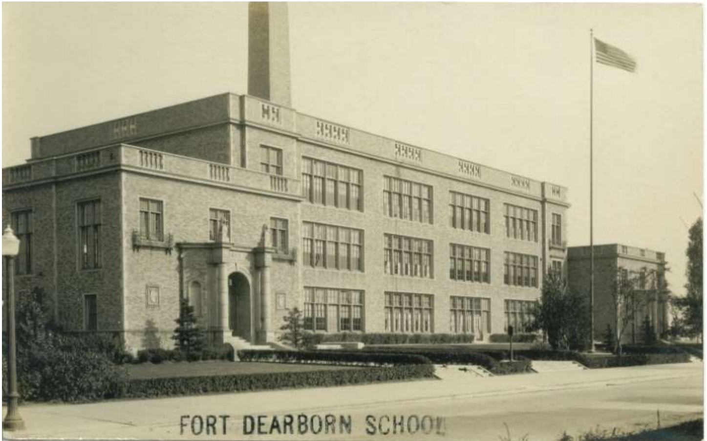
IMAGE 12: Historical photo of Fort Dearborn School (exact date unknown), primary façade, facing northeast.
