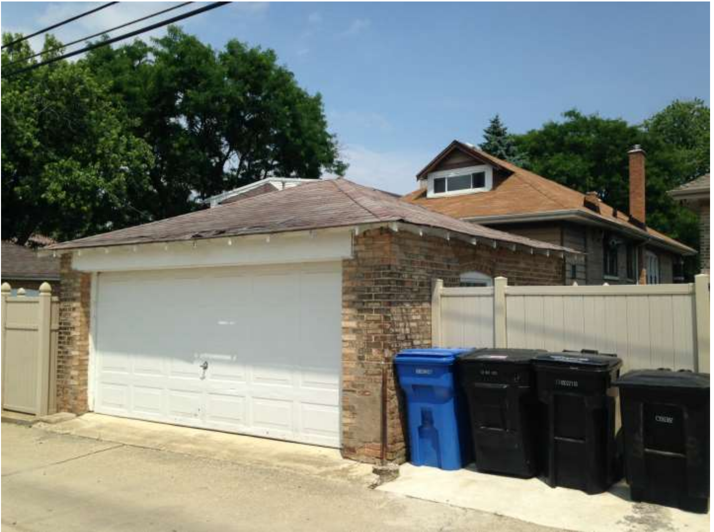
IMAGE 3: An example of a contributing garage at 9304 S. Racine.
