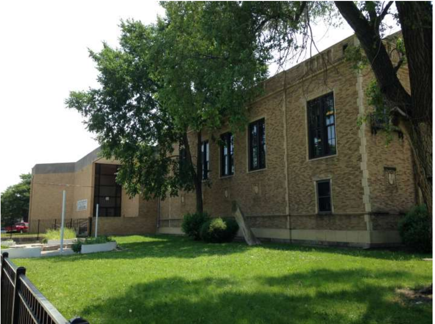
IMAGE 14: Beginning of school addition at recessed southwest portion of south façade.
