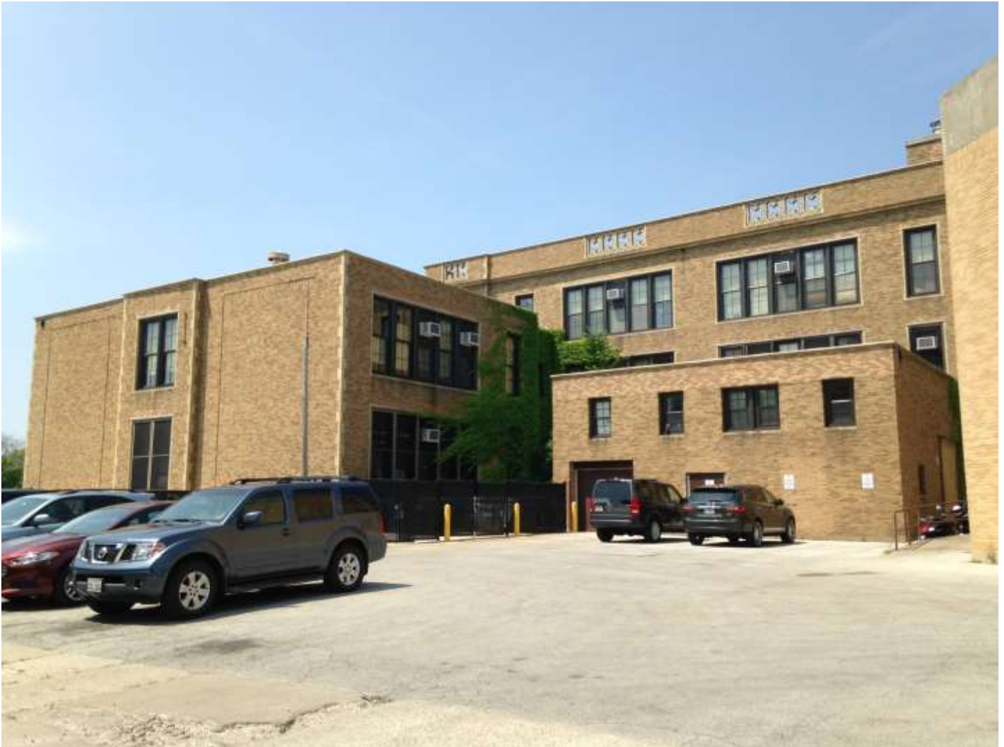
IMAGE 16: Rear of school (west façade) showing where transition from addition to original building at parking lot.
