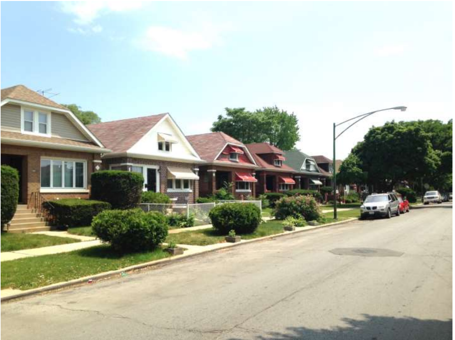
IMAGE 6: Frame gabled roofs and clipped peaks along the 8900 block of S. Racine.
