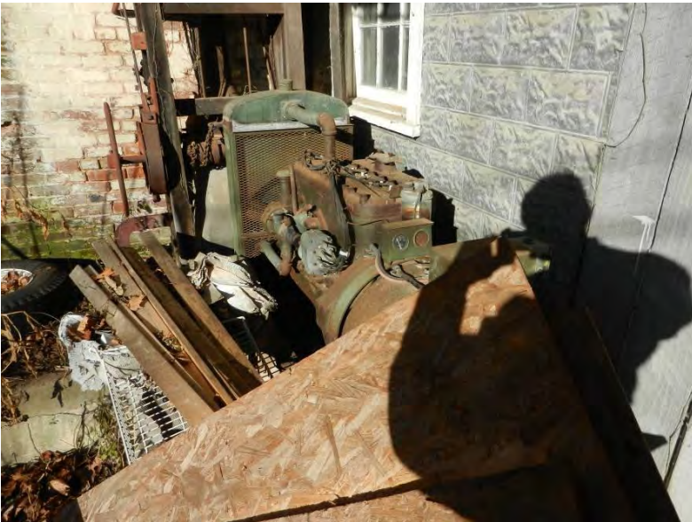
Photo 28: WV_JeffersonCounty_Feagans'Mill_028 Feagans' Mill, Entry, Looking North, Diesel Generator (United States Systems)
