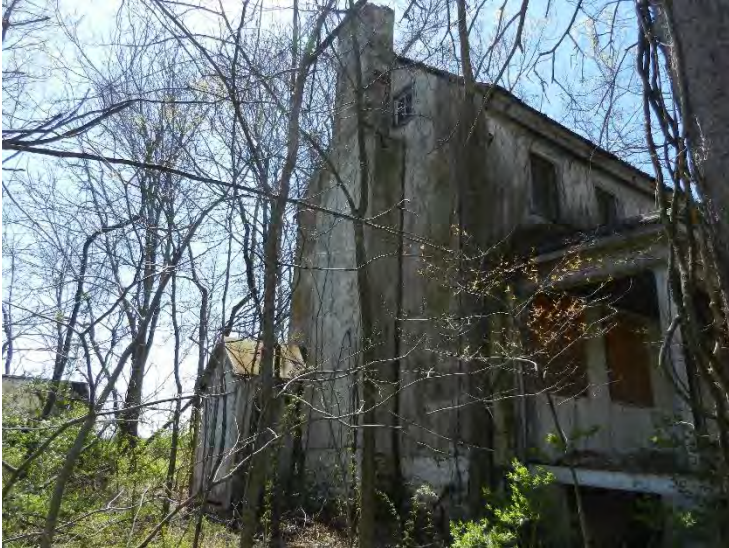
Photo 37: WV_JeffersonCounty_Feagans'Mill_037 Feagans' Miller House, Facing South-Southwest
