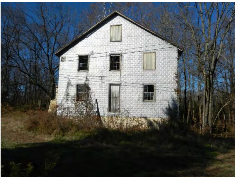
Photo 2: WV_JeffersonCounty_Feagans'Mill_002 Feagans' Mill, South Elevation (façade), Facing North
