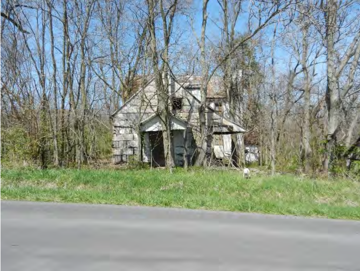
Photo 35: WV_JeffersonCounty_035 Feagans' Miller House, Facing North
