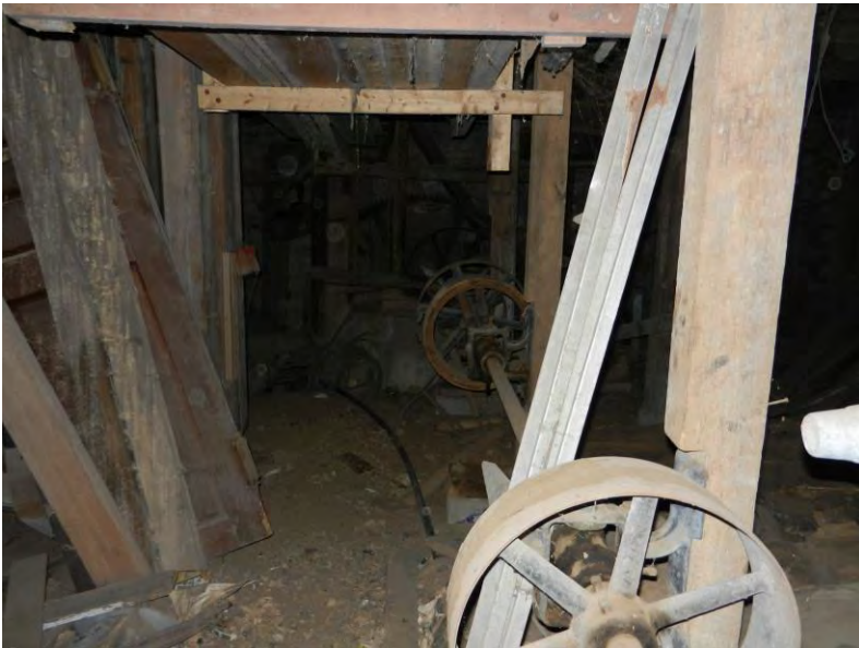
Photo 40: WV_JeffersonCounty_Feagans' Mill_040 Basement, Facing North
