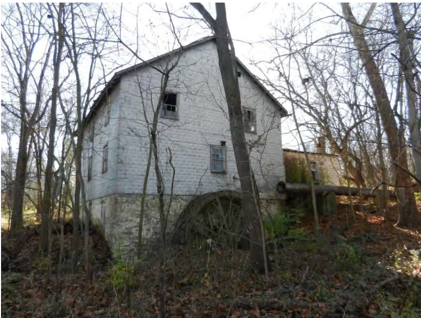
Photo 6: WV_JeffersonCounty_Feagans'Mill_006 Feagans' Mill North Elevation with Fitz Wheel and Partial Flume (variant)
