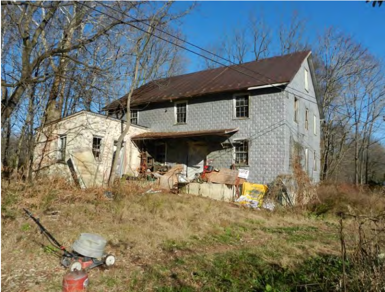
Photo 1: WV_JeffersonCounty_Feagans'Mill_001 Feagans' Mill, South and West Elevations, Facing Northeast
