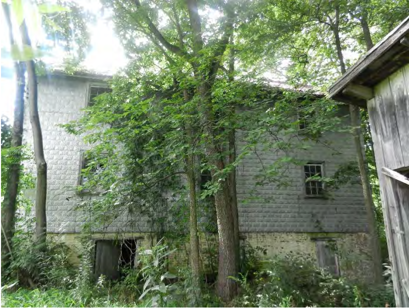
Photo3: WV_JeffersonCounty_Feagans'Mill_003 Feagans' Mill East Elevation, Facing West
