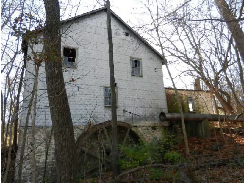
Photo 5: WV_JeffersonCounty_Feagans'Mill_005 Feagans' Mill North Elevation with Fitz Wheel and Partial Flume
