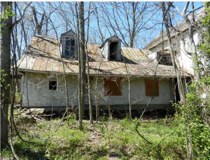
Photo 36: WV_JeffersonCounty_Feagans' Mill_036 Feagans' Miller House, Facing West
