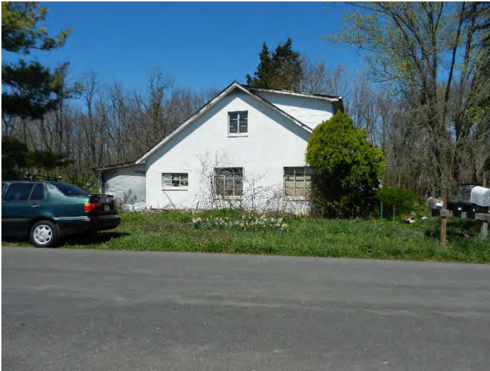
Photo 31: WV_JeffersonCounty_Feagans'Mill_031 Lutz House, Looking North
