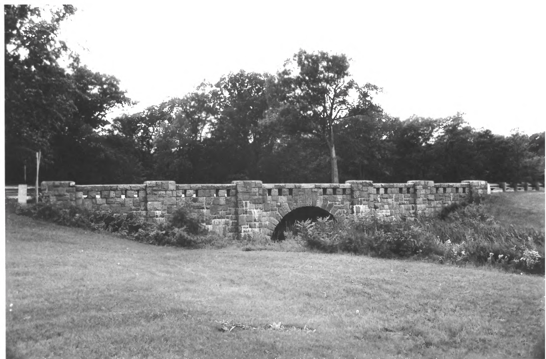
Bridge No. 5265 U.S. Highway 169, Garrison Crow Wing Co., MN D12656-20
