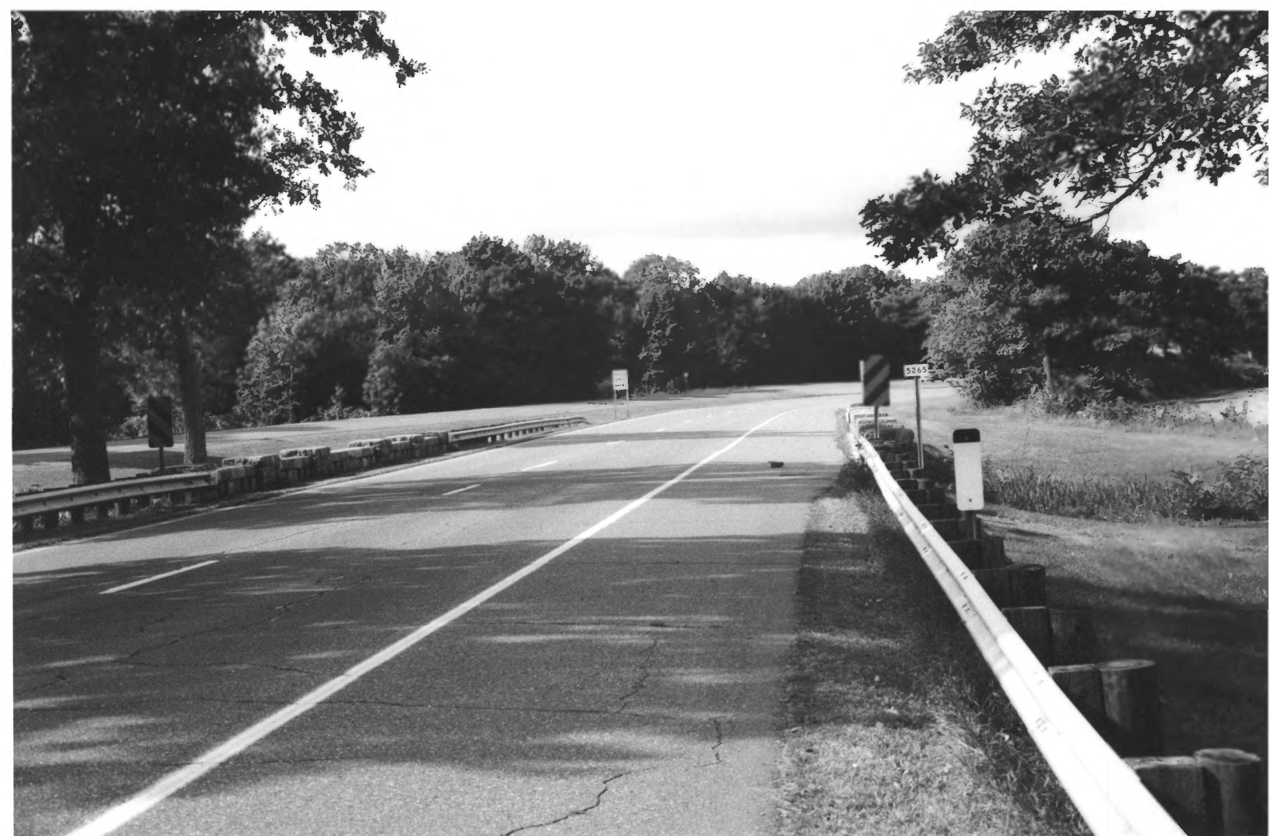
Bridge no. 5265 U.S. Highway 169, Garrison Crow Wing Co., MN 012656-2T
