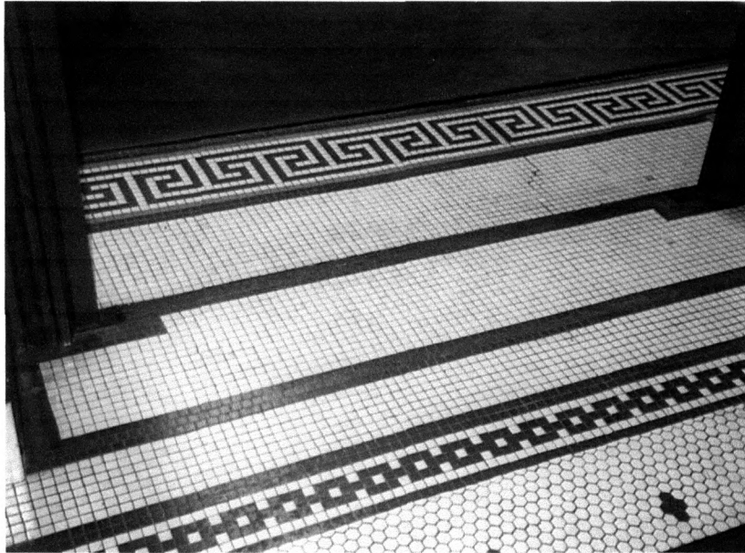
Doorway showing the different decorative tile patterns in the dining room (top) and living room (bottom)
