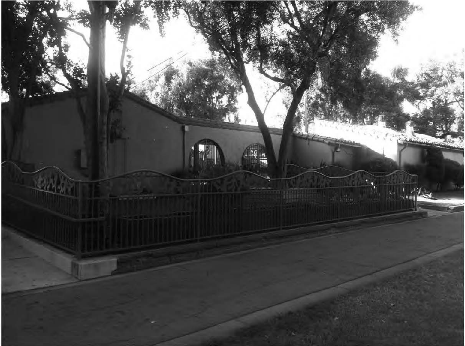
CA_Los Angeles County_Plummer Park Community Club House_004
