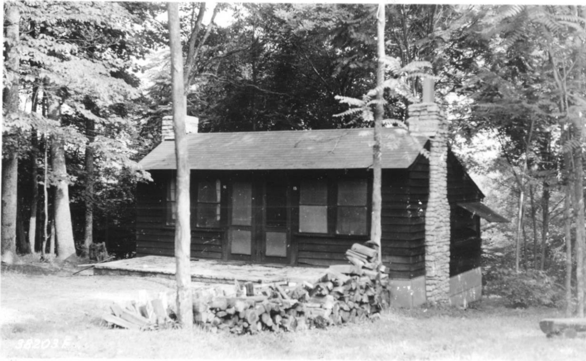
Figure 11: Photograph of Cabin 15, taken sometime prior to the transfer to the state in 1953. Note that at this time this cabin had two doors, it currently has only one door.
