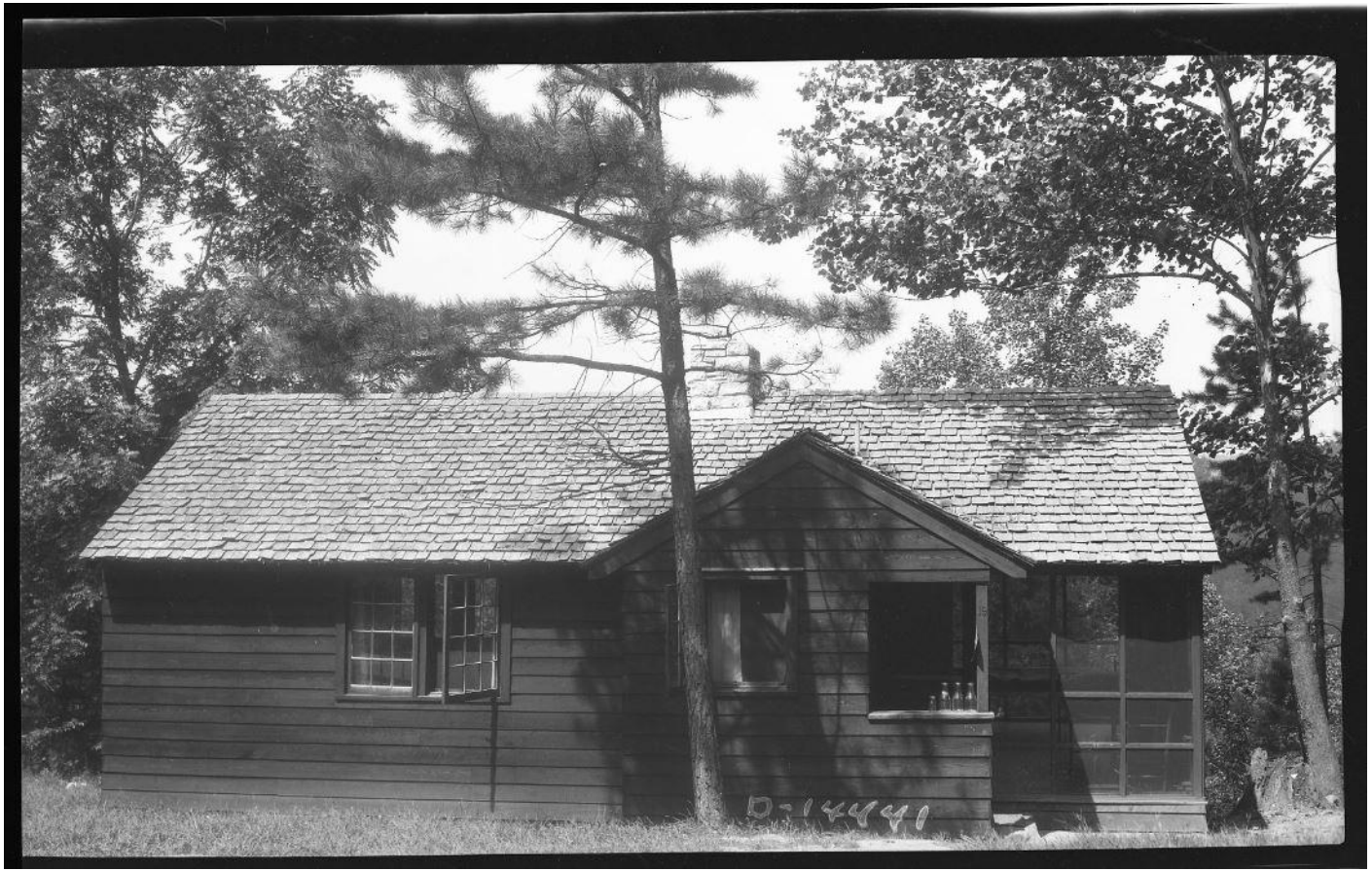
Figure 1: Photograph from September 10, 1940. “Cabin 19” Cabin 14 currently. Note the change in windows and reconfiguration of the screen porch. Photograph courtesy of National Archives at Atlanta
