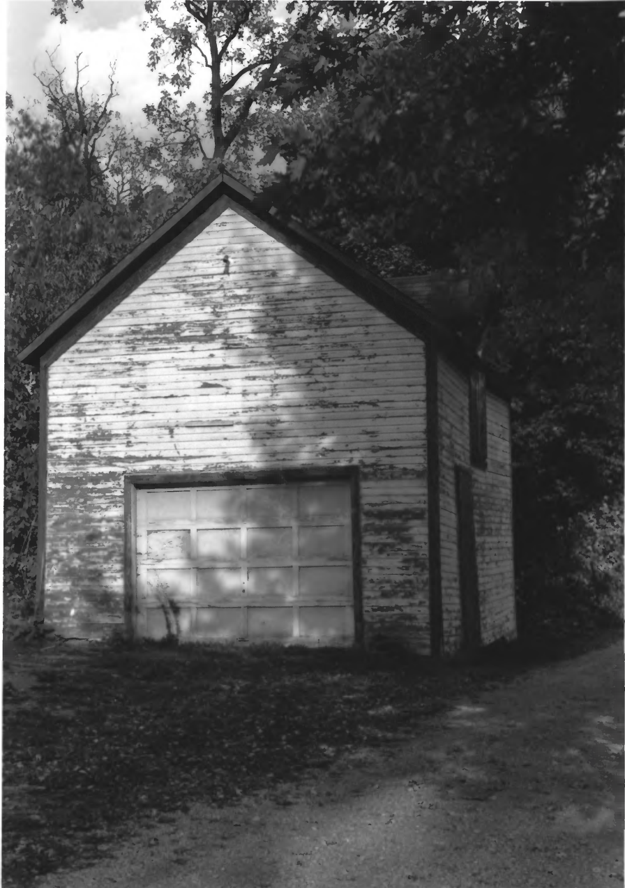
Kaukauna Lock Hst Dst, Kaukauna, Outagamie County, Photo # 5 of 7
