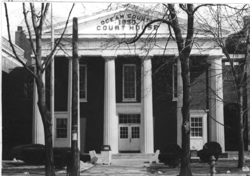
(10) Ocean County Courthouse Old Village of Toms River Multiple Resource Nomination Photographer: Charles Gaertner Date of photo: Spring 1978 Negative: Ocean County Museum View: North
