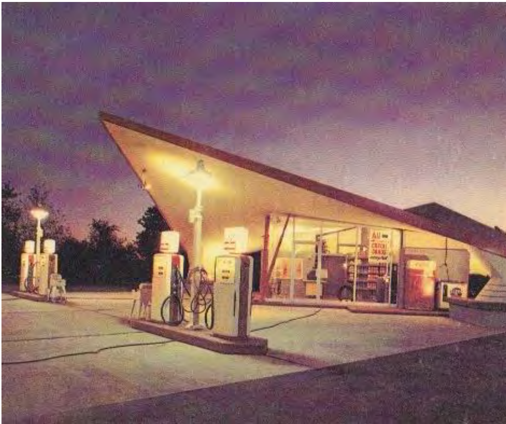
Figure 7: Vickers Petroleum Service Station in Hayesville shortly after it was constructed. This photo shows that there were storefront systems at both the front and rear facades of the interior store space. Photo from "50 th '1918...": page 13.
