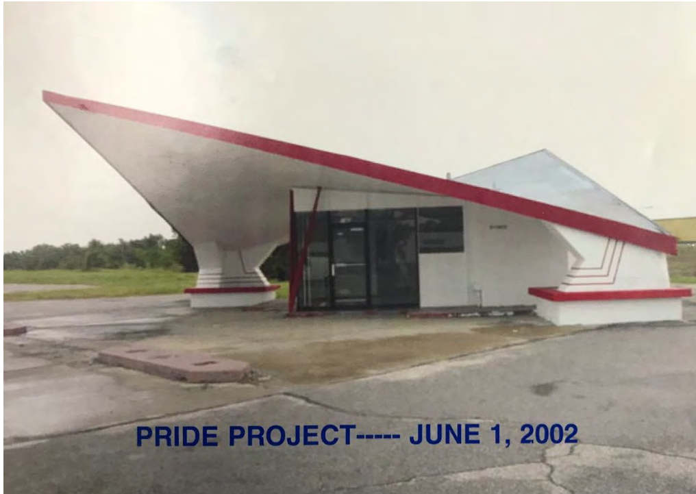
Figure 5: After the Pride Project in 2002. A first reconstruction was built in 1999 with a wood-framed bulkhead above the storefront. Volunteers painted the building as part of the Pride Project. Photo courtesy of Rosemarie Corby.
