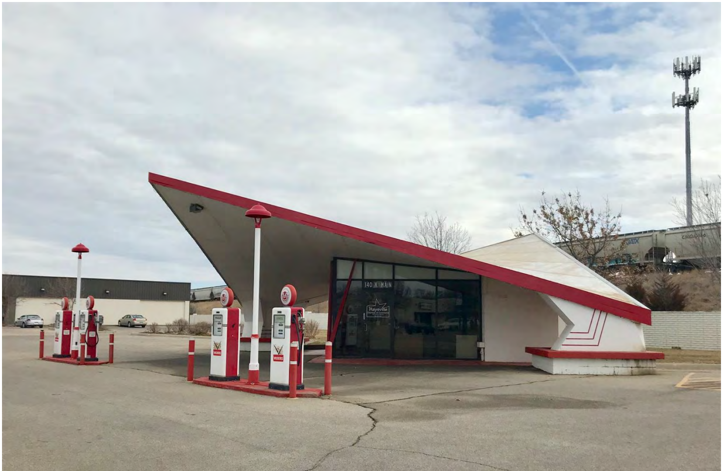
Photo: The two axes of the building can be observed. The batwings open to the east and west.
