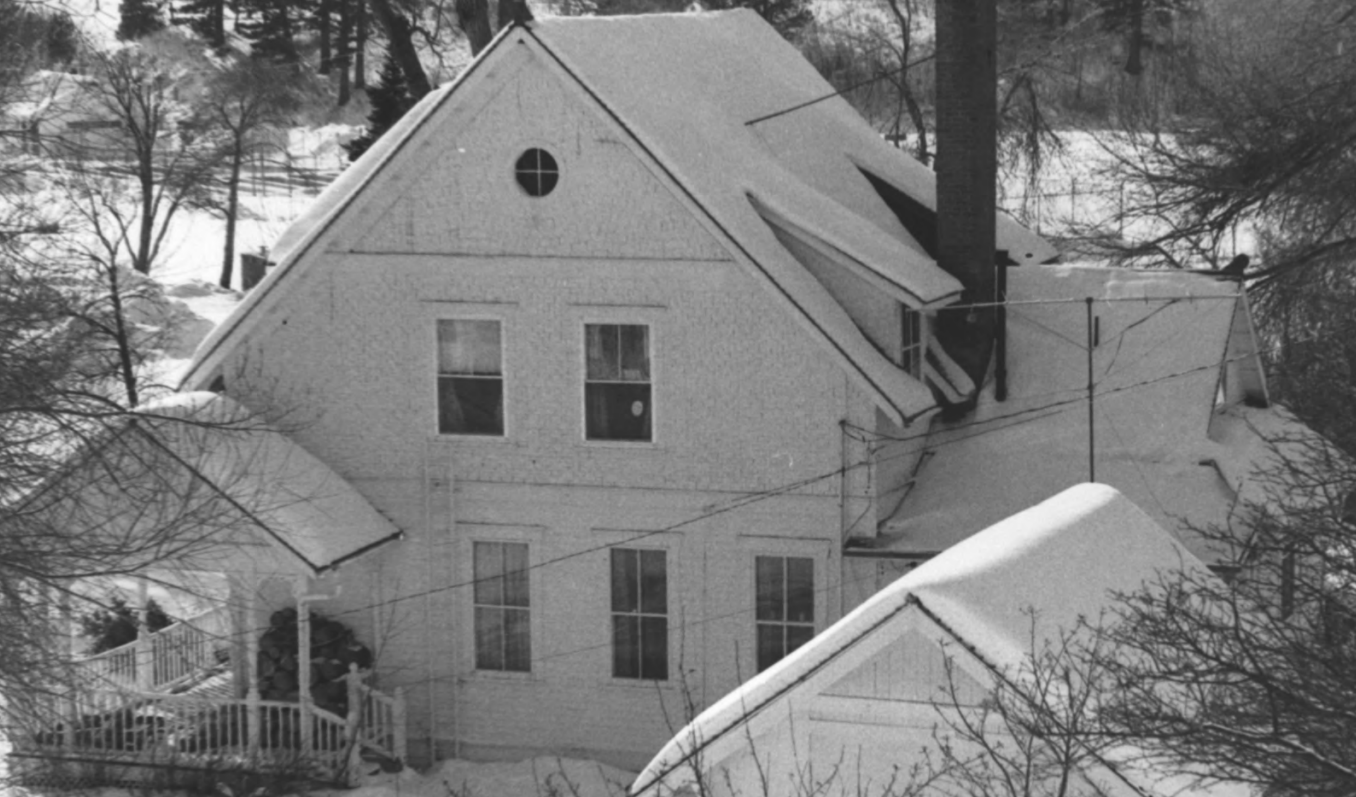
Bozeman Fish Cult. Devlpt. Ctr. Supt.'s House, also bath cottage North Elevation Kingston Heath, MT. St. Hist. Soc. 1978
