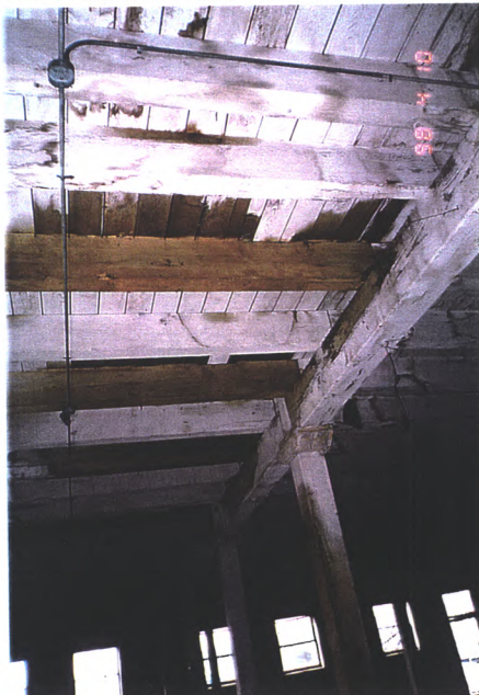
Below: Post and beam detail all other floors
