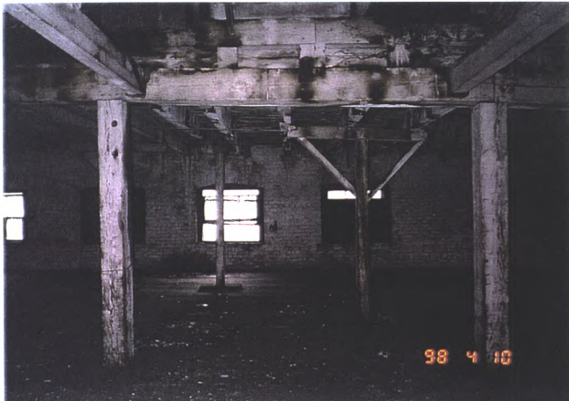
Above: Post and beam detail—fifth floor
