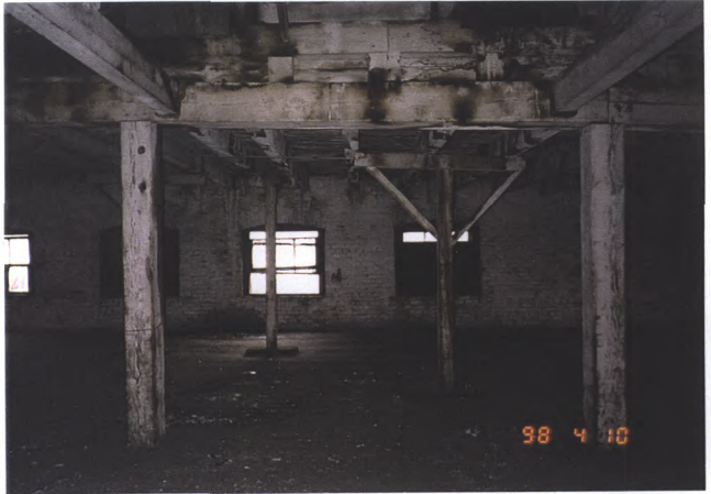
Above: Post and beam detail—fifth floor
