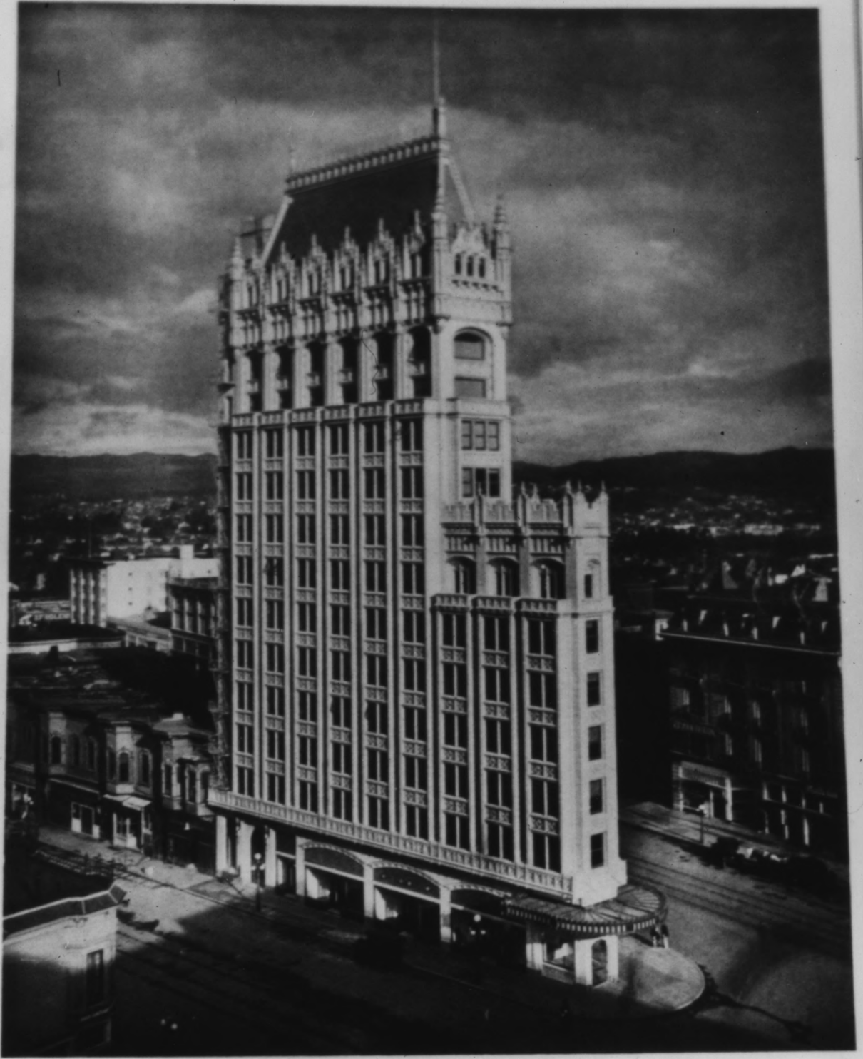
West Elevation, Federal Realty Building, Oakland Benjamin Geer McDougall, Architect, San Francisco
