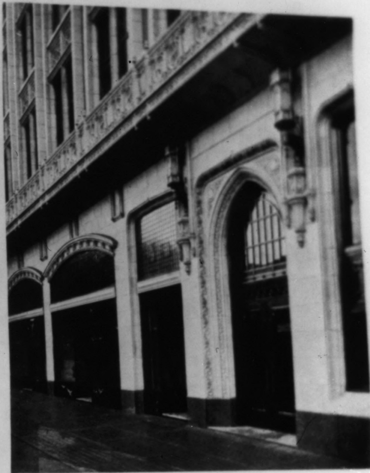
Broadway Entrance and Stairs
