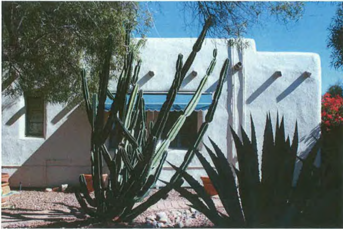
Photo 3 of 12. Partial west elevation, south wing detail
