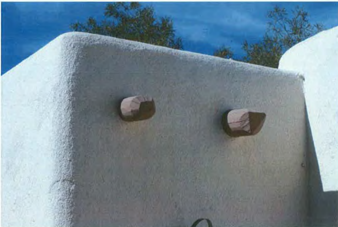
Photo 6 of 12. Partial north elevation, viga and wall detail.
