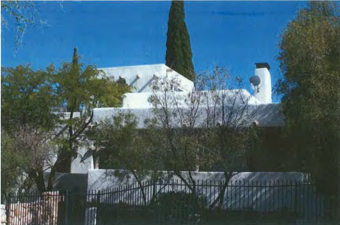
Photo 1 of 12. Partial west elevation, looking east
