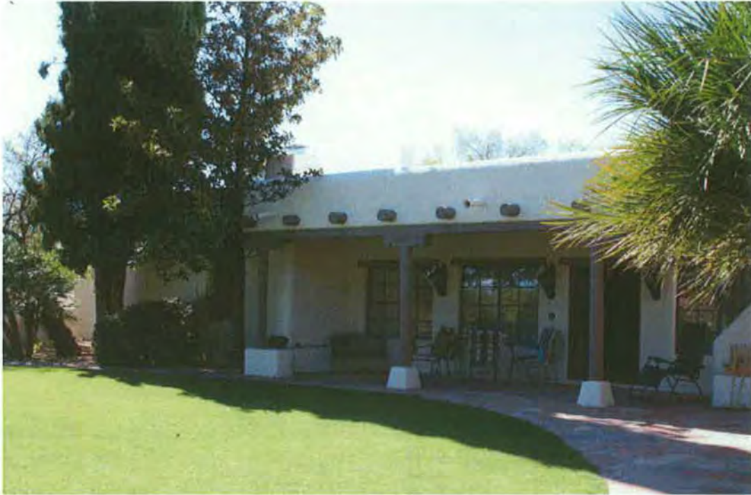
Photo 5 of 12. Partial east elevation, porch detail.
