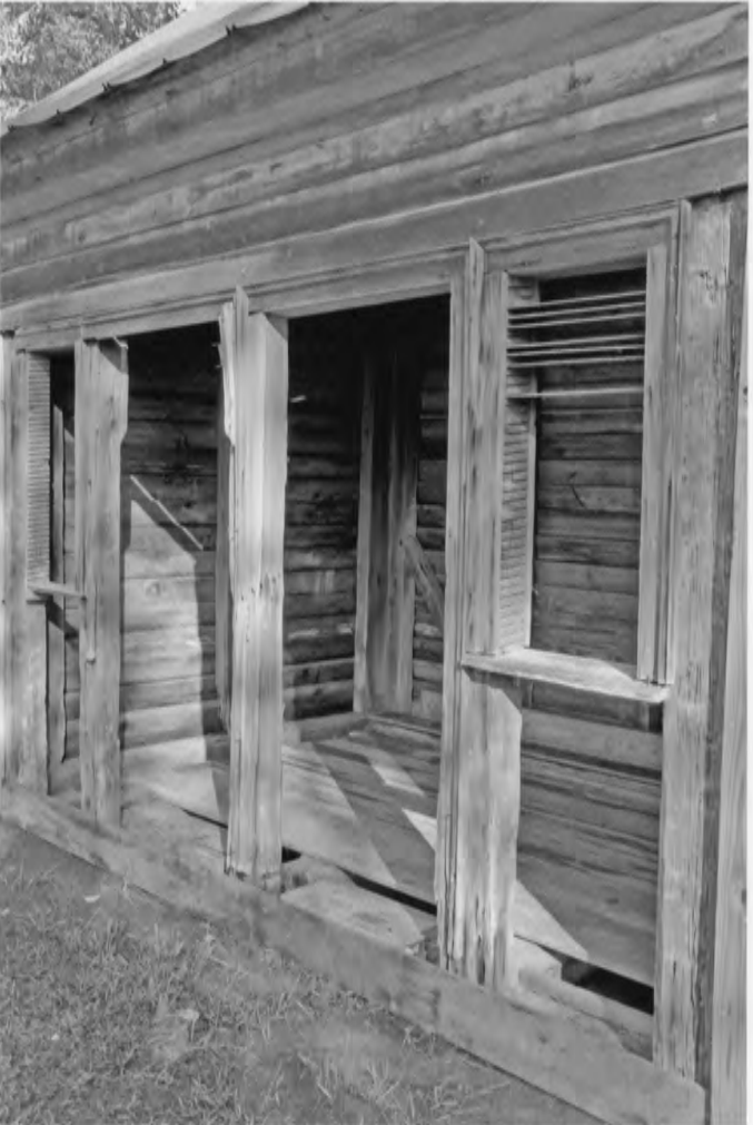
41. McLaurin-Roper-McColl Farmstead 1104 Laurin Willis Road, Clio vicinity Marlboro County, South Carolina 1820s Outbuilding, Facade, Showing Slat Windows, October 2008
