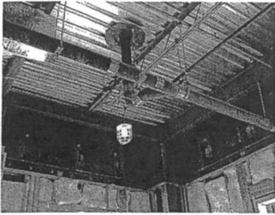
**Figure 110** Low roof parapet bracing extending under roof deck and fastened to limestone water table on inside face at existing building
