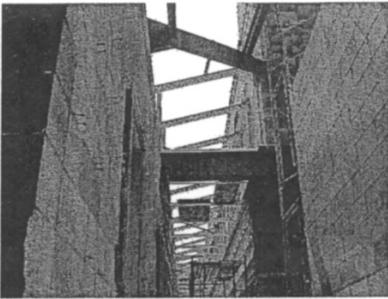
Figure 29 Hip framing at low roof
