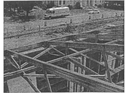
Figure 42 Exterior wall supporting low roof trusses – See item 13
