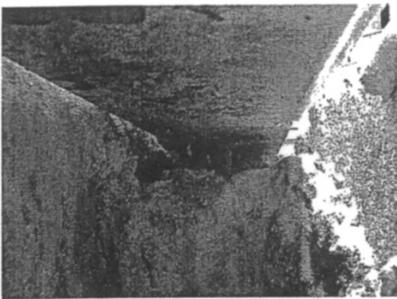
Figure 55 Typical embed plate at interior wall at low roof. Void between grout and plate - See item 15
