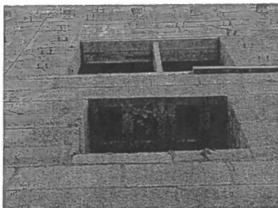
Figure 68 UngROUTED lintel over louver opening – See item 24
