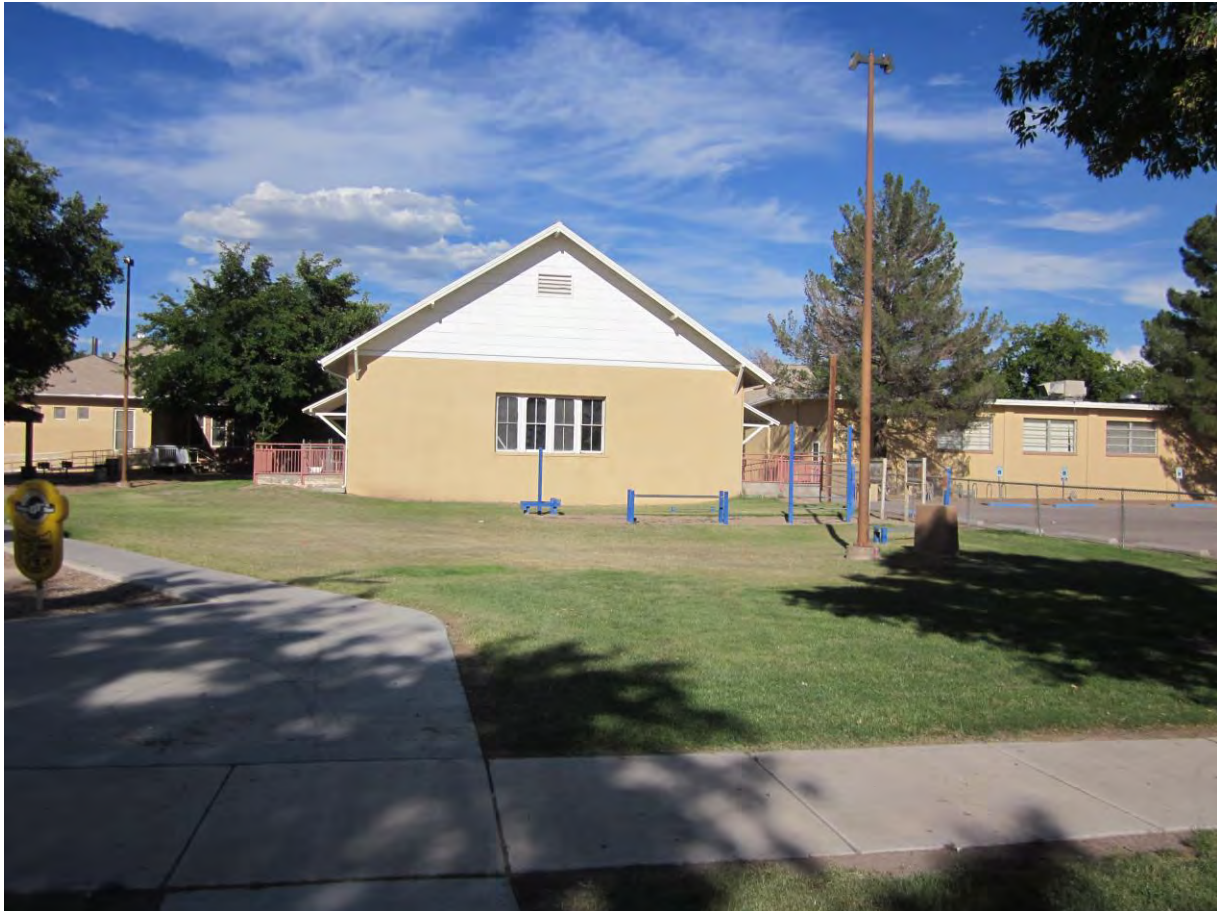
Photo 8 of 26. Rear elevation with classroom wing, 1934 (left), auditorium (center), and cafeteria (right), photographer facing northeast.
