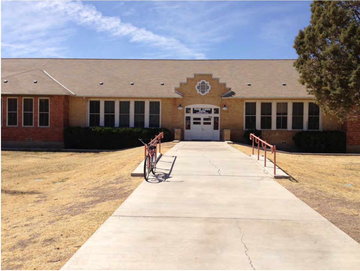
Photo 2 of 26. Main elevation, detail, photographer facing southwest.
