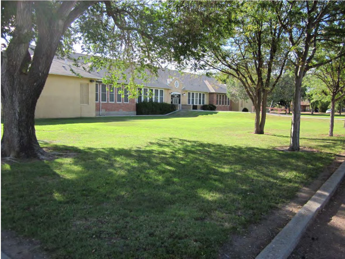
Photo 1 of 26. Main (west) façade, photographer facing west.
