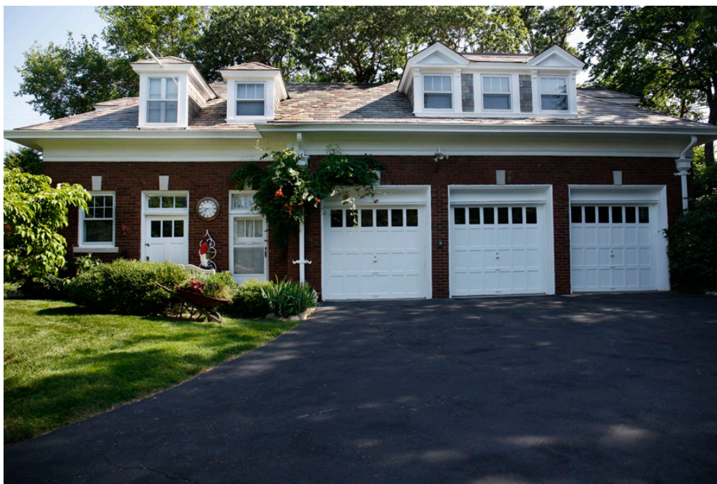
Photograph 13. Carriage house façade.
