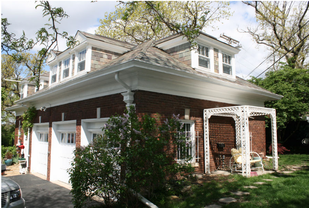
Photograph 15. South and east carriage house elevations.
