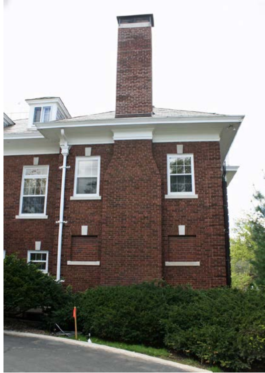
Photograph 4. West portion of north façade.
