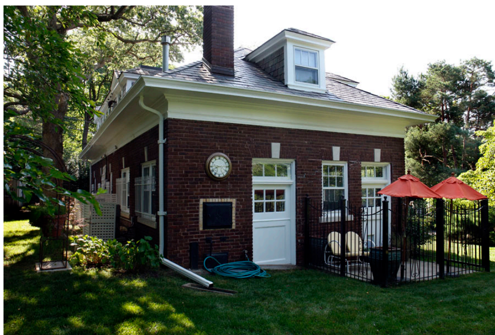
Photograph 14. West and north carriage house elevations.
