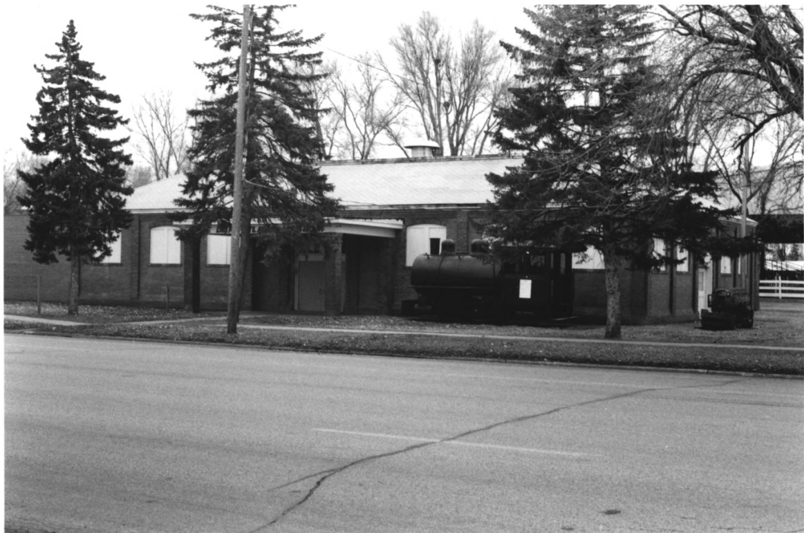
Dairy Building, Beadle County, S.D., No. 1
