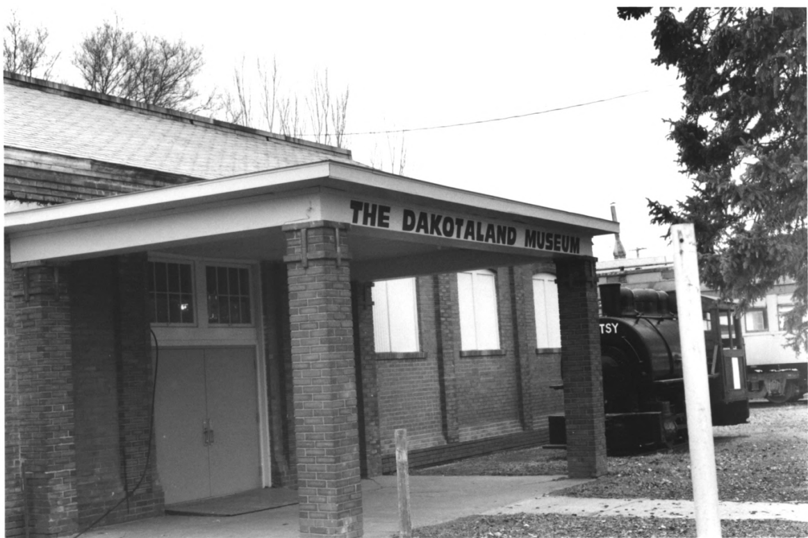
Dairy Building, Beadle County, S. D., No. 3
