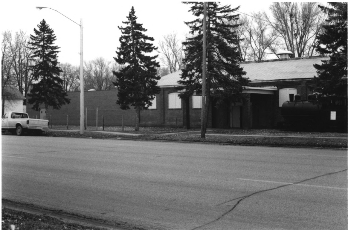
Dairy Building, Beadle County, S.D., No. 2
