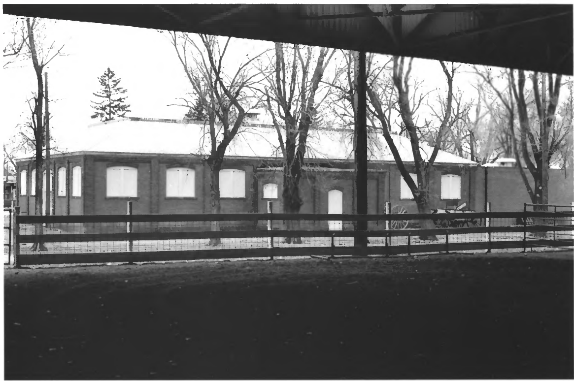
Dairy Building, Beadle County, S.D., No. 4
