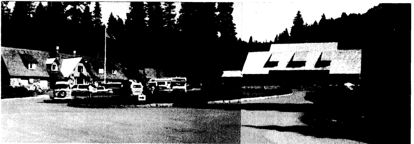
Administrative plaza looking north from the entrance; Ranger Dormitory (left), Administration Building (right).
