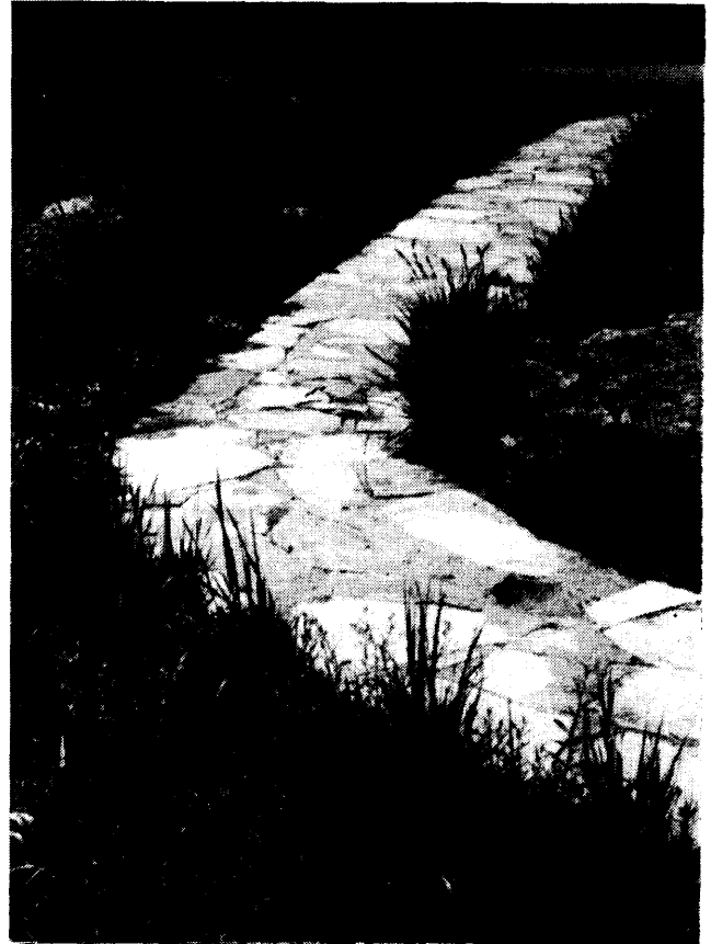
Flagstone walkway, Superintendent's Residence, west entrance.
