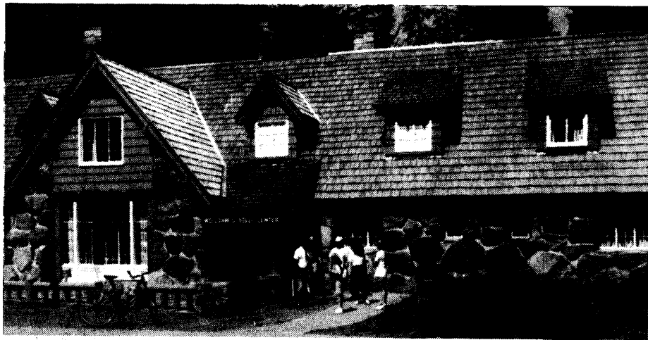
Ranger Dormitory (William G. Steel Center); current visitor center.
