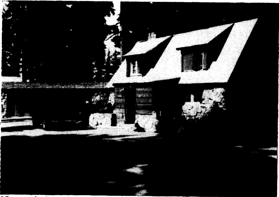
View south along spur road showing typical post WW II snow tunnel addition and widened road bed, 1990
