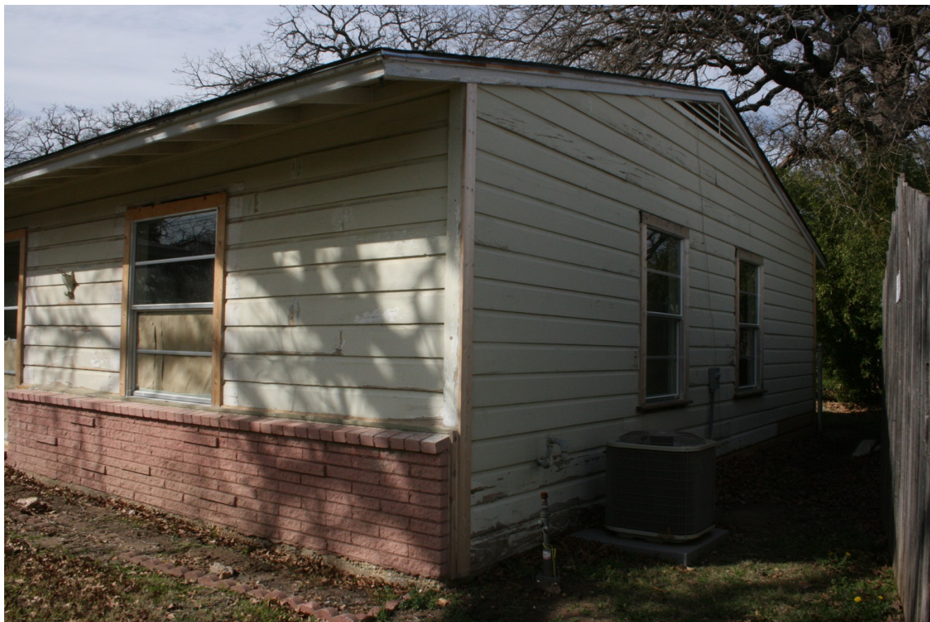
Paine House – southeast oblique Camera facing northwest Photo 3
