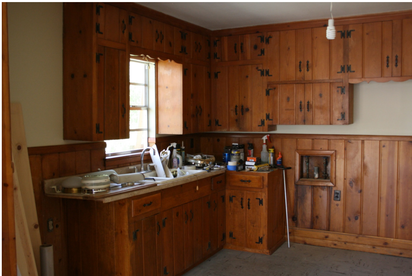
Paine House – kitchen Camera facing northeast Photo 6
