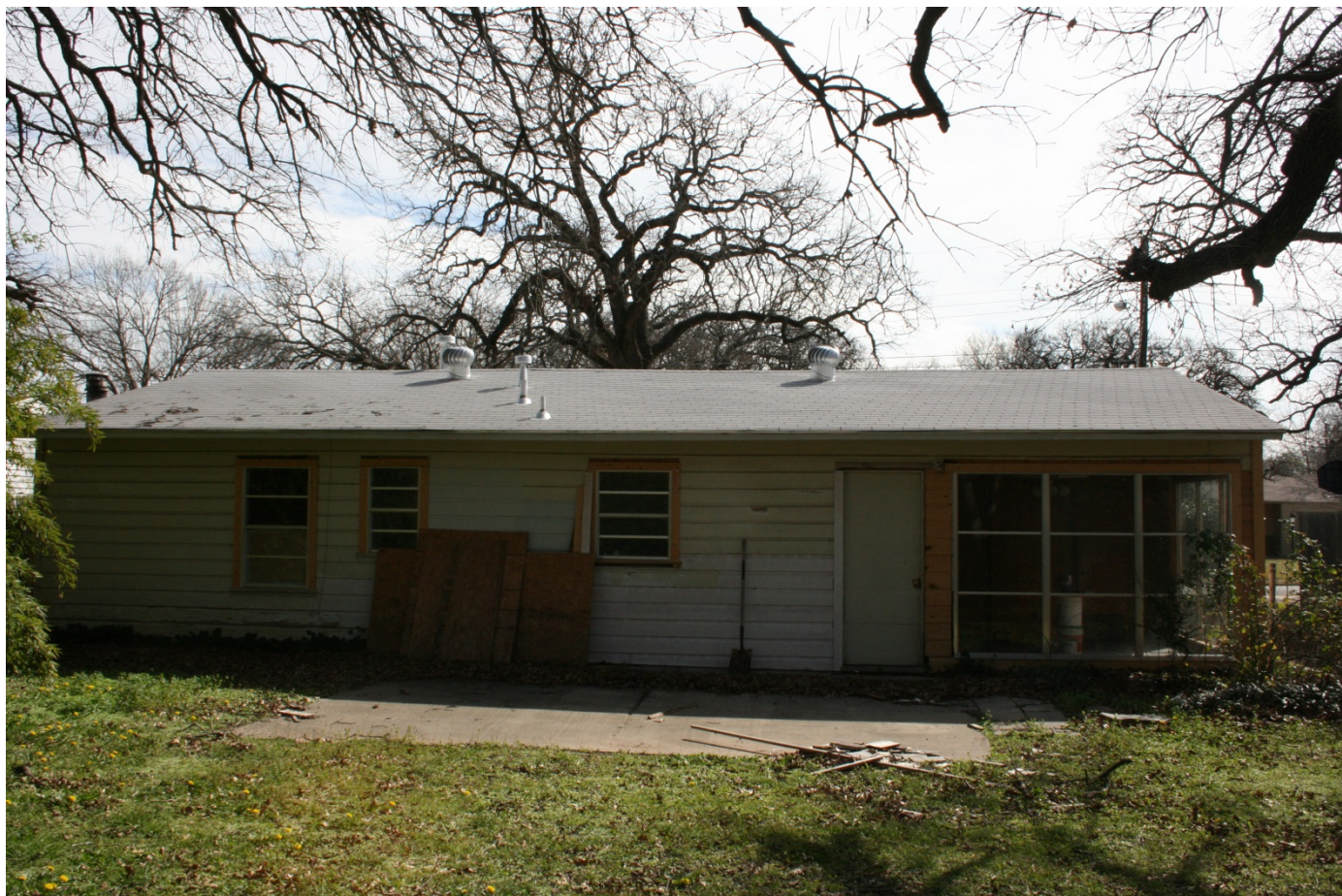
Paine House – north elevation Camera facing south Photo 4
