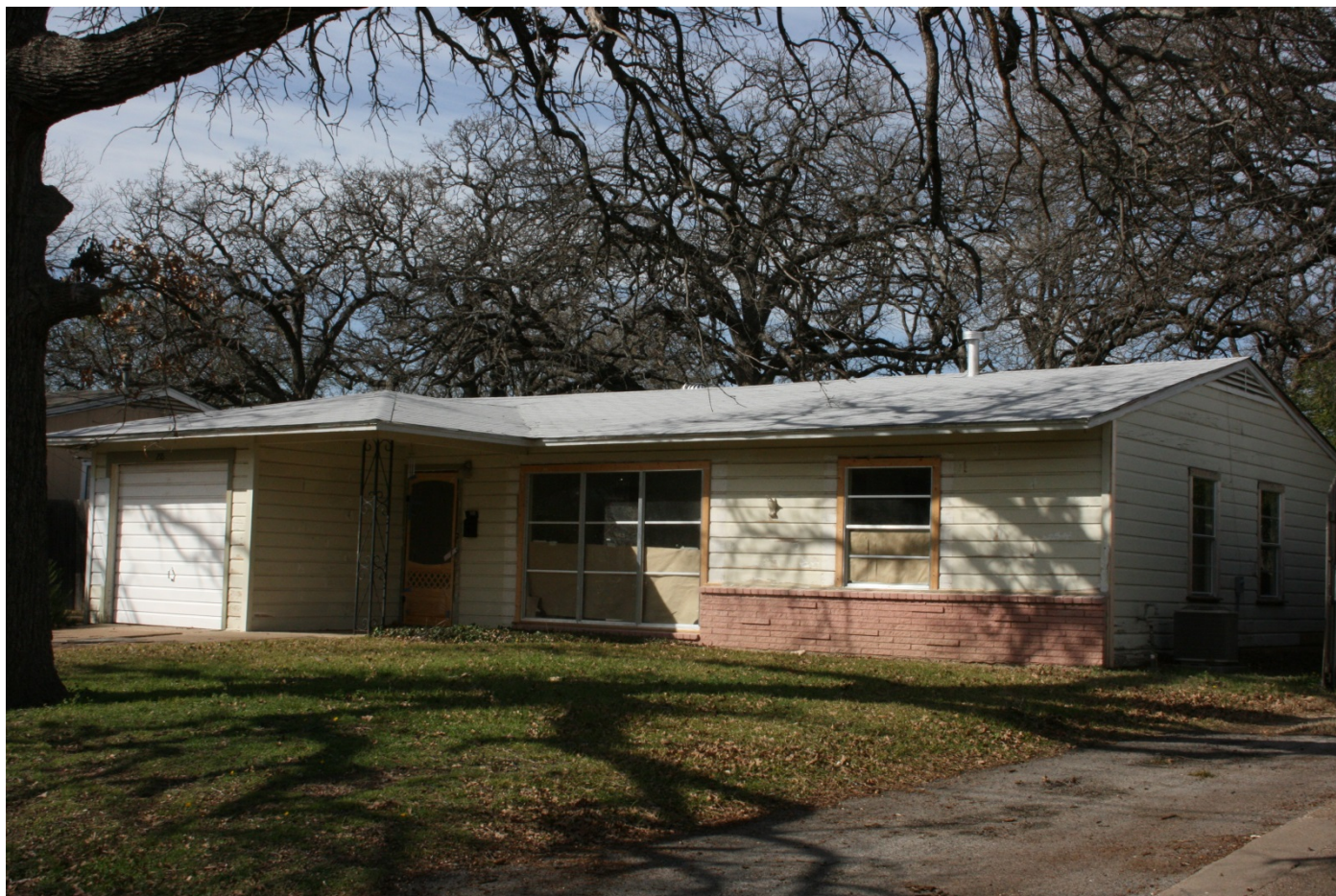
Paine House – south and east elevations Camera facing northwest Photo 2
