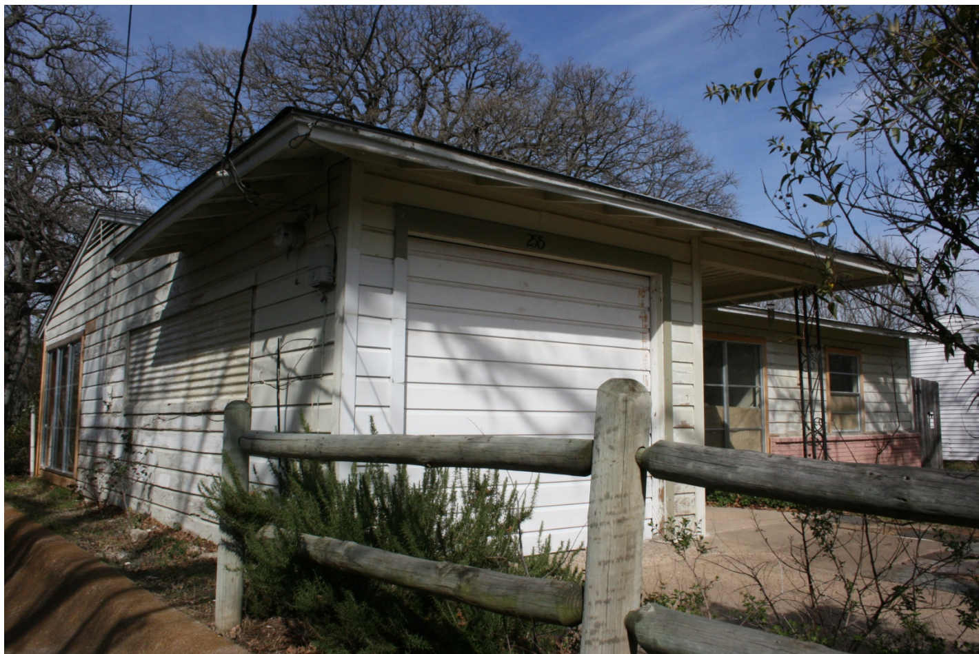
Paine House – Southwest oblique Camera facing northeast Photo 5
