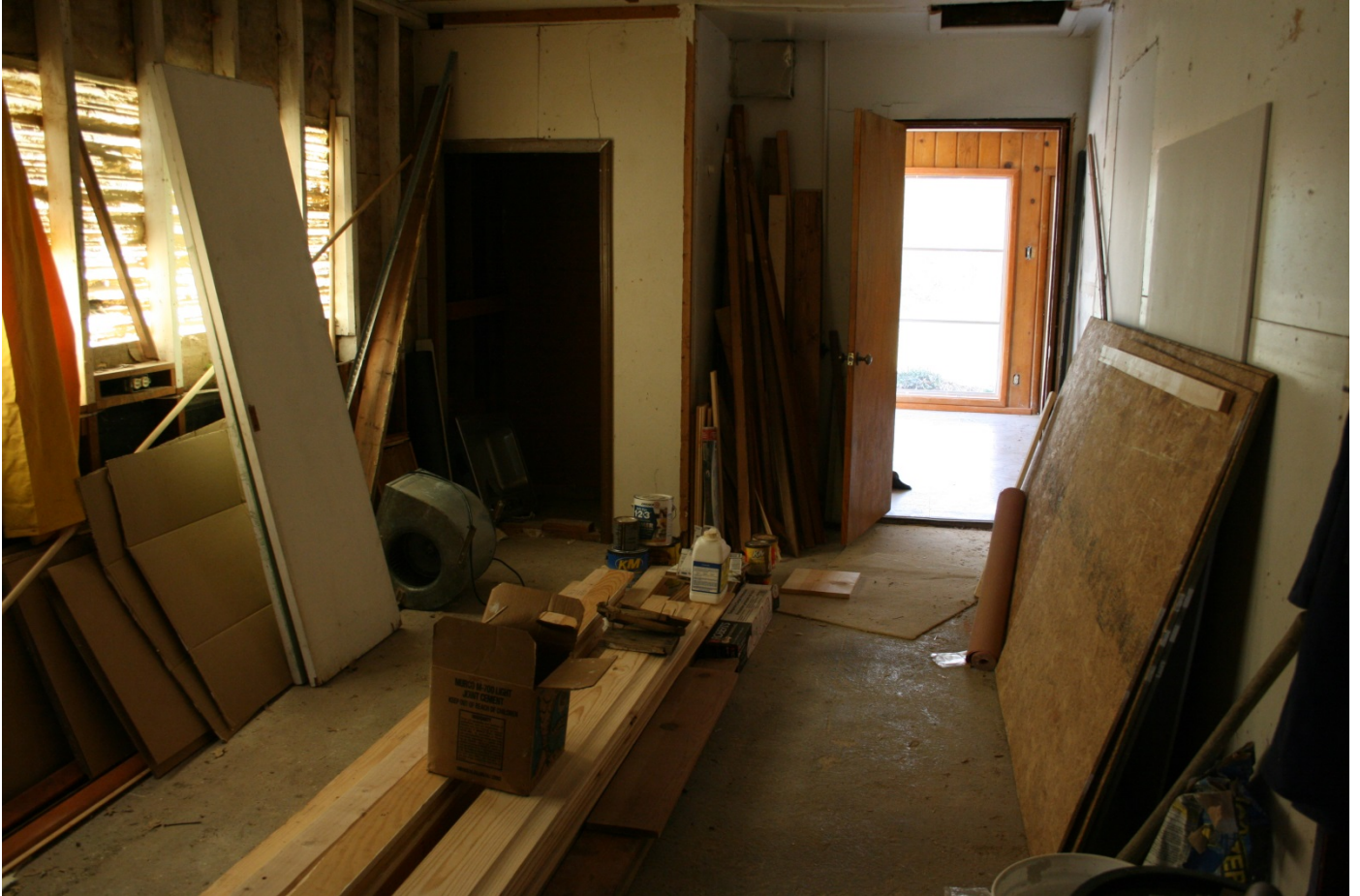
Paine House – garage interior Camera facing north Photo 9
