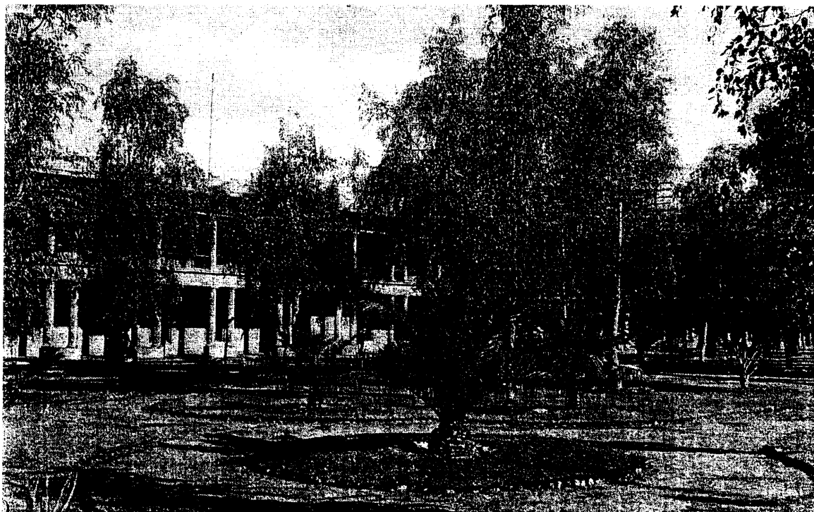
H9: Santa Fe Park in the foreground and the El Garces/Needles Depot at the background, ca. 1910. (Courtesy of Architect Milford Wayne Donaldson, FAIA historic postcard collection)
