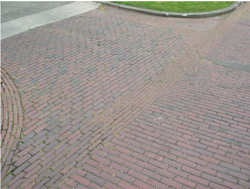
3 of 6 – N 9 th Street at 900 Block, Detail of brick gutter and transition to alley.
