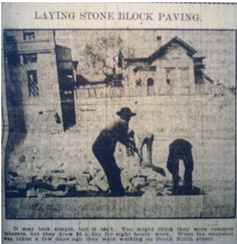
Laying of Wilkeson sandstone setts on South 9 th Street. Tacoma Daily Ledger , 05/19/1907, pg. 23.
