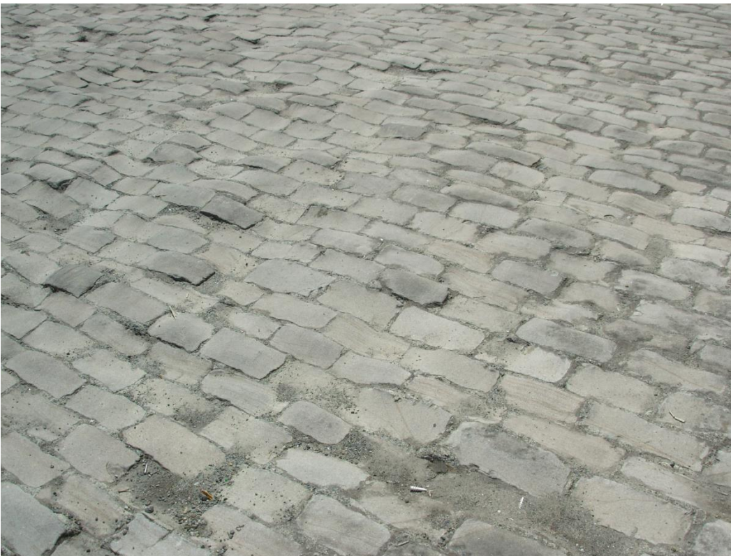
5 of 6 – N 11 th Street at 1000 Block, detail of sandstone pavers showing condition.
