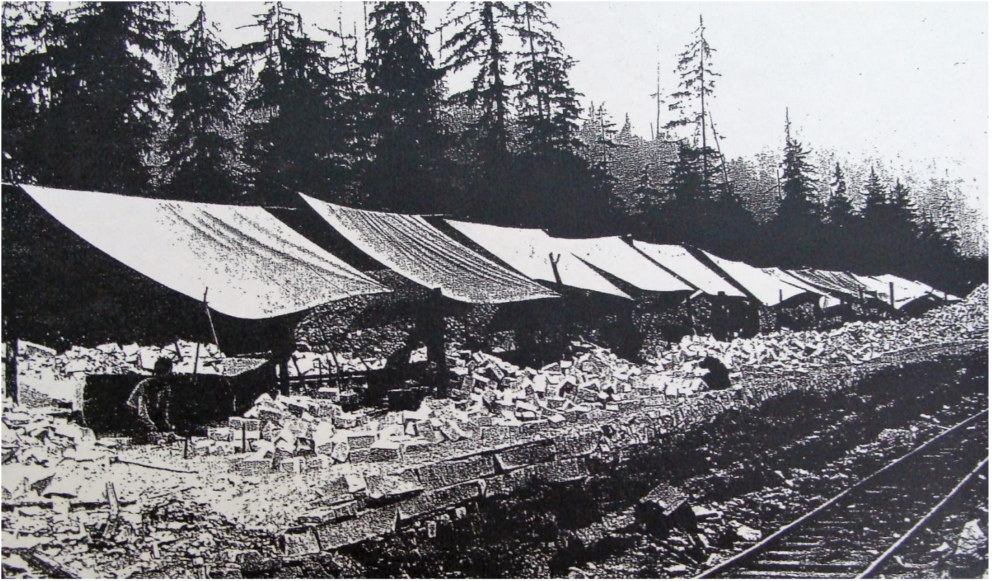
Sett production at Wilkeson Sandstone Quarry, date unknown, Lee Pickett Collection, University of Washington.
