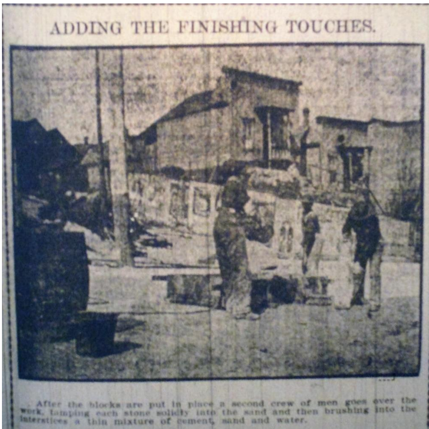
Laying of Wilkeson sandstone setts at unidentified location. Tacoma Daily Ledger , 05/19/1907, pg. 23.
