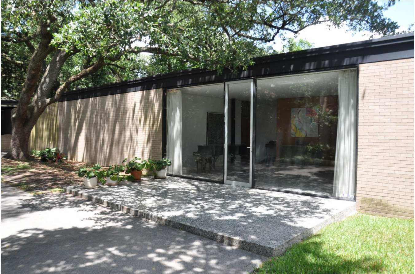
Photo 3 Southeast elevation. Detail of front entrance, camera facing northwest.
