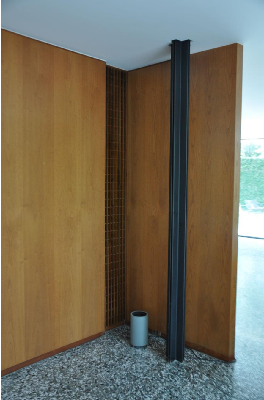
Photo 11 Detail of steel column and return air register, camera facing northeast.
