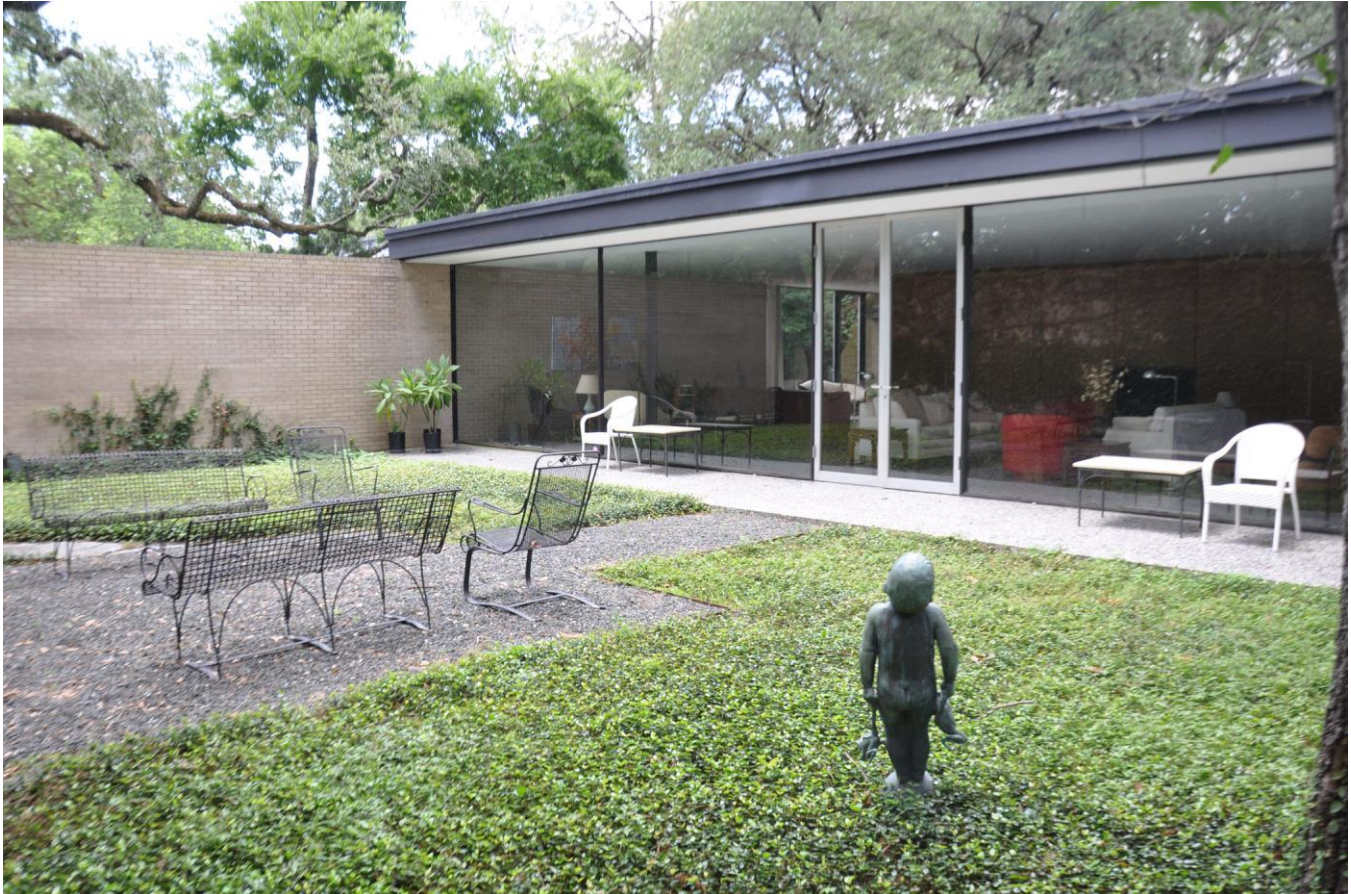
Photo 5 Northeast (courtyard) elevation, camera facing southwest.
