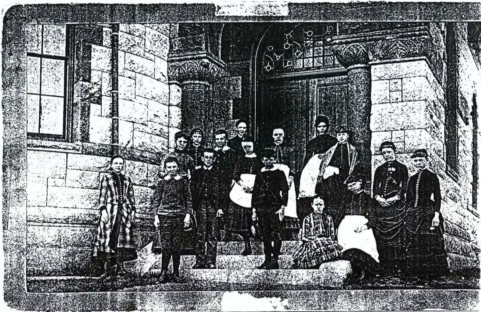
UPPER SCHOOL, AUTUMN TERM 1886 GOODNOW MEMORIAL BUILDING, LIBRARY ENTRANCE PRINCETON, MASSACHUSETTS
