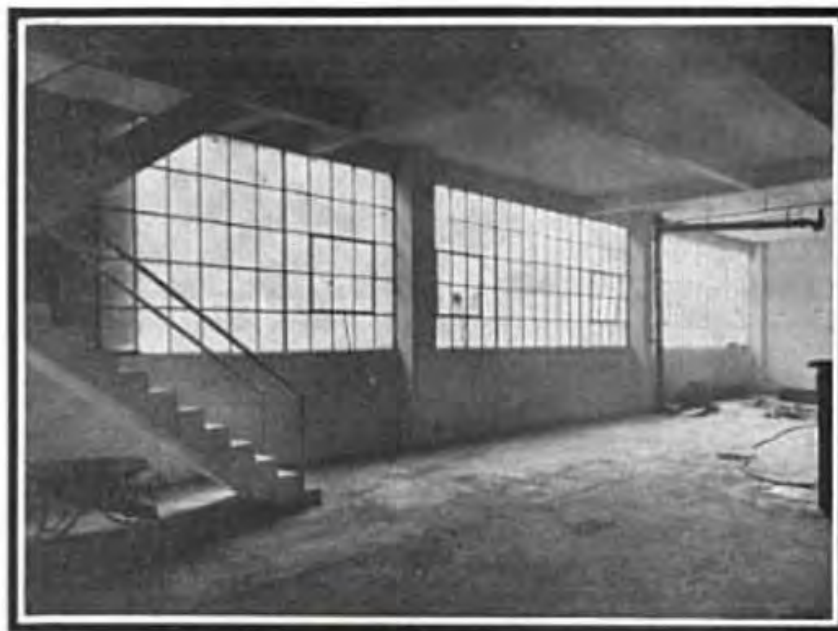
Basement of Brown's Garage, Showing Excellent Lighting Arrangement.
