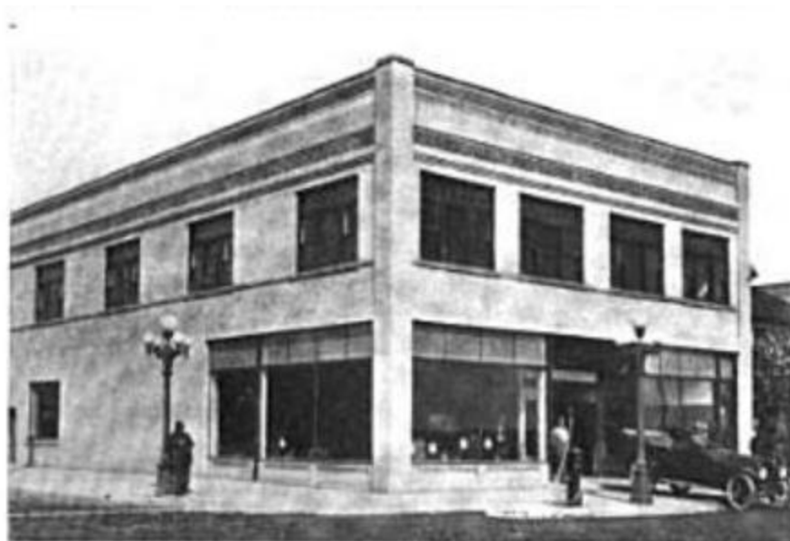
Fig. 26—Turner's Garage, Dickenson, N. D.
