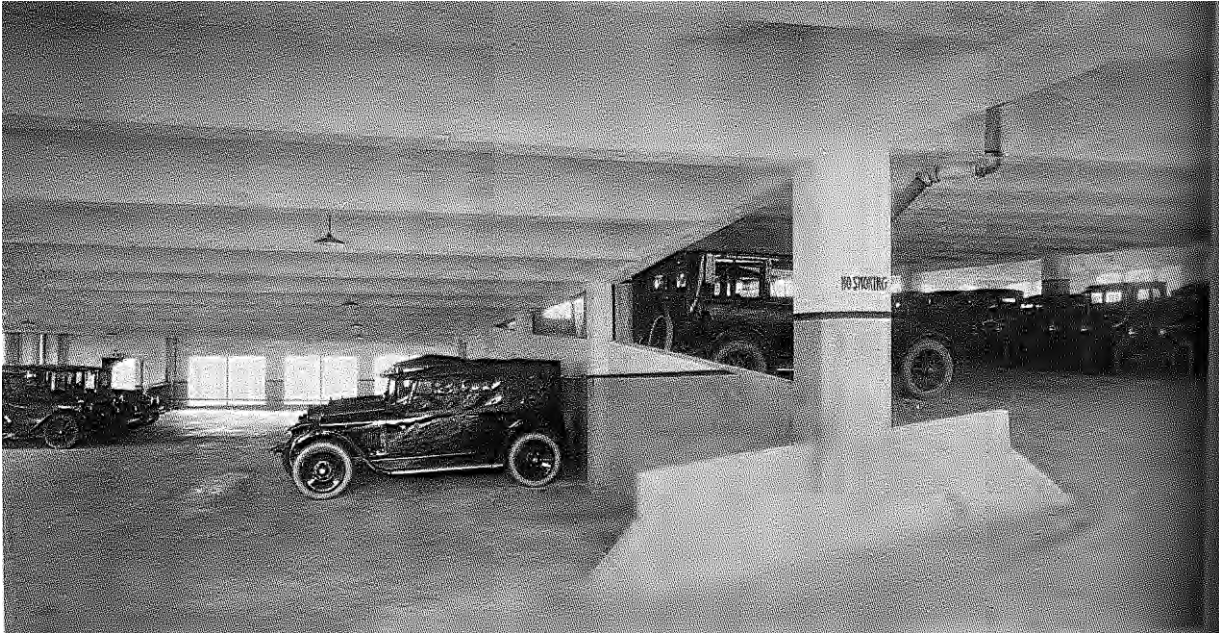
Figure 16: Slope Floor Design, Fort Shelby Garage, Detroit. Source: The Architectural Forum 46:3 (March 1927).
