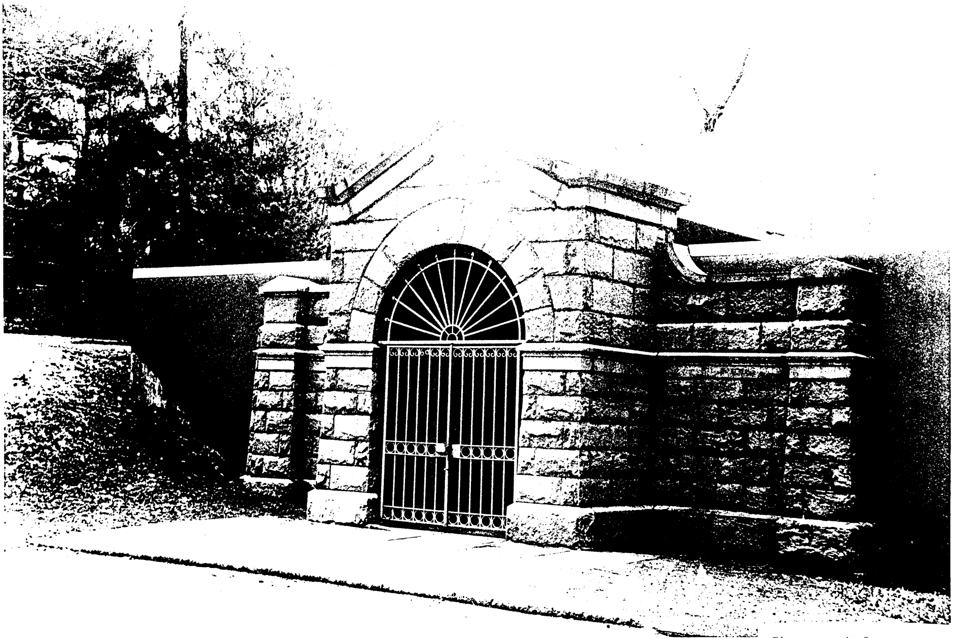
Photograph 3 Crematory View southeast
