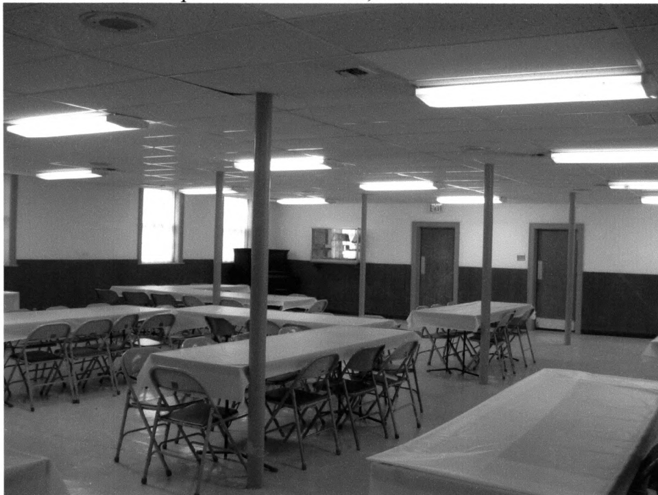
Social Hall in basement underneath sanctuary View to the South
