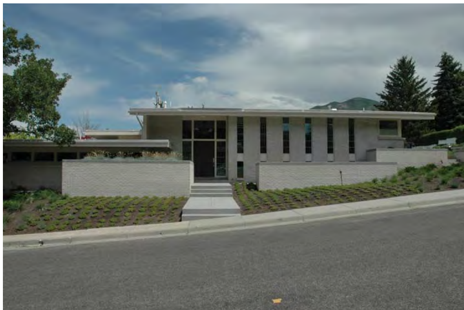
Photograph 2 of 10 South elevation of Price House. Camera facing north.
