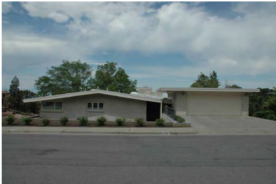
Photograph 8 of 10 East elevation of Price House, garage on right. Camera facing west.
