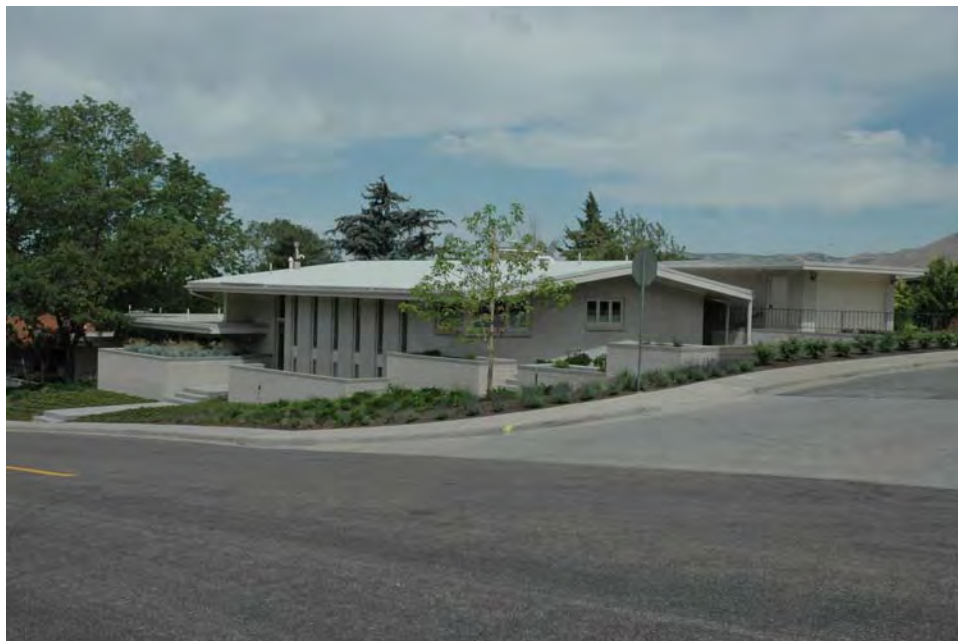
Photograph 1 of 10 South and east elevations of Price House. Camera facing northwest.
