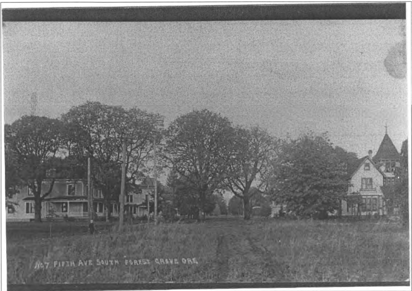
Figure 7: Looking West down 15 th Ave (formerly 5 th Ave. ) circa 1902. Ivan Marble House (1890) at 1504 Elm can be seen on the right side of the photograph; the Watts House (1904) at 2434 15 th Avenue can be seen in the foreground on the left side of the photo. The Bailey House (1892) can be seen behind the Watts House located at 2422 15 th Avenue.
