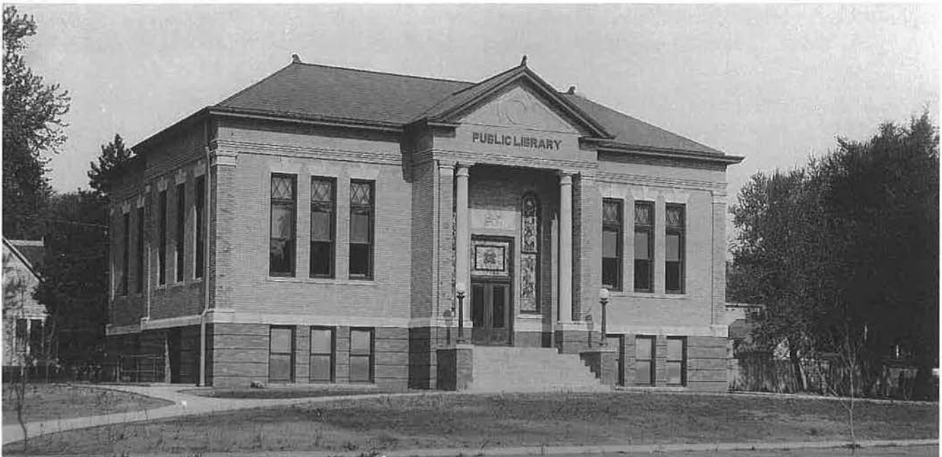
Figure 12: 1909 Looking northwest at completed Clarinda Carnegie Library. Judy Aulik Collection.
