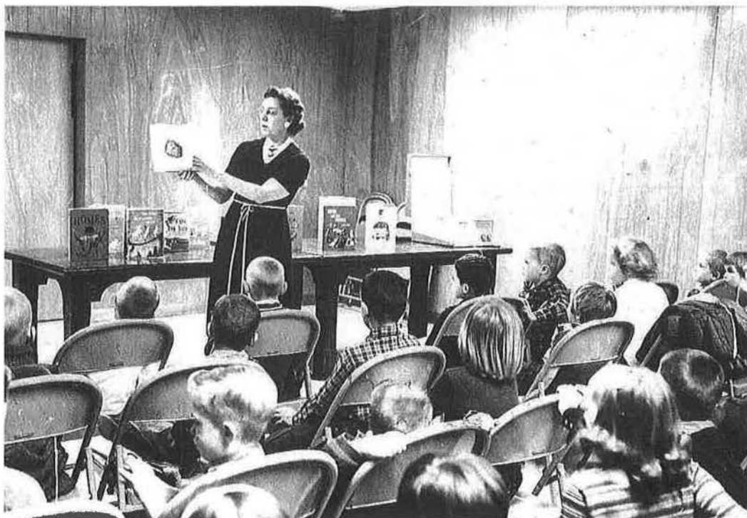
Figure 22: 1950s Auditorium in the basement. Clarinda Public Library Collection.
