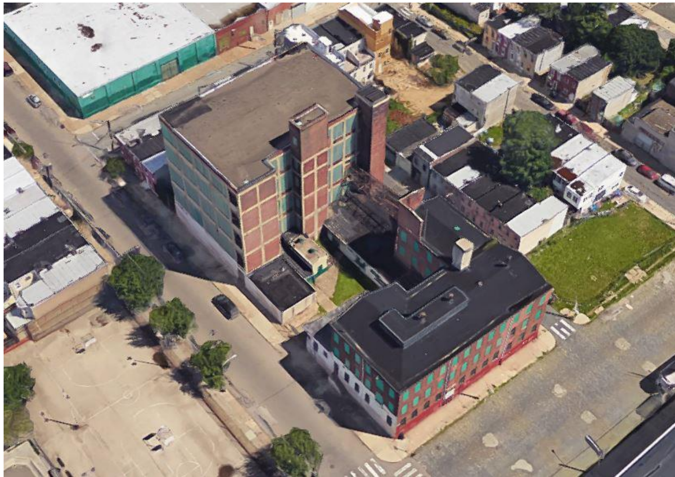
Figure 21 – Current Aerial View, Looking Northwest
