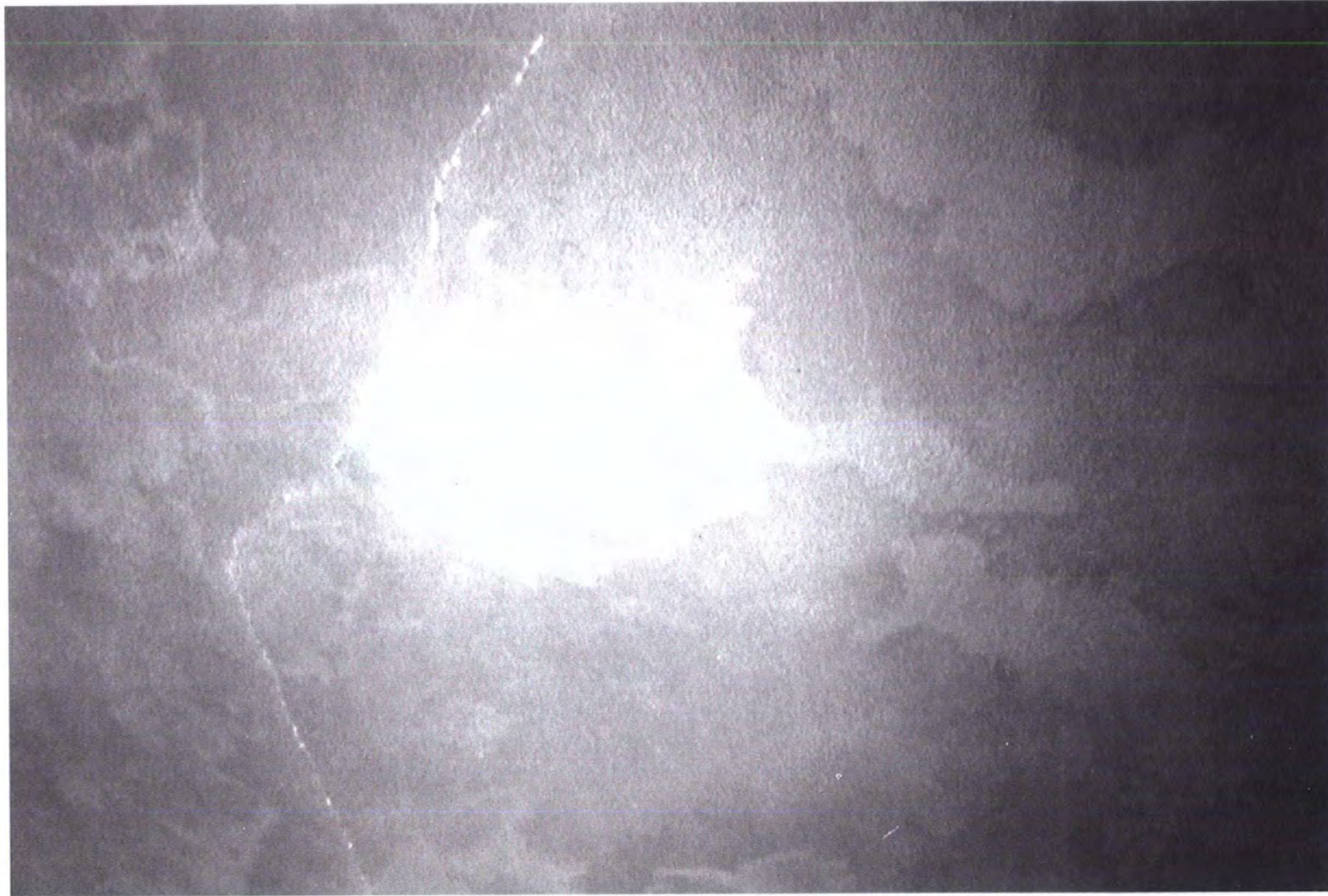
ILLUSTRATION # 5 Portion of now hidden cloud-decorated living room ceiling, seen while sheetrock was removed during repairs in 1996.
