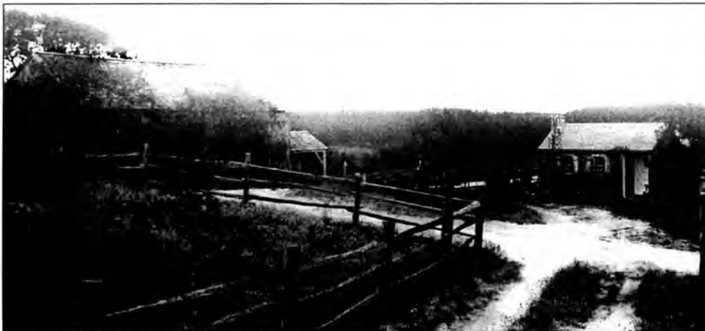
1942 Photograph of Atwood-Higgins landscape, looking northeast toward Barn and Guest House. Source: George K. Higgins's journal, on file, NPS Salt Pond Visitor Center, Eastham, MA.
