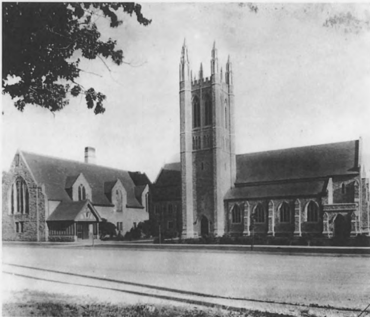
H0003. View of west/north elevation following 1925 addition, no date
