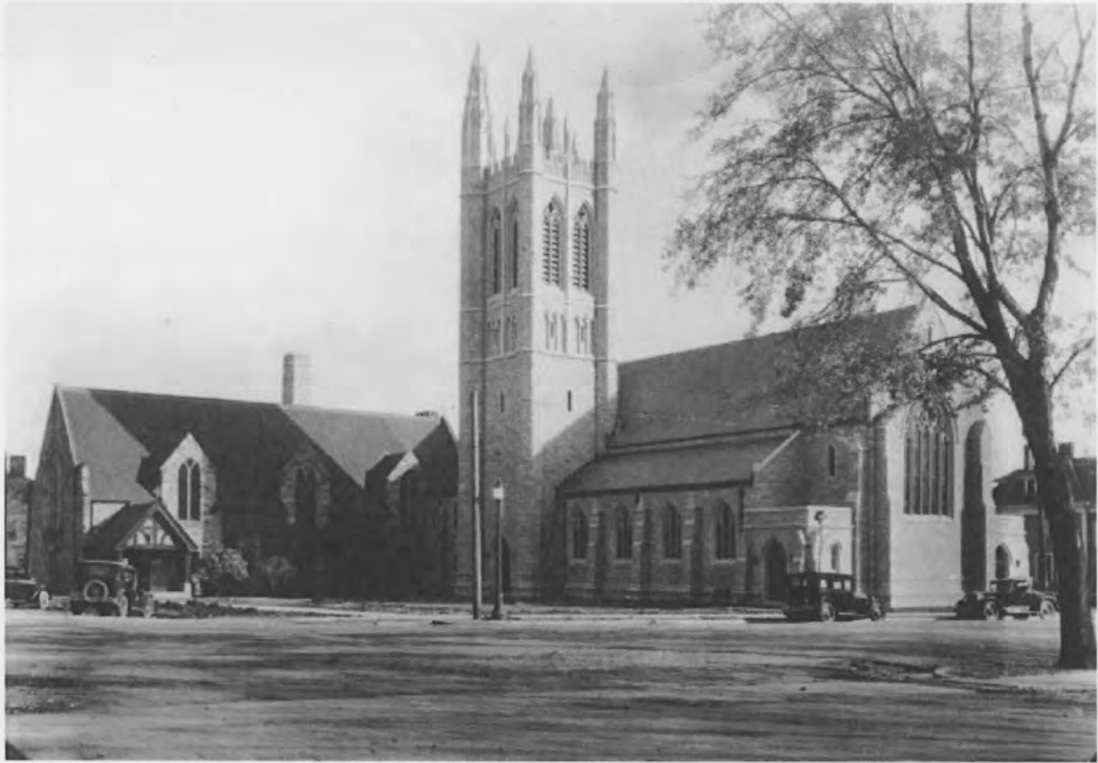
H0004. View of west/north elevations, ca. 1925-1930
