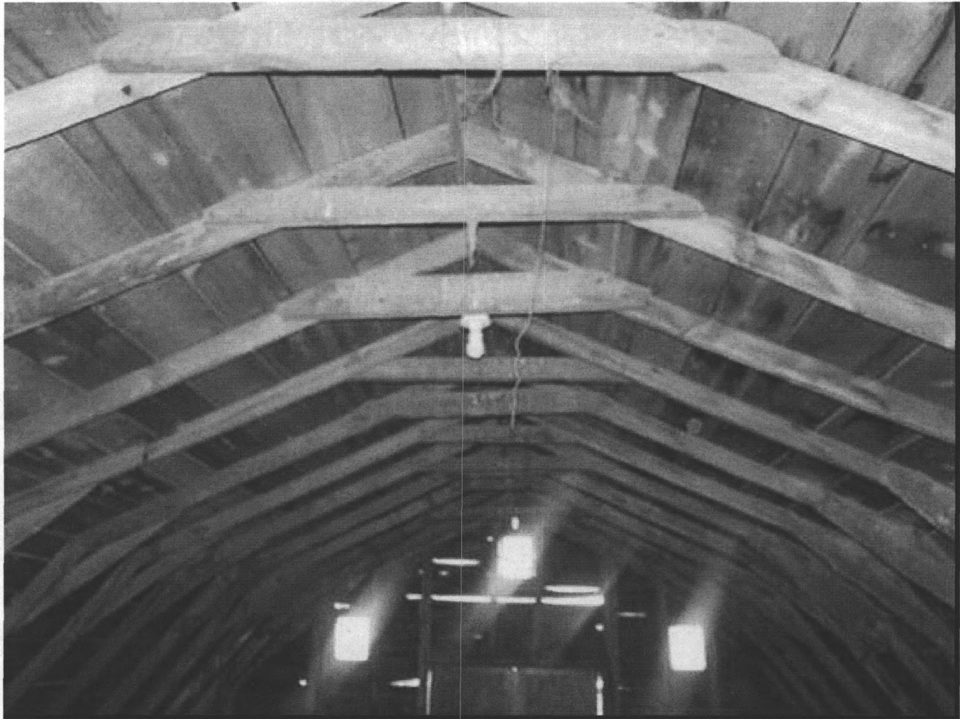
Direction: East. Description: Demonstrating the original barn roof truss system. MT_BigHornCounty_YoungAlvinBarnandCabinHistoricDistrict_0023
