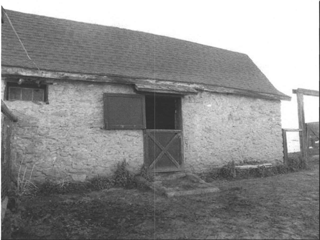
Direction: North. Description: South elevation of the original barn. MT_BigHornCounty_YoungAlvinBarnandCabinHistoricDistrict_0015
