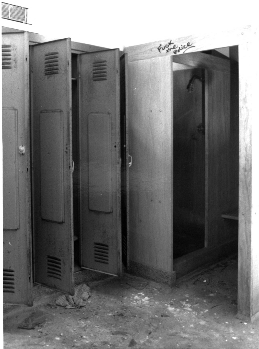
CULVER UNION HOSPITAL, CRAWFORDSVILLE, MONTGOMERY COUNTY, IN - PHOTO NO. 36
