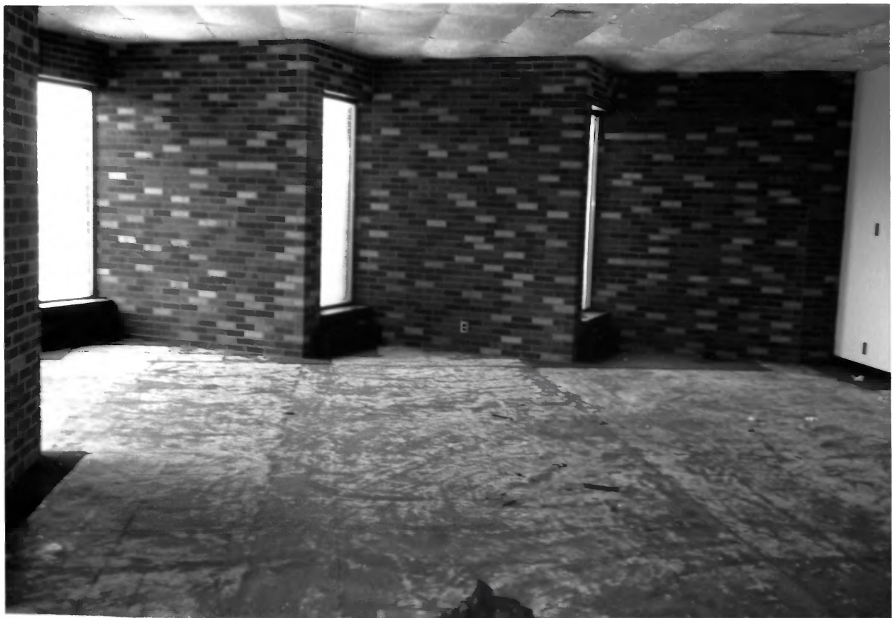
CULVER UNION HOSPITAL, CRAWFORDSVILLE, MONTGOMERY CO; IN- PHOTO NO. 29
