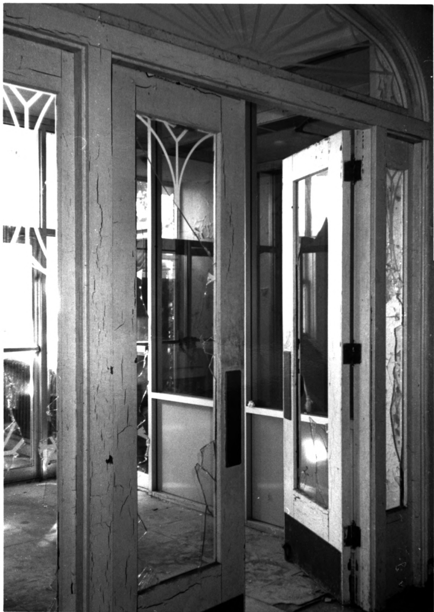
CULVER UNION HOSPITAL, CRAWFORDSVILLE, MONTGOMERY CO, IN - PHOTO No. 21
