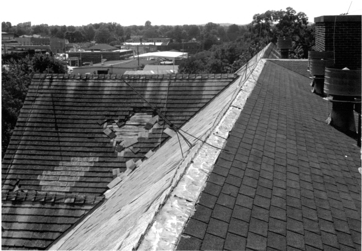
CULVER UNION HOSPITAL, CRAWFORDSVILLE, MONTGOMERY CO., IN. PHOTO No. 38
