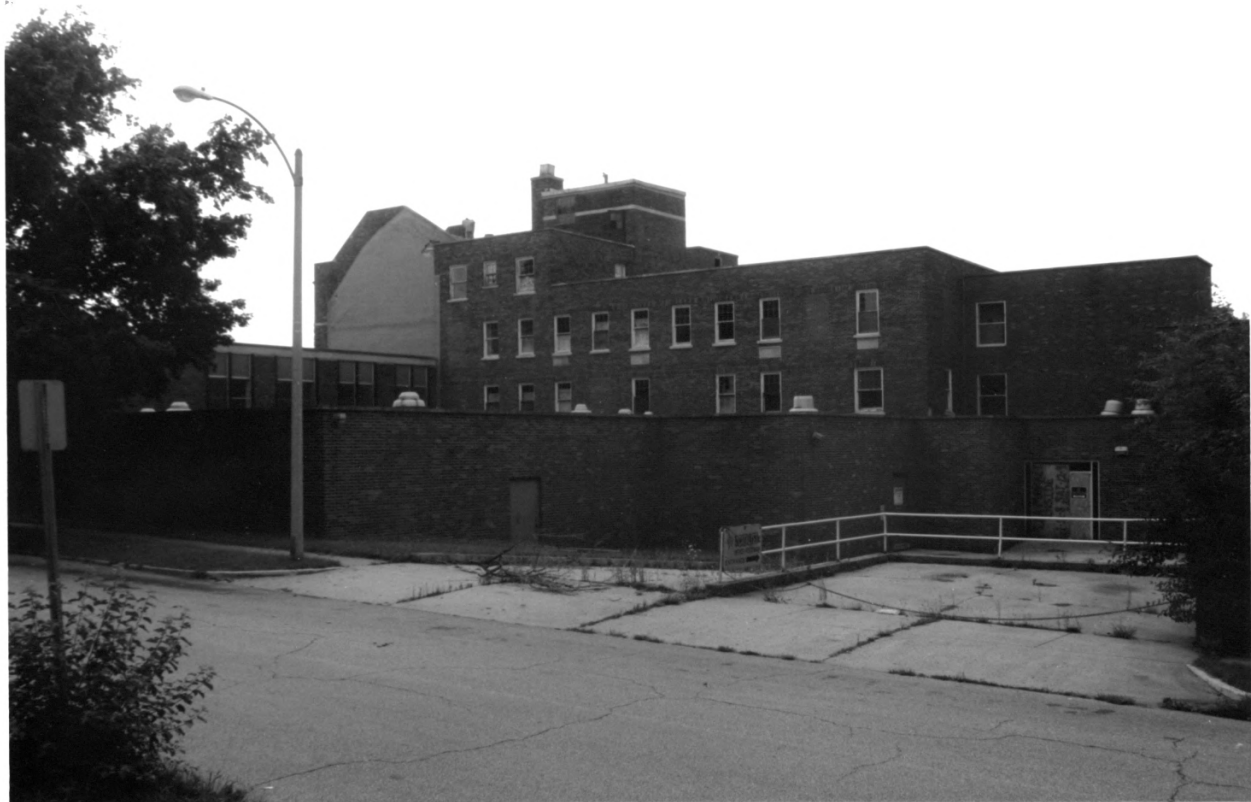
CULVER UNION HOSPITAL, CRAWFORDSVILLE, MONTGOMERY CO., IN - PHOTO NO. 13
