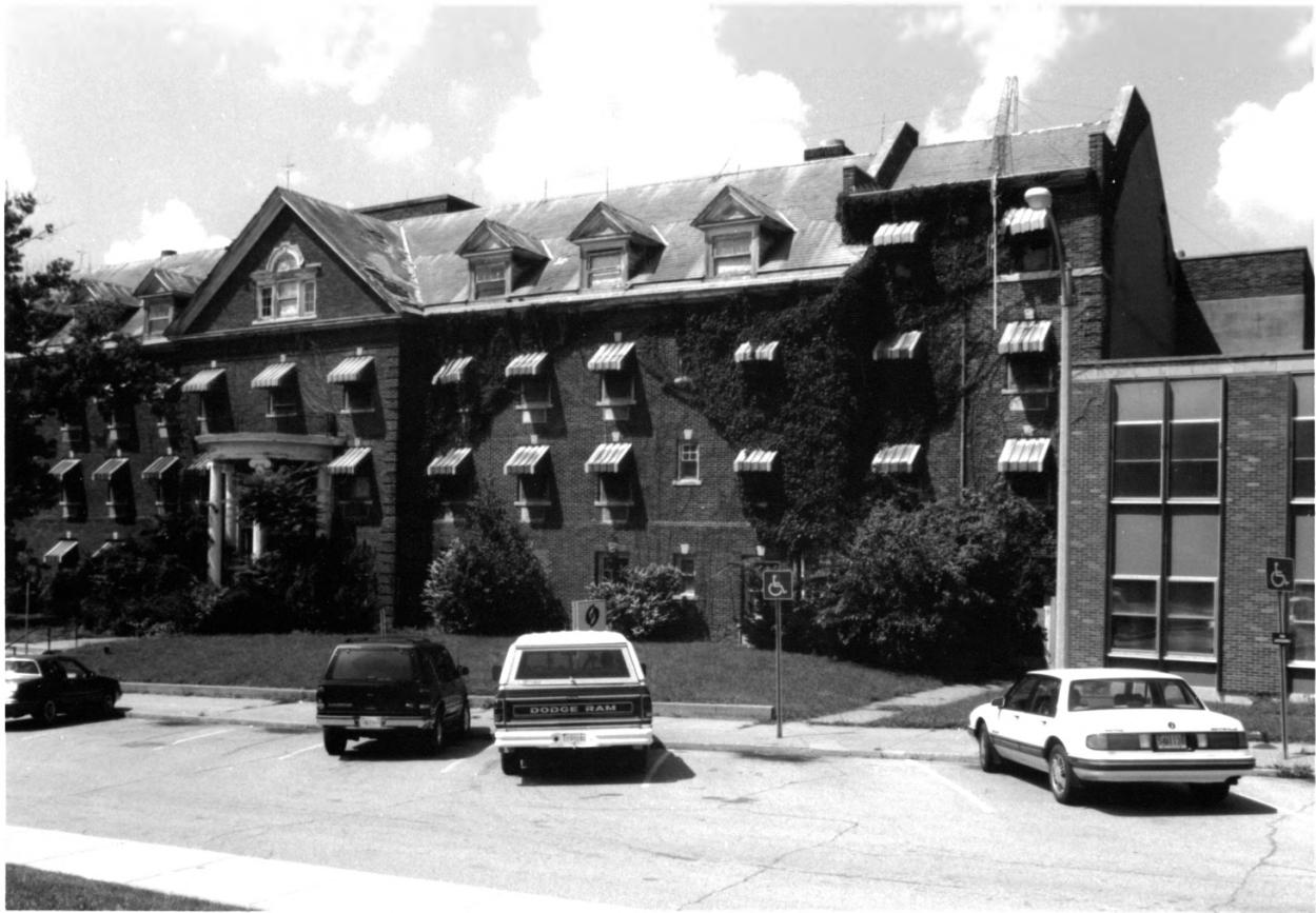
CULVER UNION HOSPITAL, CRAWFORDSVILLE, MONTGOMERY CO., IN, PHOTO No. 1
