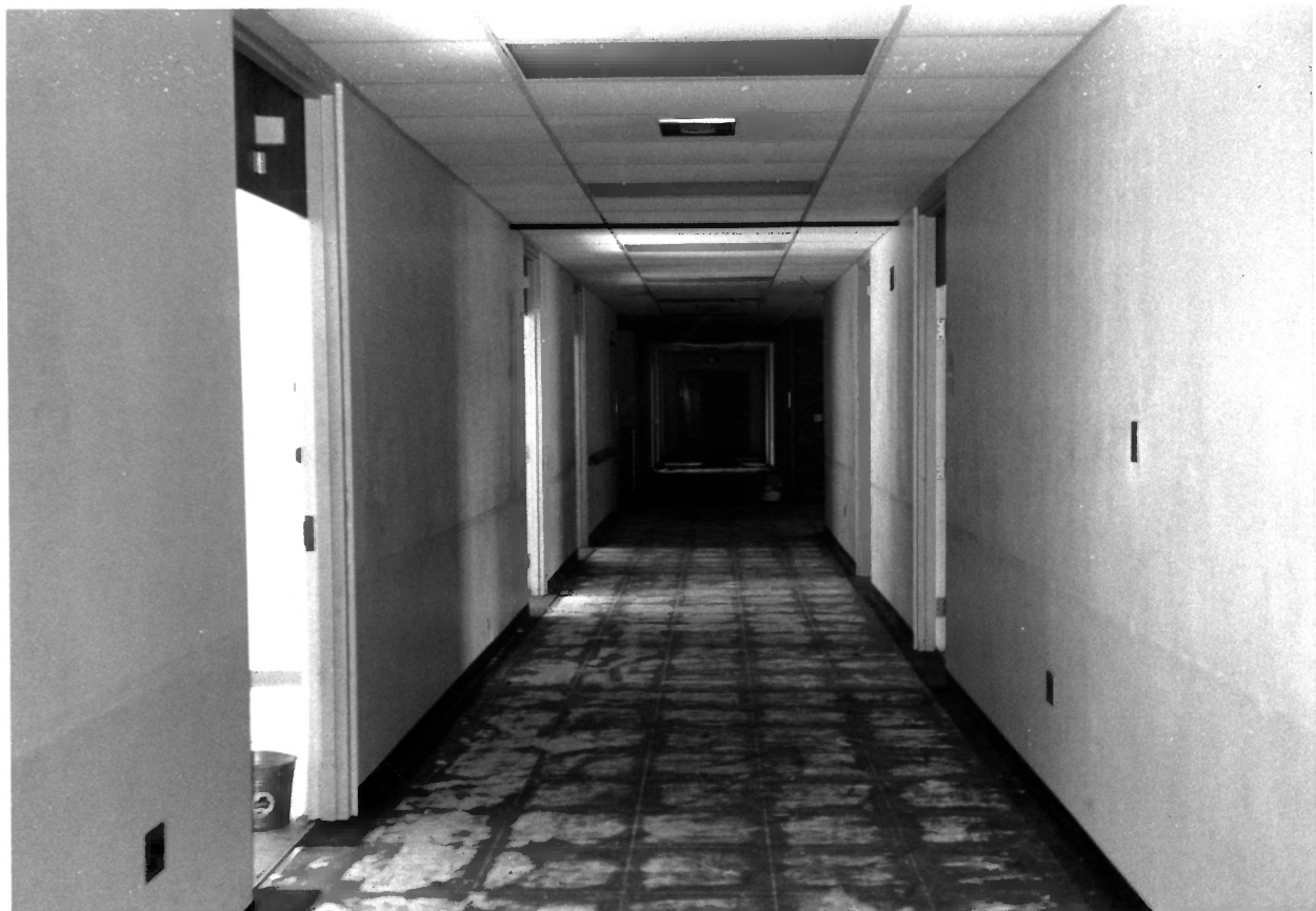
CULVER UNION HOSPITAL, CRAWFORDSVILLE, MONTGOMERY CO., IN - PHOTO No. 28
