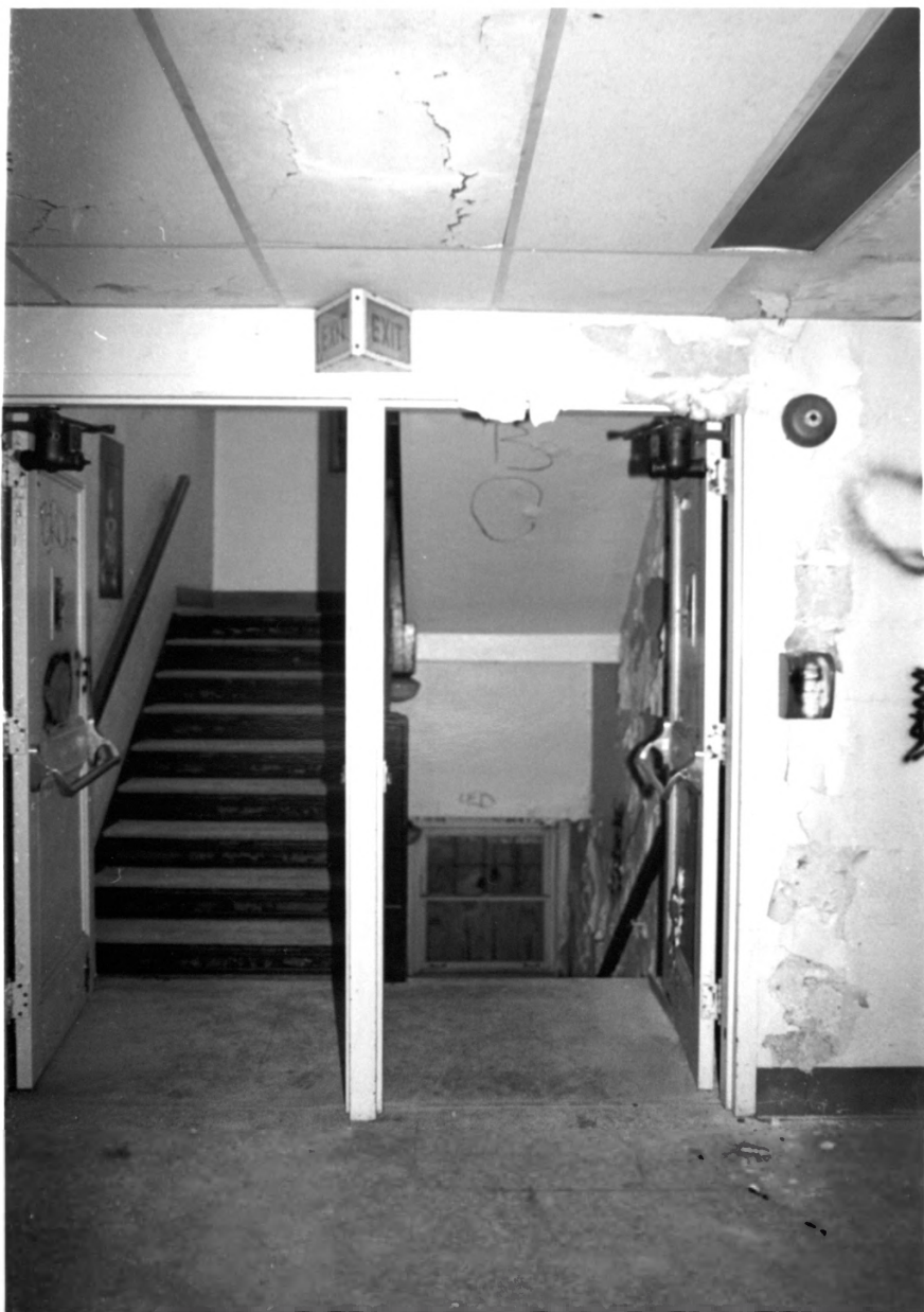
CULVER UNION HOSPITAL, CRAWFORDSVILLE, MONTGOMERY COUNTY, IN - PHOTO No. 25
