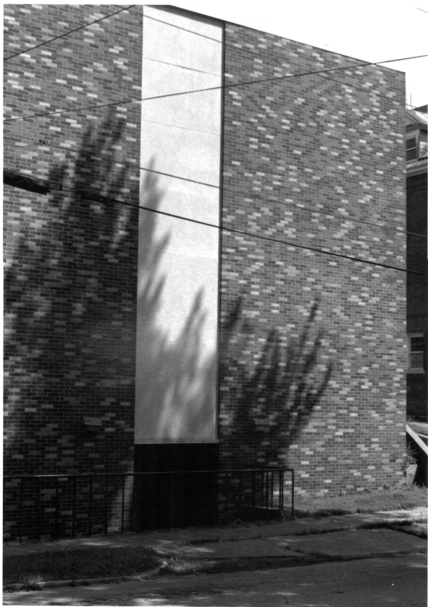
CULVER UNION HOSPITAL, CRAWFORDSVILLE, MONTGOMERY COUNTY, IN - PHOTO NO. 8
