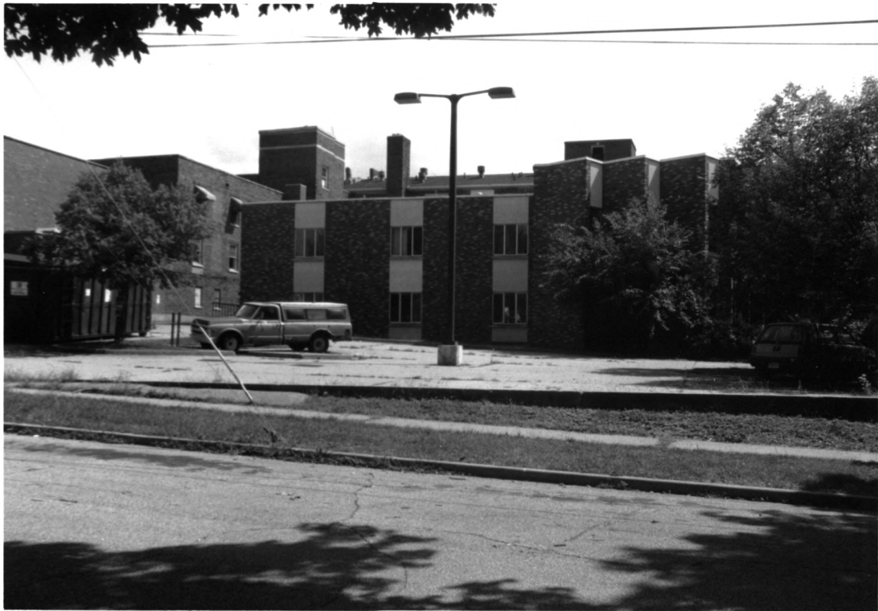
CULVER UNION HOSPITAL, CRAWFORDSVILLE, MONTGOMERY COUNTY, IN - PHOTO No. 10
