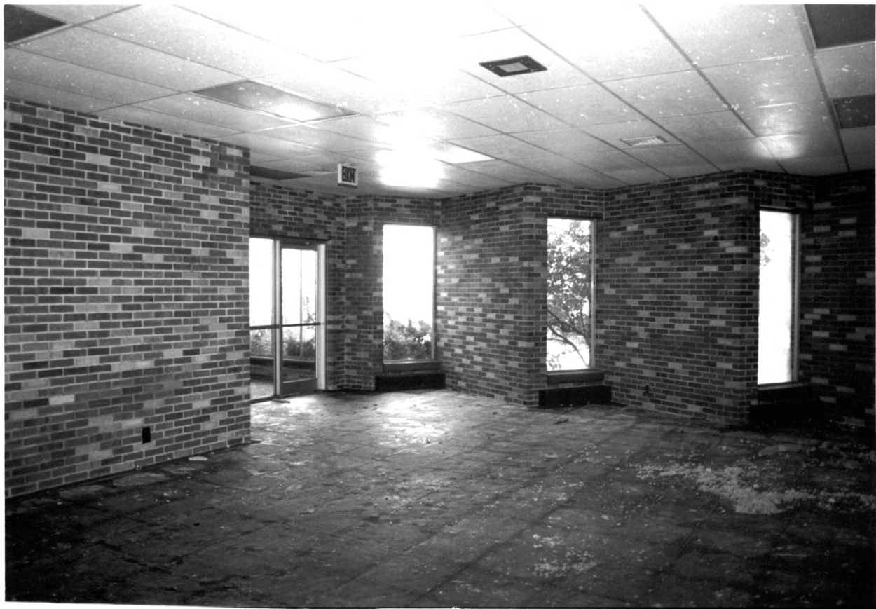
CULVER UNION HOSPITAL, CRAWFORDSVILLE, MONTGOMERY CO., IN - PHOTO No. 23
