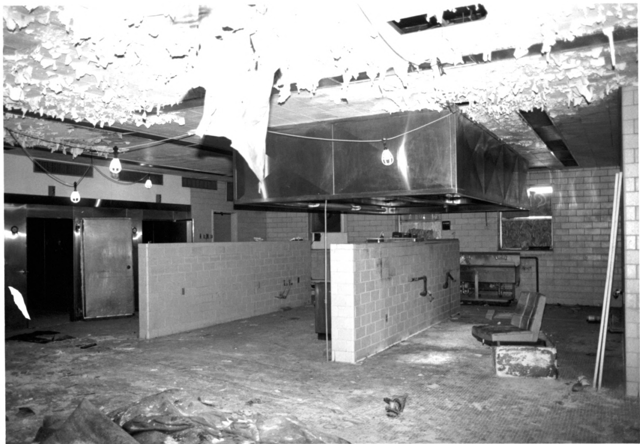
CULVER UNION HOSPITAL, CRAWFORDSVILLE, MONTGOMERY CO., IN - PHOTO No. 22
