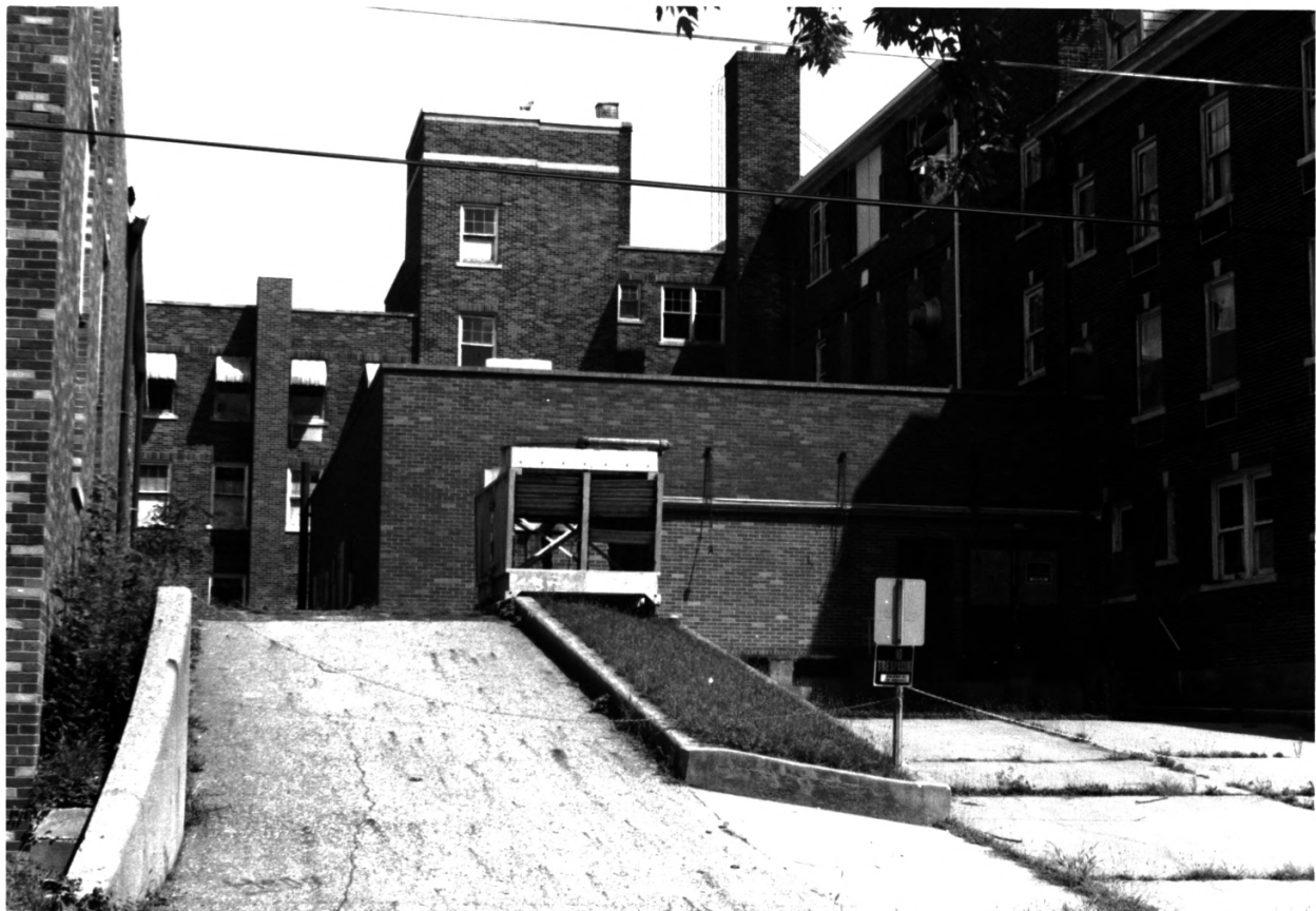
CULVER UNION HOSPITAL, CRAWFORDSVILLE, MONTGOMERY CO, IN - PHOTO No. 7
