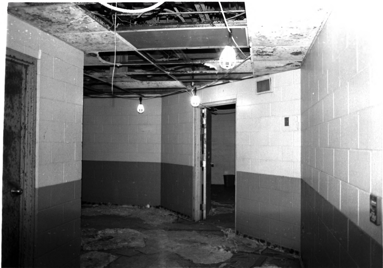
CULVER UNION HOSPITAL, CRAWFORDSVILLE, MONTGOMERY CO, IN - PHOTO NO. 17
