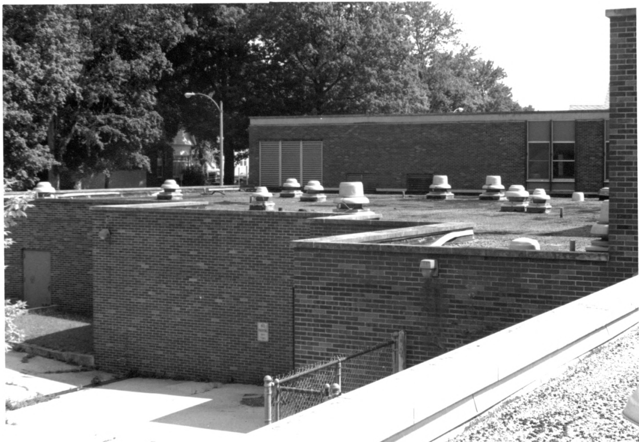
CULVER UNION HOSPITAL, CRAWFORDSVILLE, MONTGOMERY CO, IN - PHOTO NO. 24
