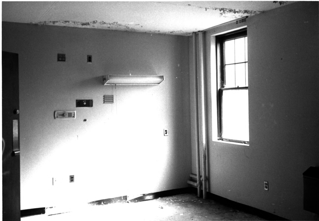
CULVER UNION HOSPITAL, CRAWFORDSVILLE, MONTGOMERY COUNTY, IN - PHOTO No. 27
