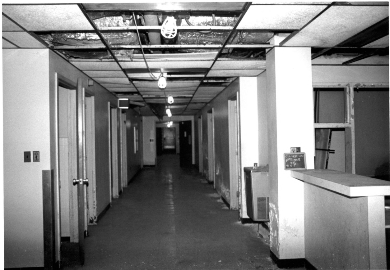
CULVER UNION HOSPITAL, CRAWFORDSVILLE, MONTGOMERY CO., IN - PHOTO No. 20
