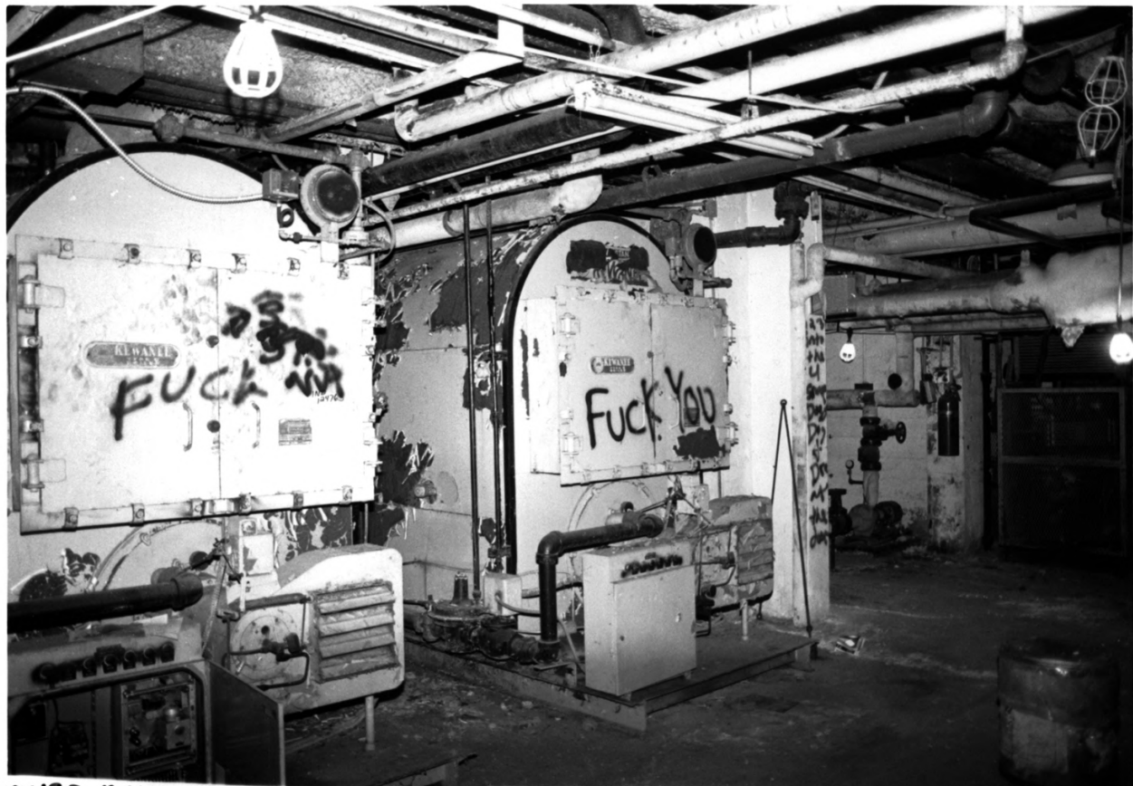
CULVER UNION HOSPITAL, CRAWFORDSVILLE, MONTGOMERY CO.; IN - PHOTO NO. 16
