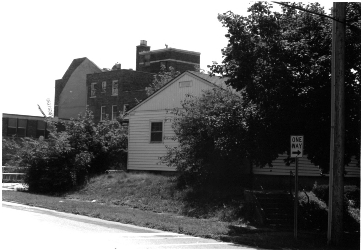
CULVER UNION HOSPITAL, CRAWFORDSVILLE, MONTGOMERY CO., IN - PHOTO NO. 12
