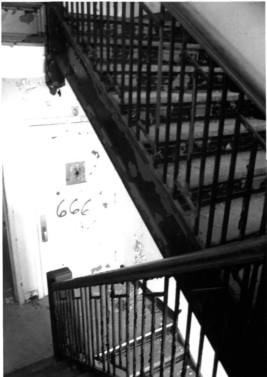
CULVER UNION HOSPITAL, CRAWFORDSVILLE, MONTGOMERY COUNTY, IN - PHOTO No. 32
