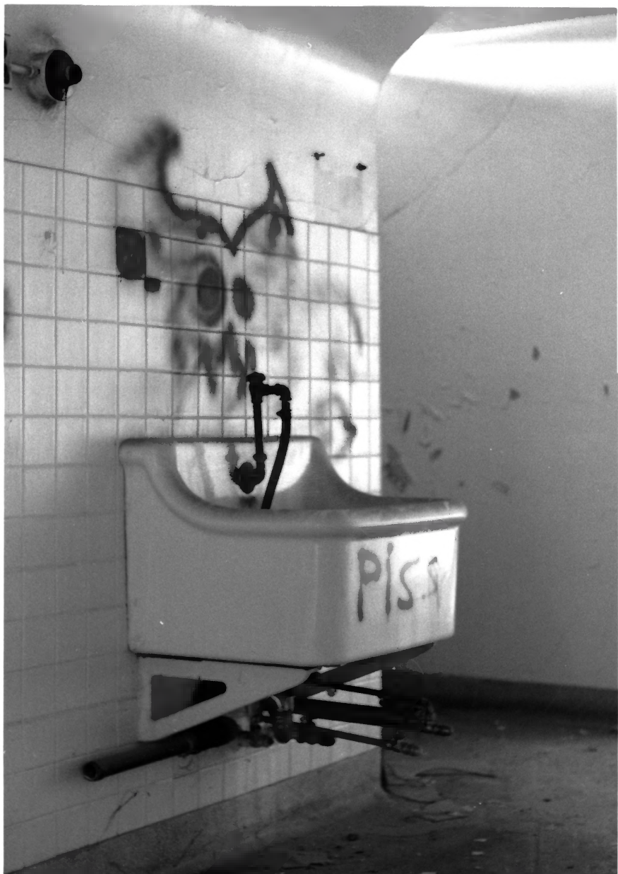
CULVER UNION HOSPITAL, CRAWFORDSVILLE, MONTGOMERY COUNTY, IN - PHOTO No. 35
