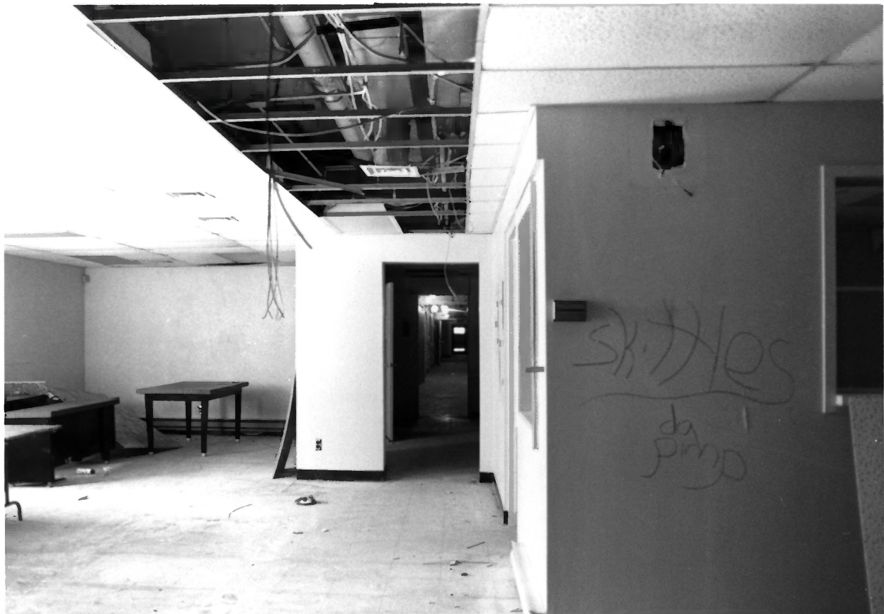
CULVER UNION HOSPITAL, CRAWFORDSVILLE, MONTGOMERY CO., IN - PHOTO No. 18
