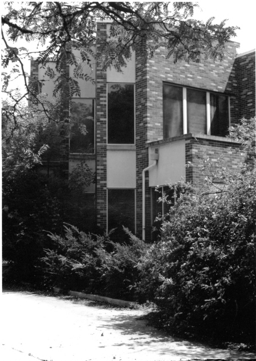
CULVER UNION HOSPITAL, CRAWFORDSVILLE, MONTGOMERY COUNTY, IN - PHOTO NO. 9
