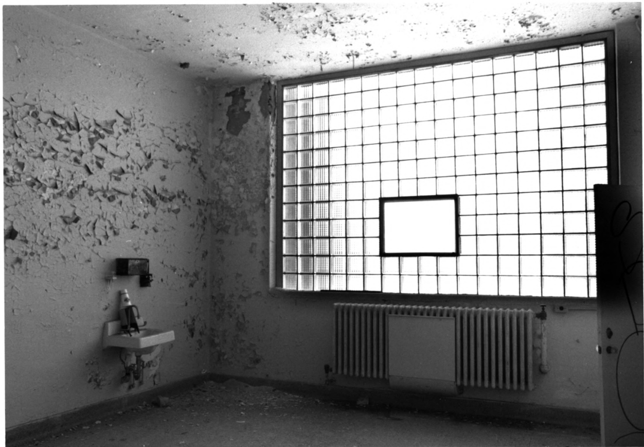
CULVER UNION HOSPITAL, CRAWFORDSVILLE, MONTGOMERY CO., IN - PHOTO No. 37
