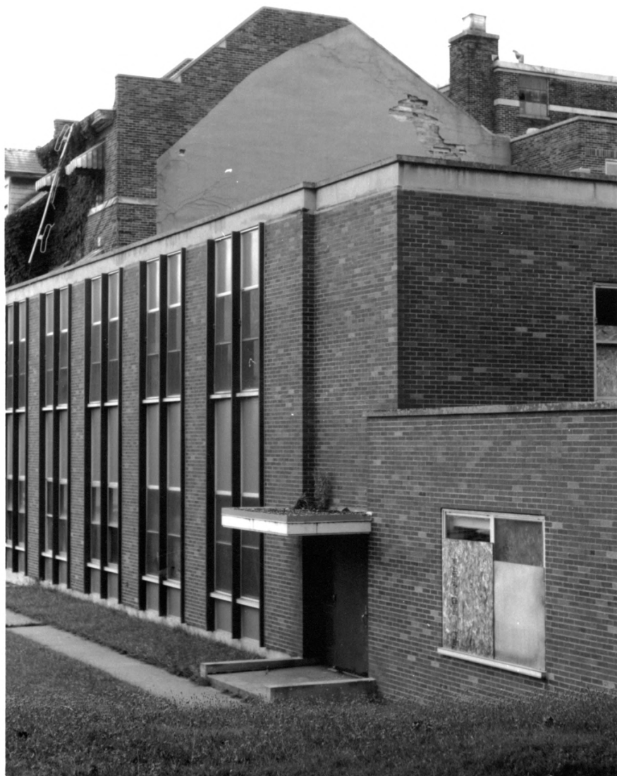
CULVER UNION HOSPITAL, CRAWFORDSVILLE, MONTGOMERY COUNTY, IN - PHOTO No. 14
