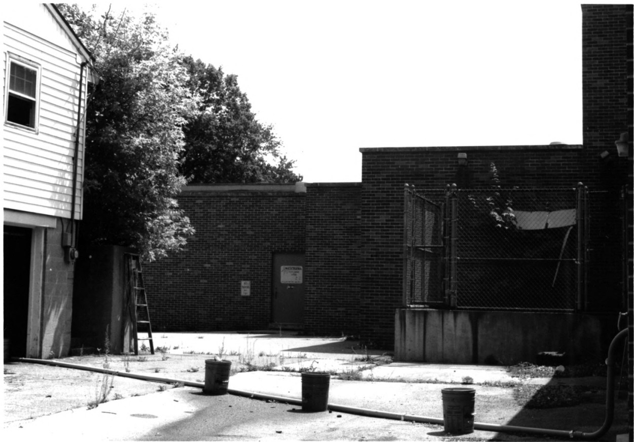
CULVER UNION HOSPITAL, CRAWFORDSVILLE, MONTGOMERY CO., IN - PHOTO No. 11
