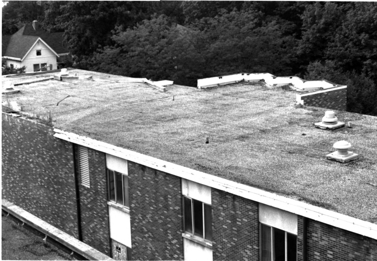
CULVER UNION HOSPITAL, CRAWFORDSVILLE, MONTGOMERY CO.; IN - PHOTO No. 30
