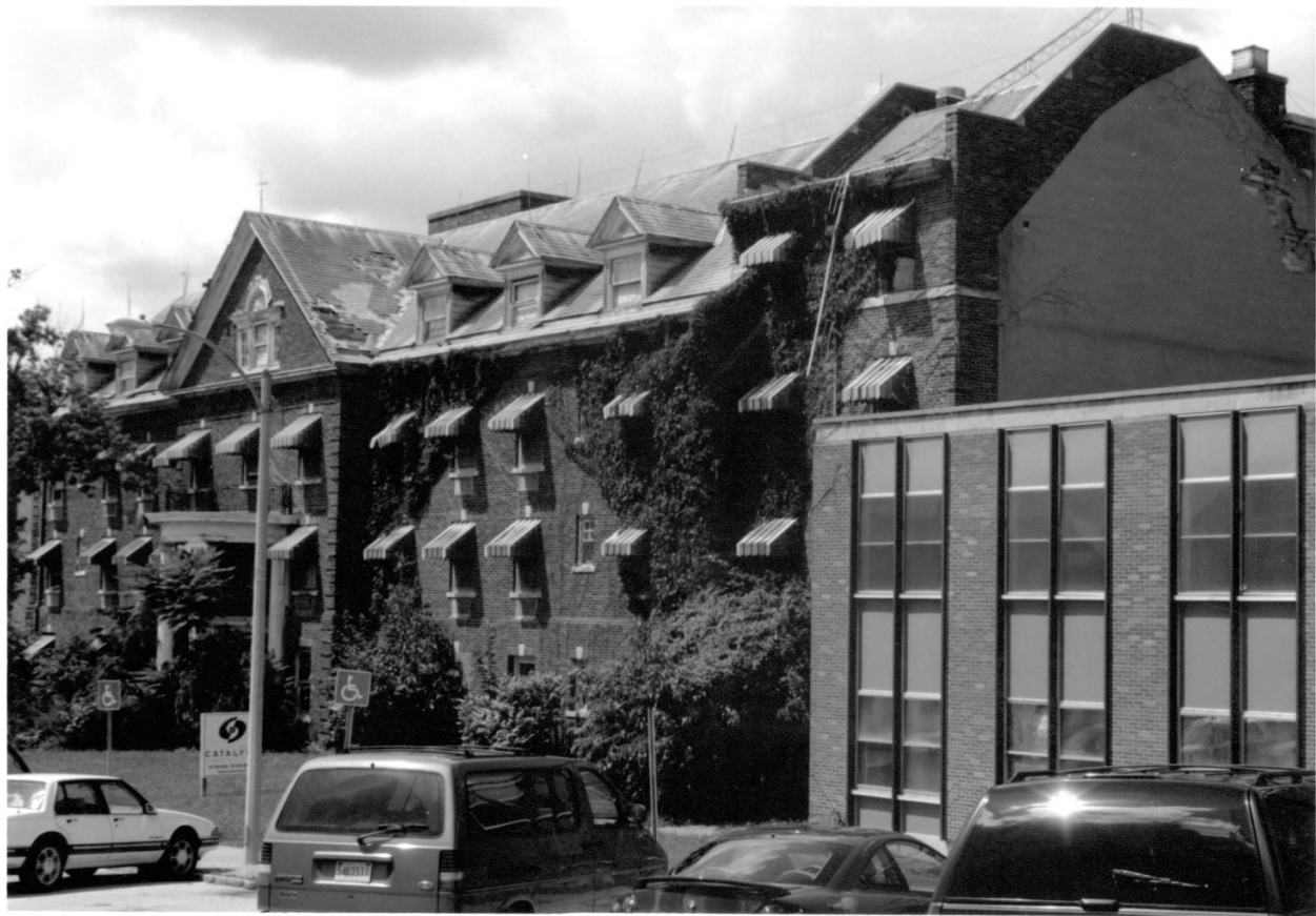
LOWER UNION HOSPITAL, CRAWFORDSVILLE, MONTGOMERY CO., IN, PHOTO No. 2
