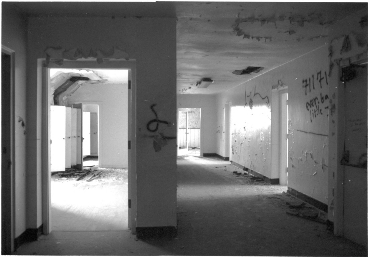
CULVER UNION HOSPITAL, CRAWFORDSVILLE, MONTGOMERY CO., IN - PHOTO No. 33
