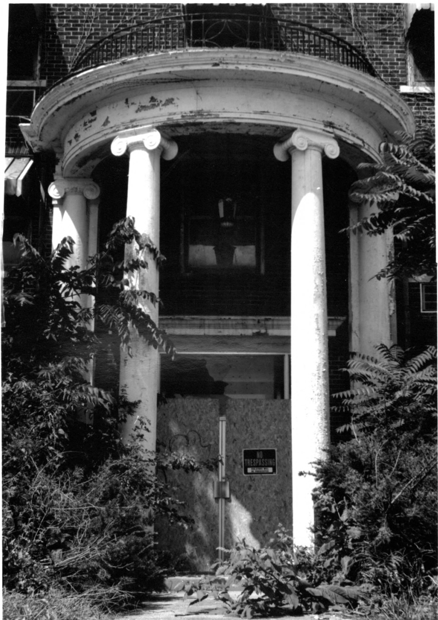
CULVER UNION HOSPITAL, CRAWFORDSVILLE, MONTGOMERY COUNTY, IN - PHOTO No. 4
