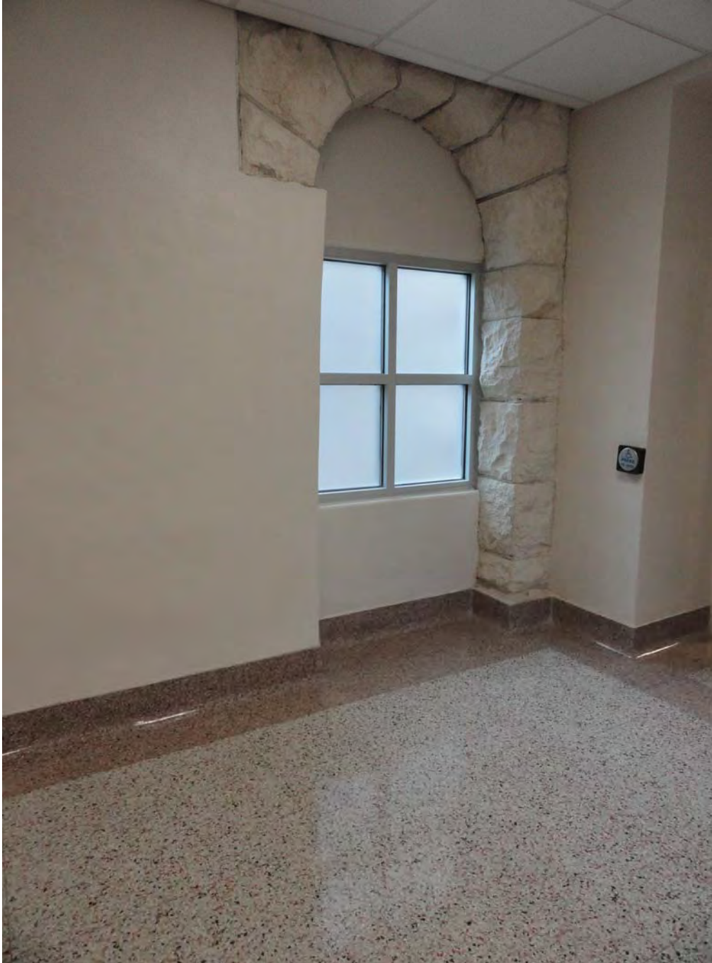
Photo 18: basement, original stone arch Photographed by Maria Pfeiffer, May 2015
