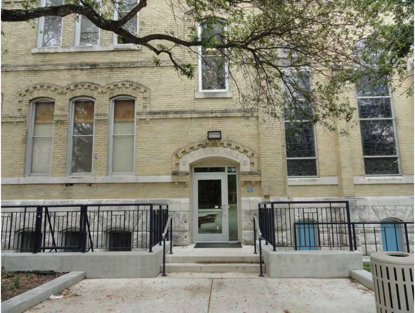
Photo 12: north elevation looking south Photographed by Maria Pfeiffer, May 2015
