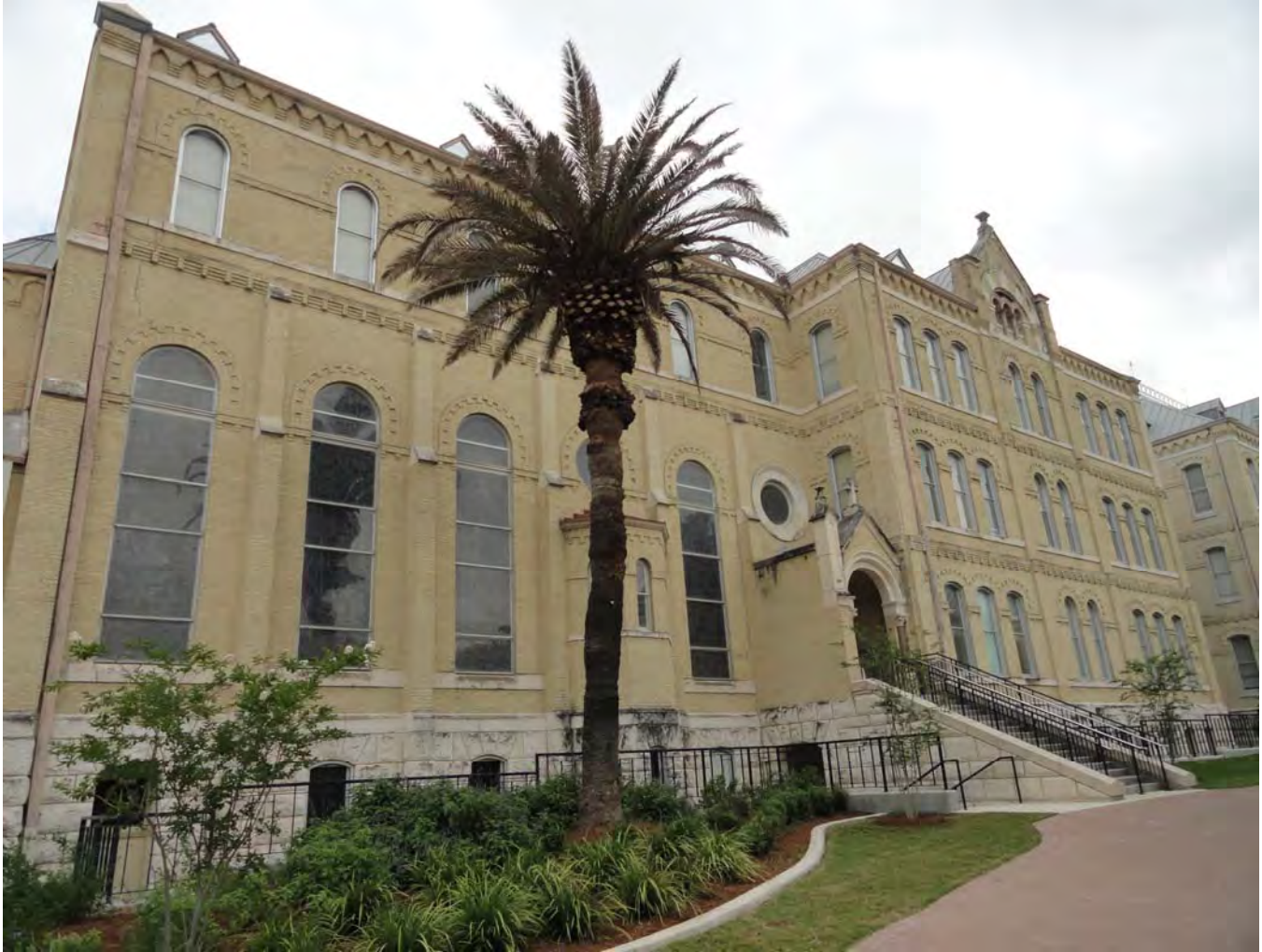
Photo 2: South elevation looking northeast Photographed by Maria Pfeiffer, May 2015
