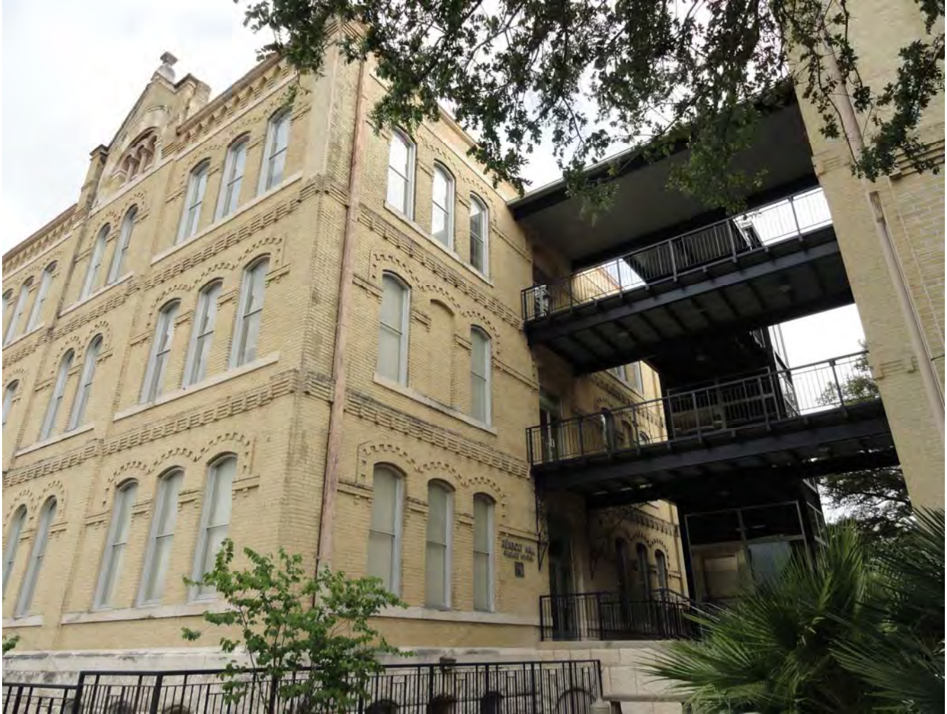
Photo 5: east elevation looking northwest Photographed by Maria Pfeiffer, May 2015
