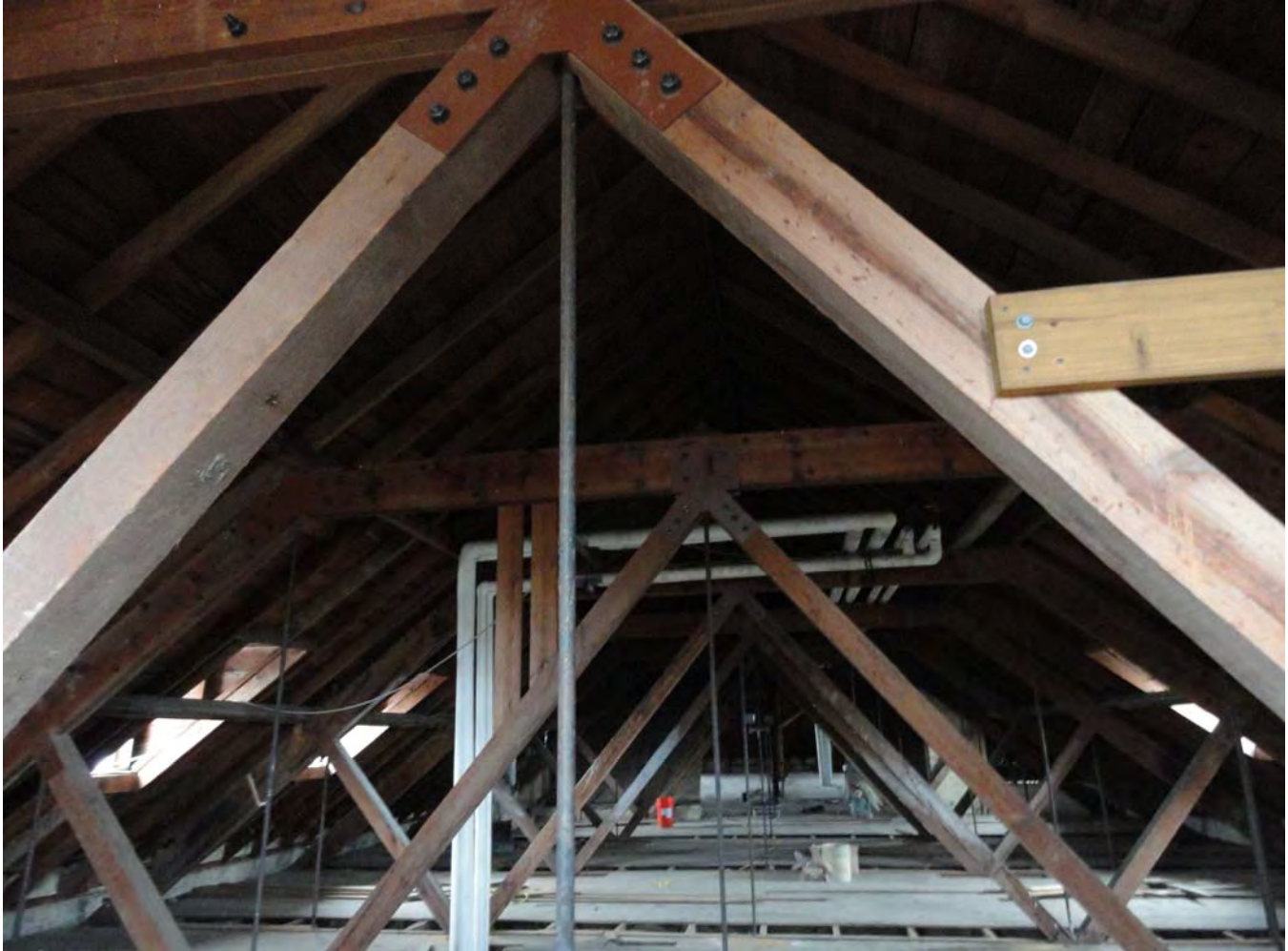
Photo 22: attic wooden trusswork Photographed by Maria Pfeiffer, May 2015
