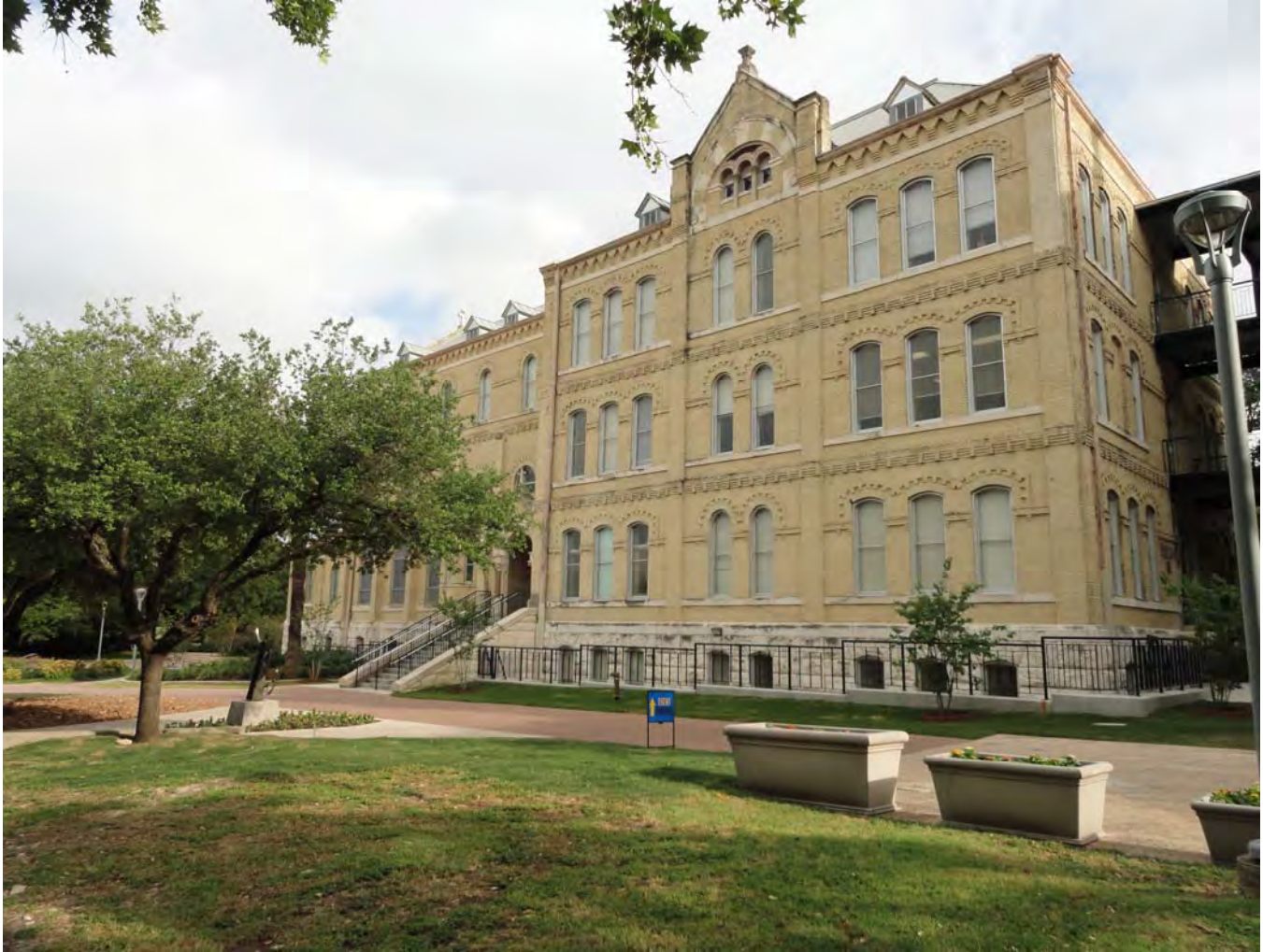
Photo 3: South elevation looking northeast Photographed by Maria Pfeiffer, May 2015
