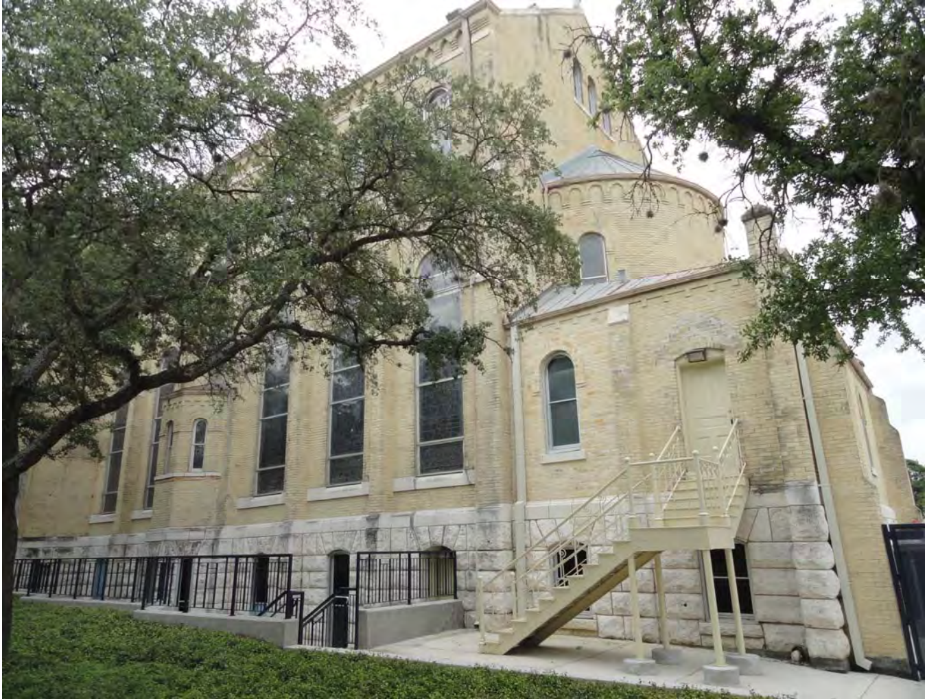
Photo 11: north elevation looking southeast Photographed by Maria Pfeiffer, May 2015
