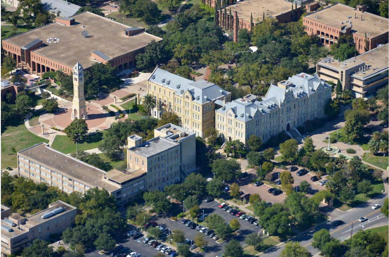
Photo 1: Reinbolt Hall, aerial view looking northwest Photographed by Maria Pfeiffer, October 2013
