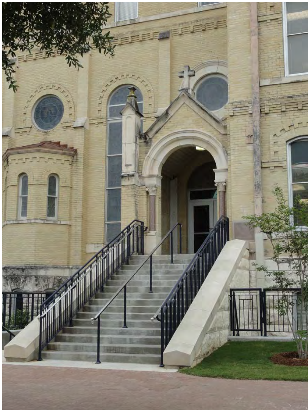
Photo 6: south entryway looking north Photographed by Maria Pfeiffer, May 2015
