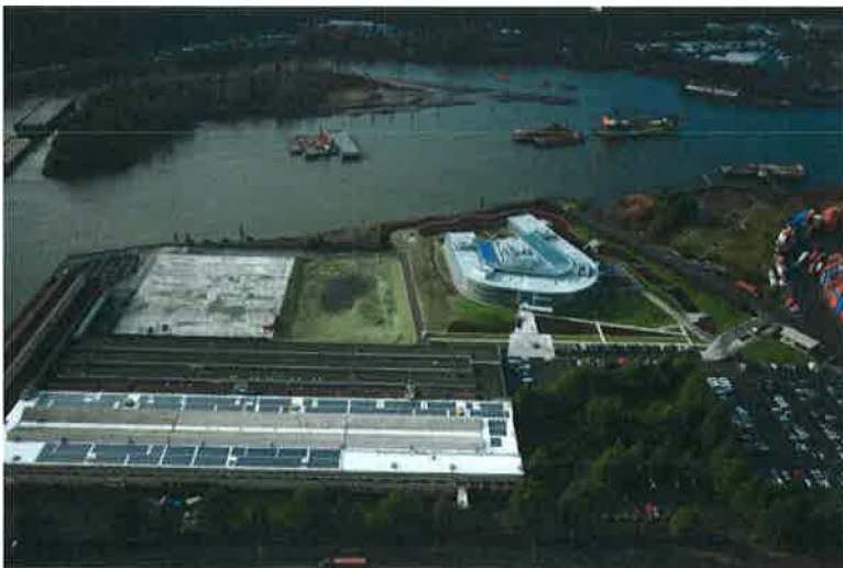
View to west photographed by Kemer Nelson for GSA, January 2013
