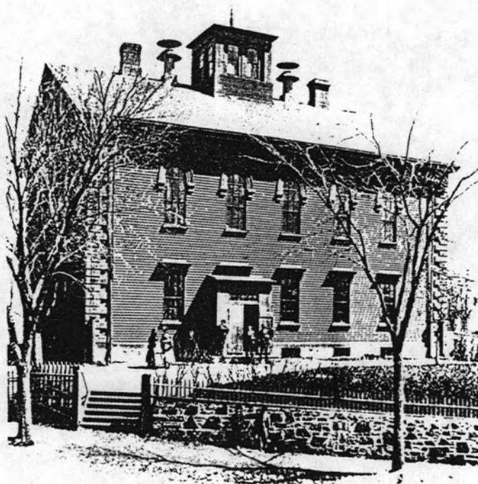
In 1852 the first high school was built in Lynn and used until 1892 when severe overcrowding necessitated the building of Lynn Classical and English High School. The original high school structure served for many years as a shoemaking school.
