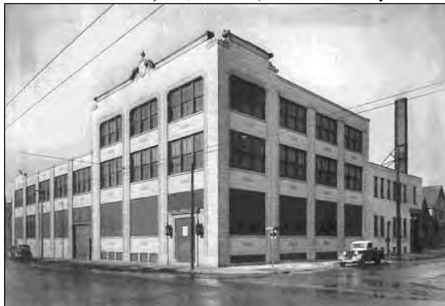
Figure 4: View of the south and east façades, ca. 1937 (Milwaukee County Historical Society)
