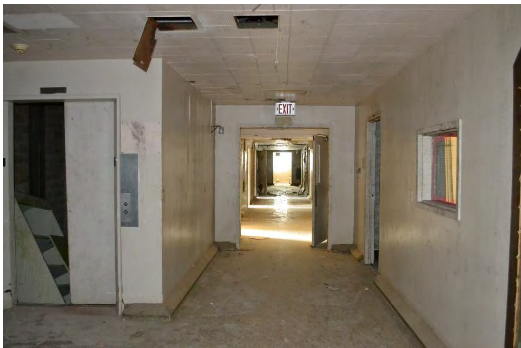
Photo 13 – Interior, first floor hallway, view west. Original terrazzo flooring, terrazzo curbs, door openings are visible.
